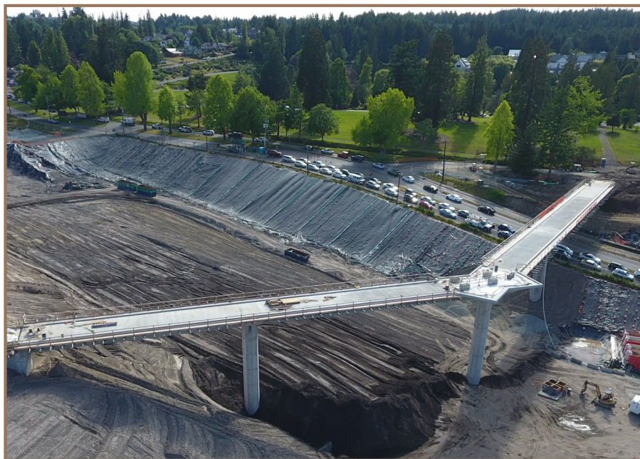
Point Defiance Trails Project during construction. Photo courtesy of Atkinson Construction.
