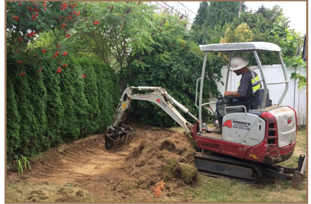
A contractor excavates contaminated soil from a yard in Tacoma.
