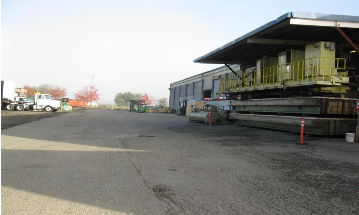
Photo 3: Slag Excavated Area and Contaminated Soil Excavated Area – from the South
