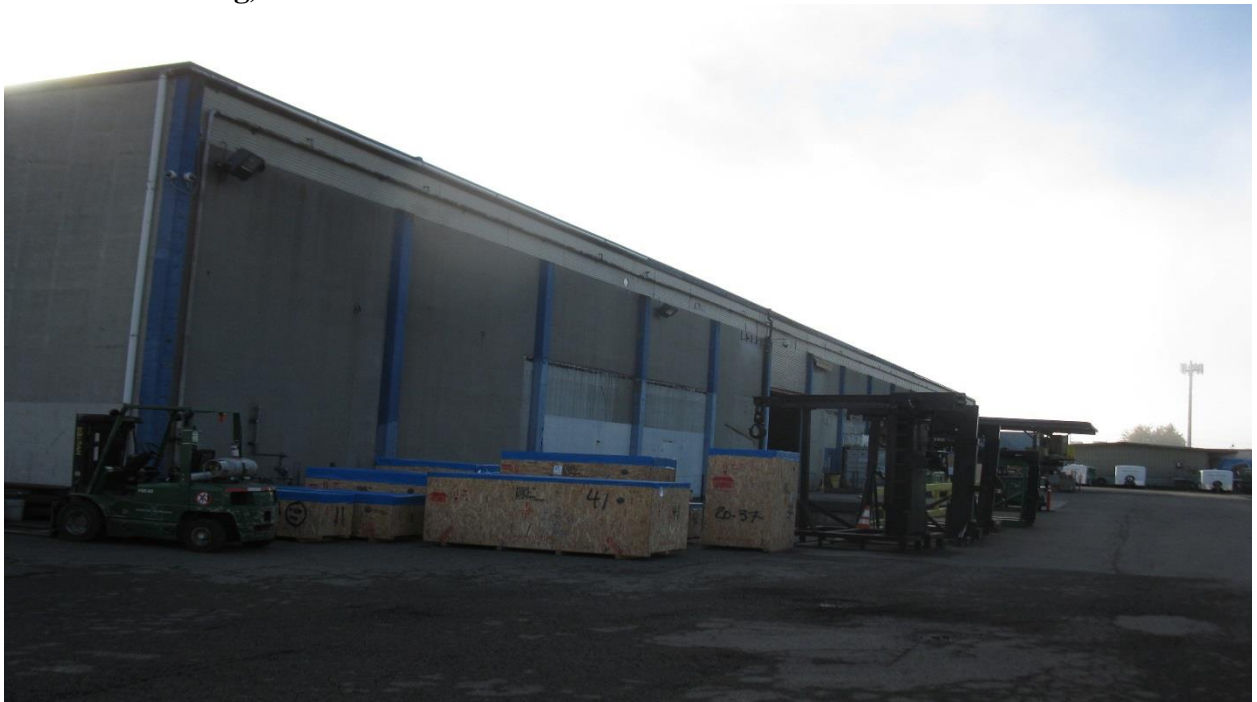
Photo 2: Slag Excavated Area and Contaminated Soil Excavated Area (middle of the Building) Area—from the Northwest
