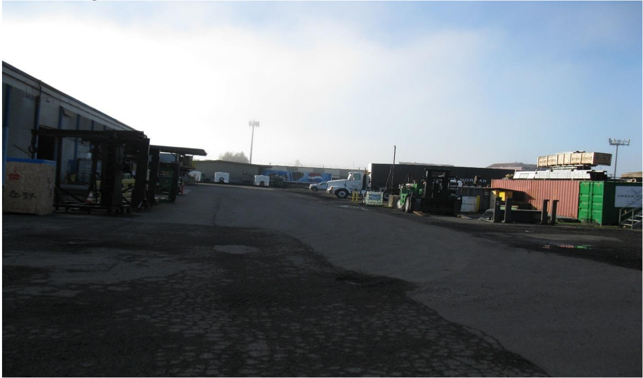
Photo 1: Slag Excavated Area – from the north
