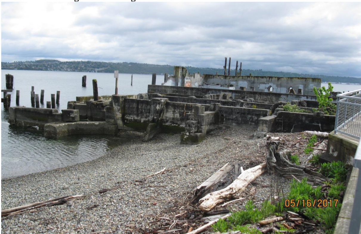
Photo 6: Remaining Mill Building/Foundation and Intertidal Area – from the West
