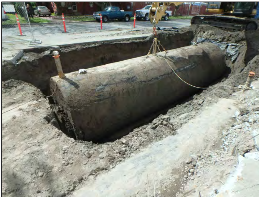
Photograph 14: View of UST2 as it was being removed from the excavation.
