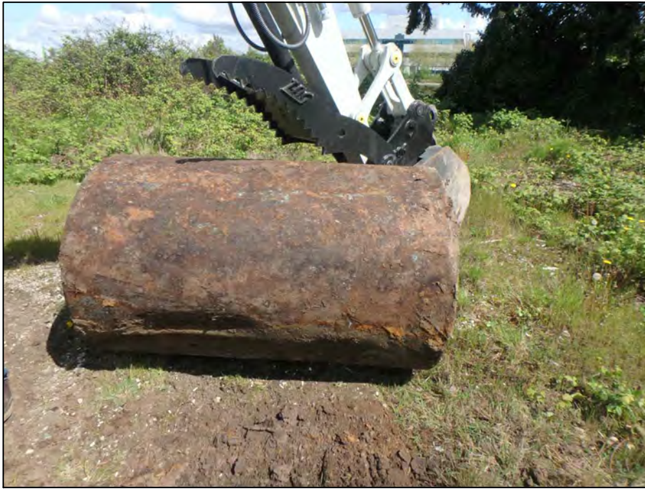
Photograph 19: View of UST5 after being removed from the excavation.
