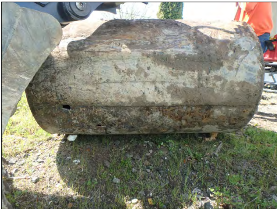
Photograph 20: View of pin holes and visible corrosion on the bottom of UST5 after its removal from the excavation.
