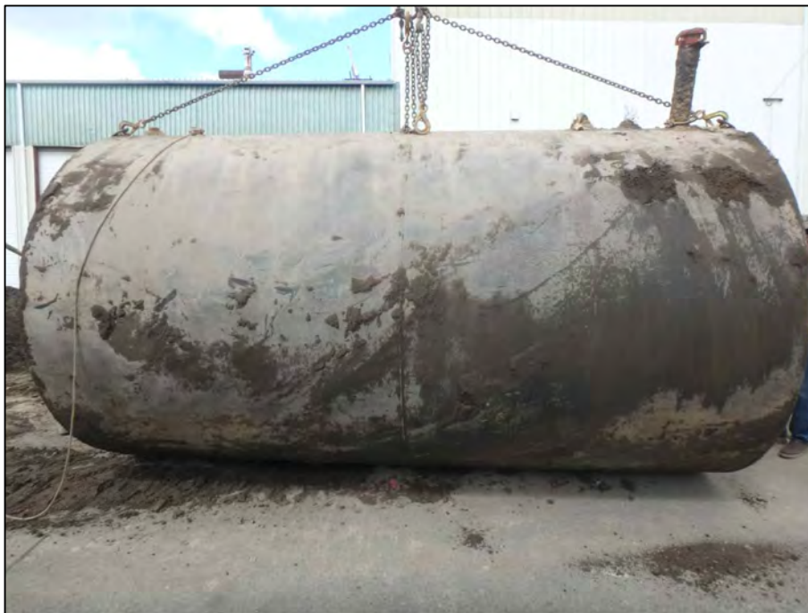
Photograph 16: View of UST3 after being removed from the excavation. No obvious signs of punctures or other evidence of a release from UST3 was observed.
