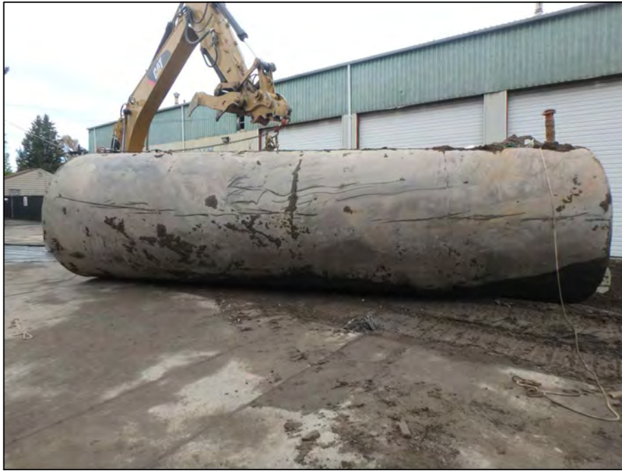
Photograph 17: Side view of UST4 after being removed from the excavation.
