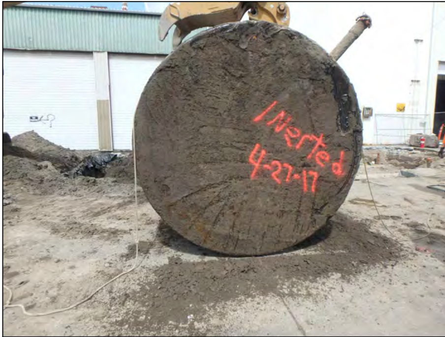
Photograph 13: Side view of UST1 after being removed from the excavation.
