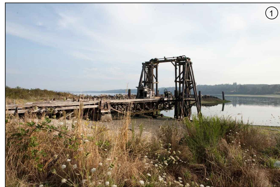
PHOTO 1: LOG TRANSFER DOCK
