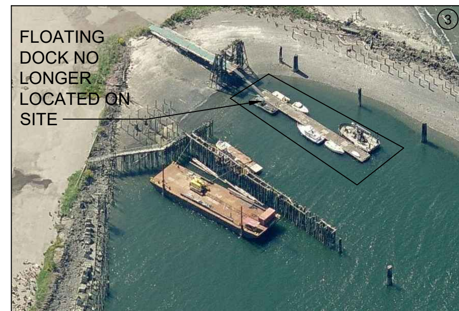
PHOTO 3: CONVEYOR/PIER (FROM BING MAPS IMAGERY)
