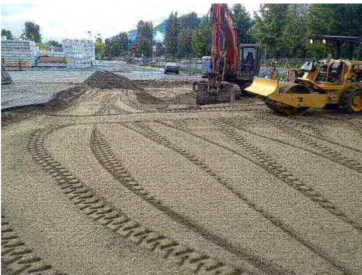
Photo #12. Backfilled excavation.
