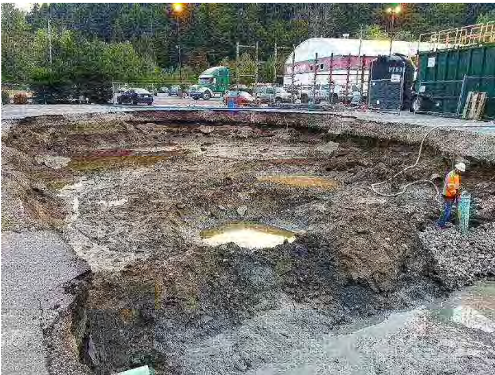
Photo #11. The final extent of excavation.
