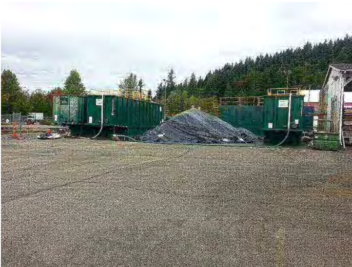
Photo #8. Dewatering effluent was stored in a series of four Baker tanks.
