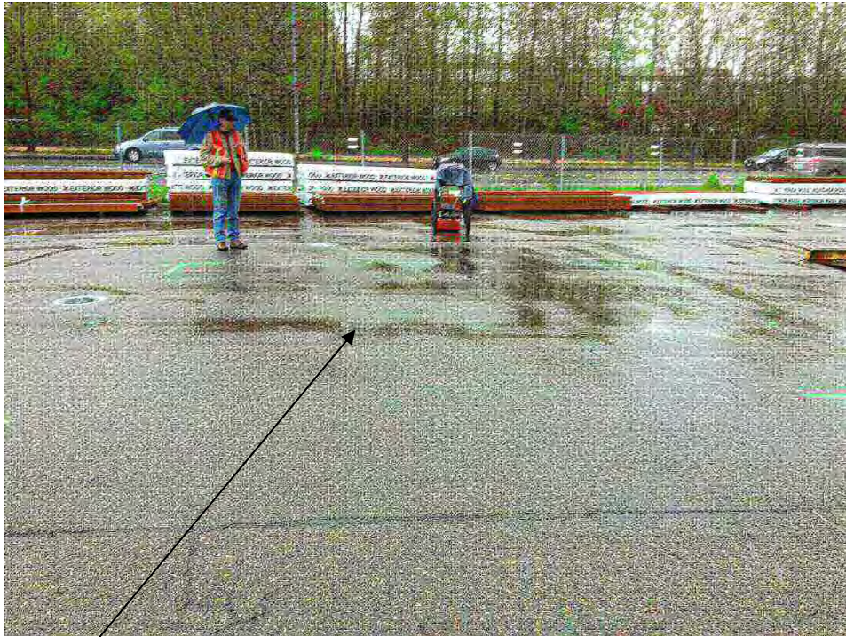
Possible UST pit
