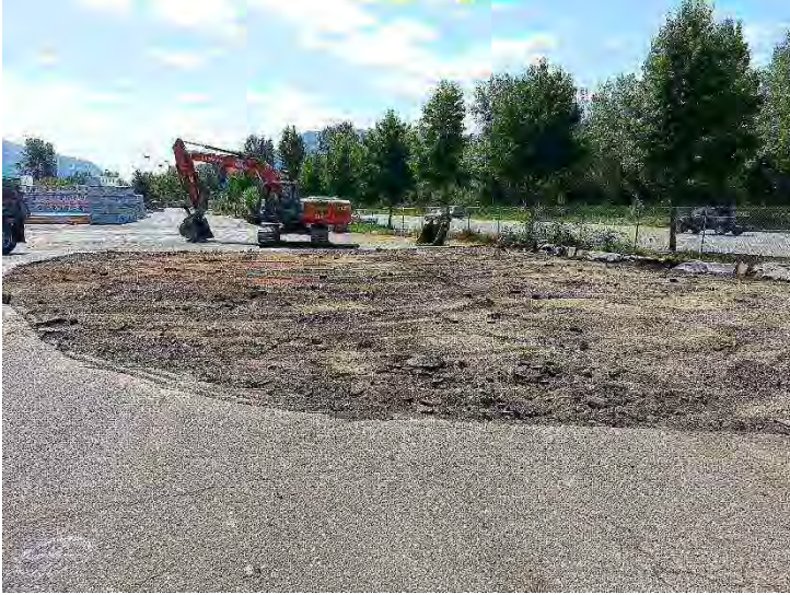
Photo #1. Asphalt removed and preparing to excavate contaminated soil.
