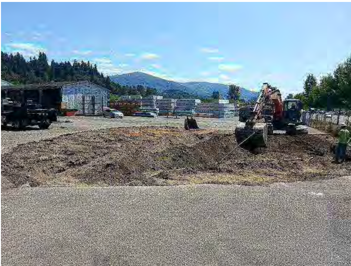
Photo #2. Removal of clean overburden fill soils.
