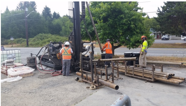
Photograph 3. Sonic drill rig advancing monitoring well MW-17.
