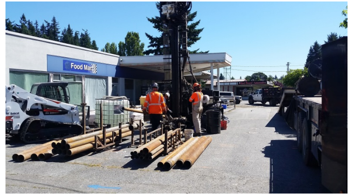
Photograph 2. Sonic drill rig advancing boring B08.
