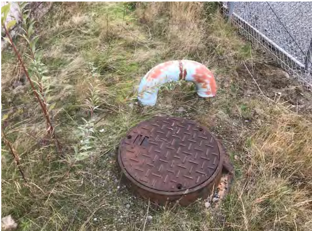
Photo 6: Leachate collection sump (manhole)
