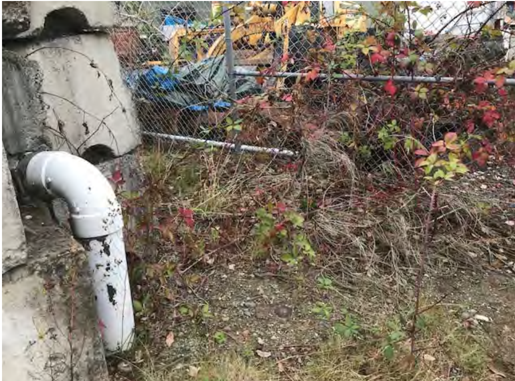
Photo 7: View to the northeast of the cell drain boot showing some aging on the paint coating
