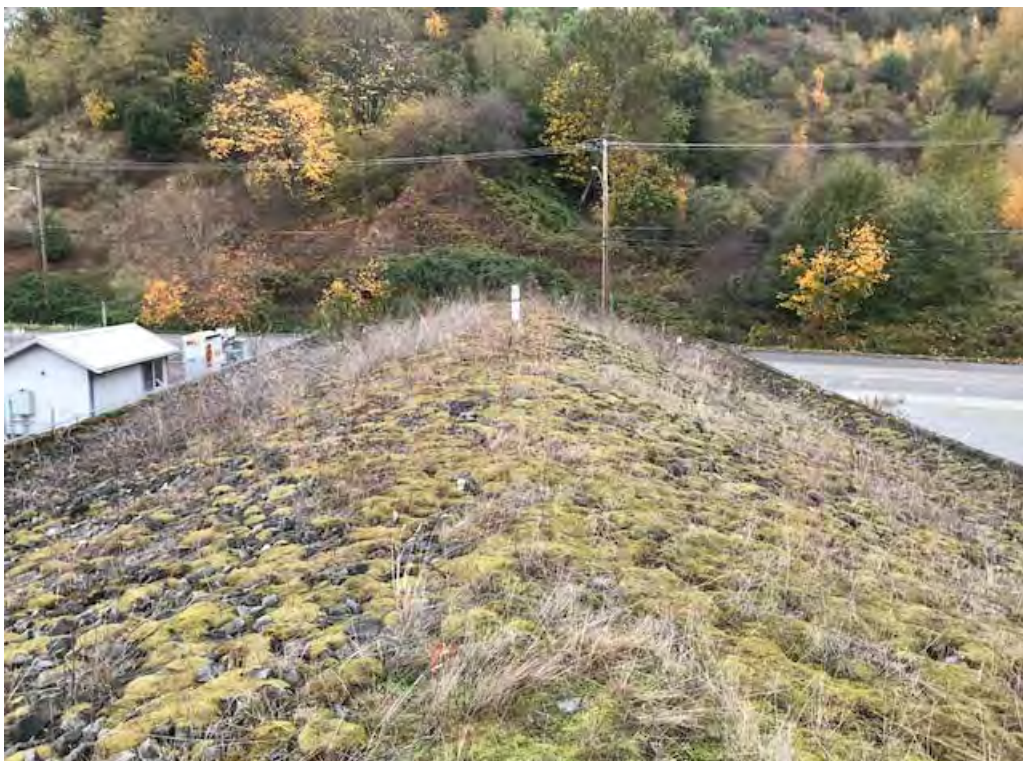
Photo 4: Top of containment cell, view to the north, northern gas boot visible
