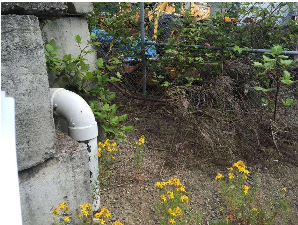
Photo 6: View to the northeast of the cell drain boot showing some aging on the paint coating. Scotch broom and blackberry bush growth visible.
