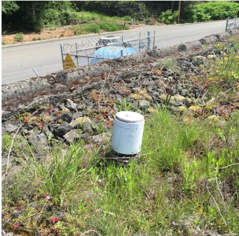
Photo 1: Cleanout boot; looking to the northeast (Marine View Drive in background).
