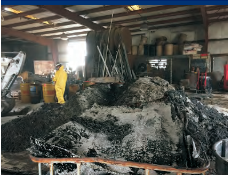
Photo 42 Sludge solidification activities in Warehouse A.
