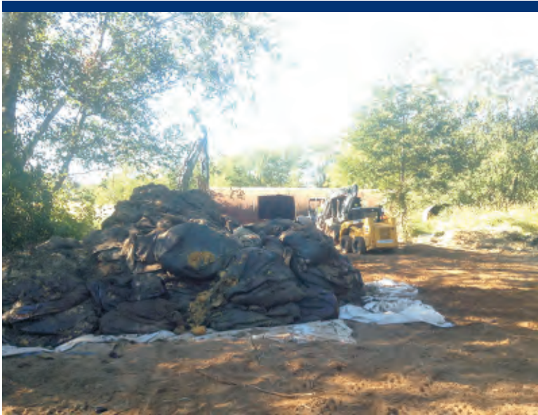
Photo 49 Stock pile of contents of Tank 50.
