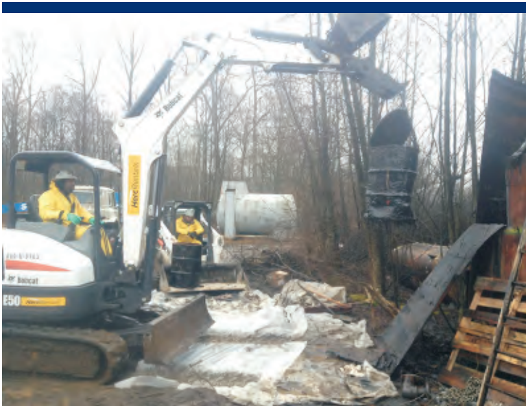
Photo 36 ERRS removing drums from Tank T-18.
