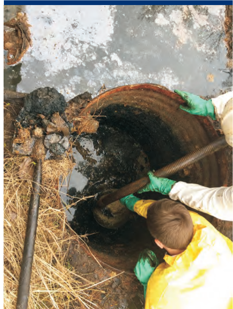
Photo 41 ERRS removing water from sump on north side of Warehouse B.
