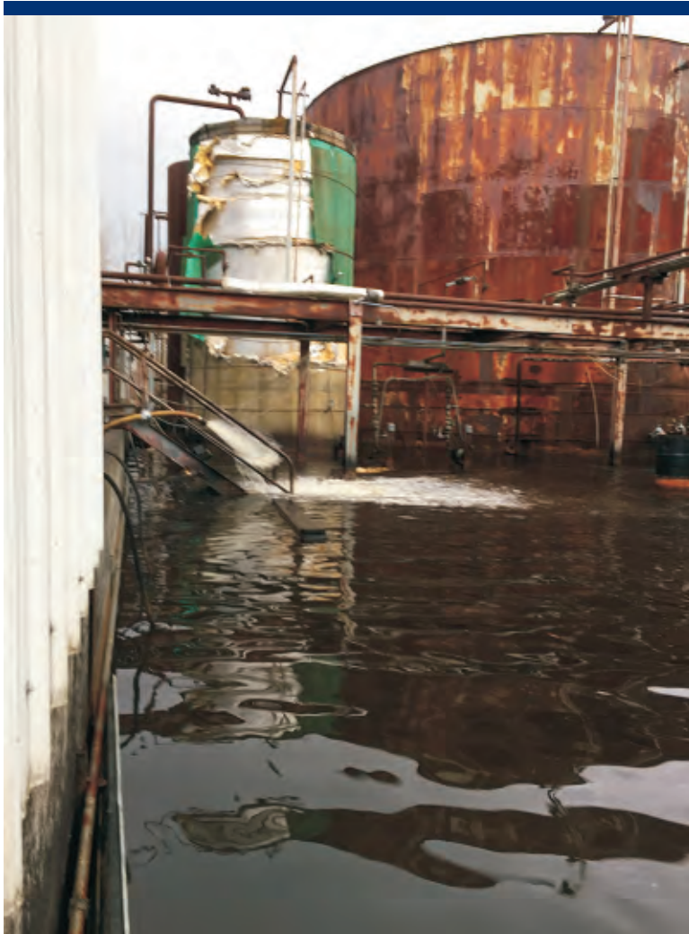
Photo 31 Pumping of water from Secondary Containment B into Secondary Containment C.
