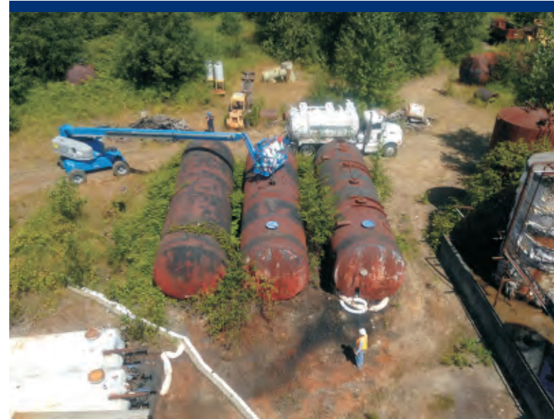
Photo 47 ERRS pumping tall oil from Tank 2.
