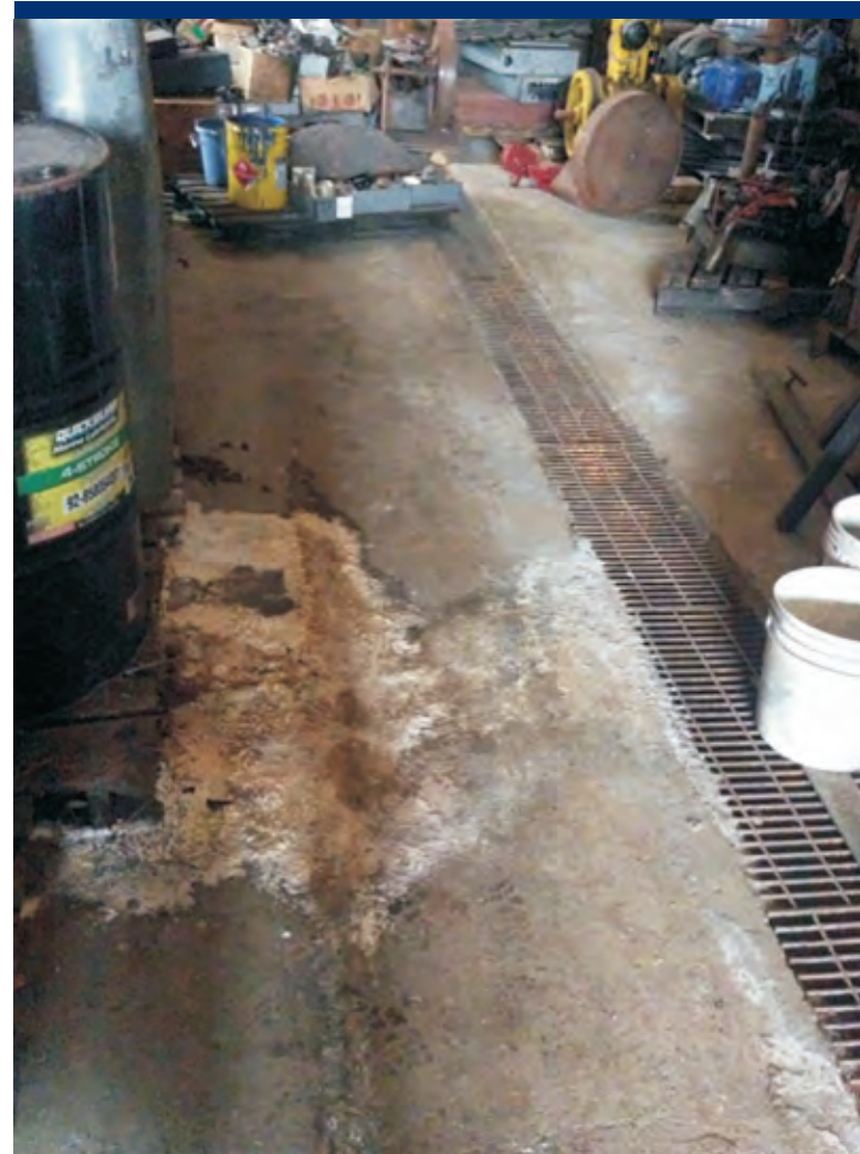
Photo 2 Trench running west to east in Warehouse A.
