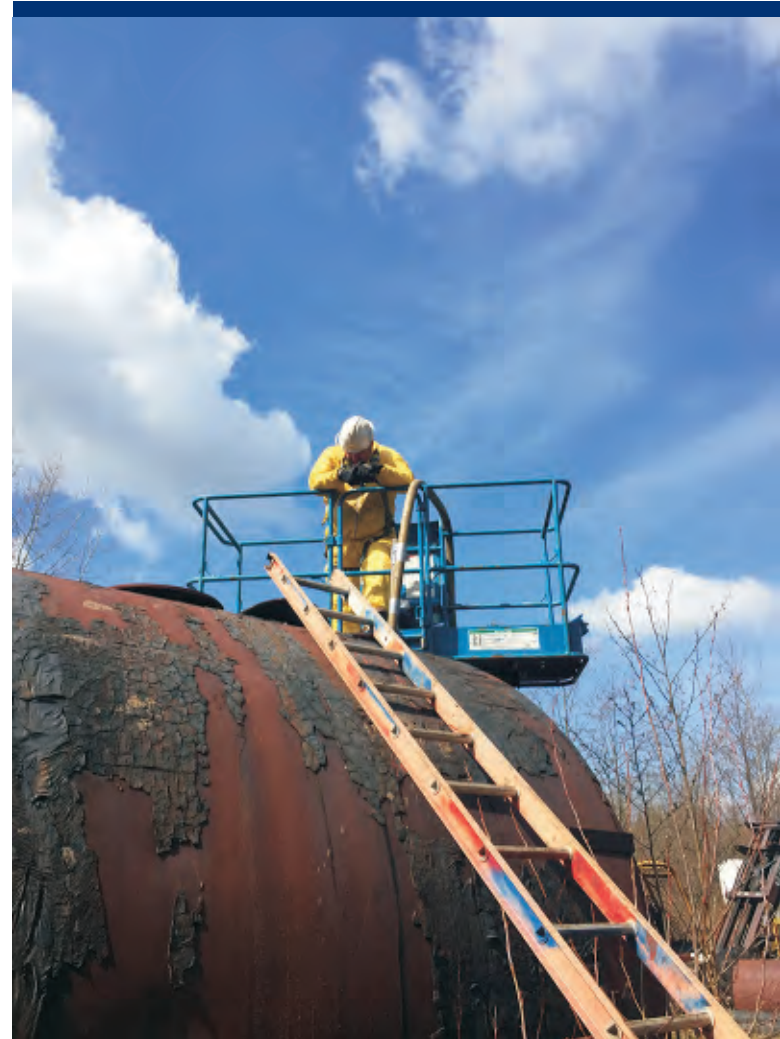
Photo 39 ERRS monitors oil removed from AST.
