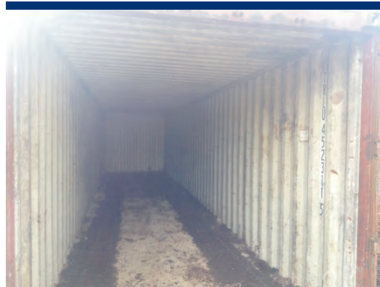
Photo 16 Final condition of Conex Box.
