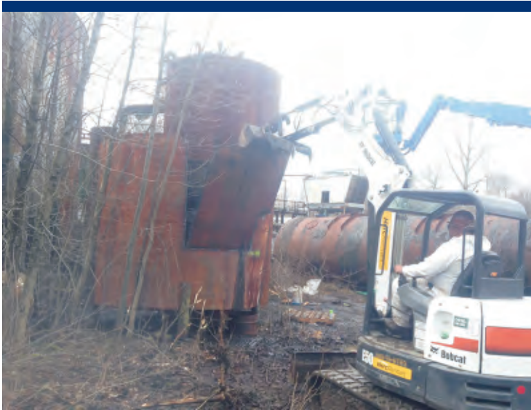
Photo 34 ERRS removing a section of sidewall from Tank T-18.
