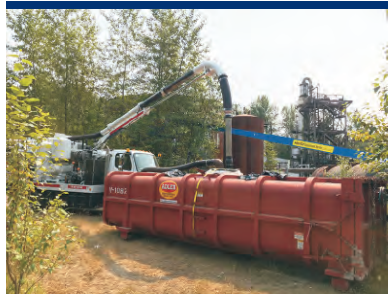
Photo 55 Sludge box setup with super sucker attached.
