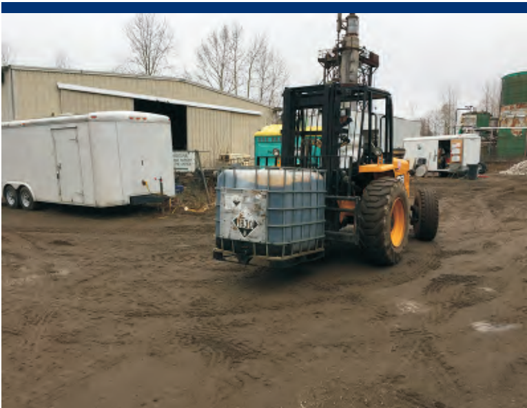
Photo 26 Tote being loaded for off-site transportation.
