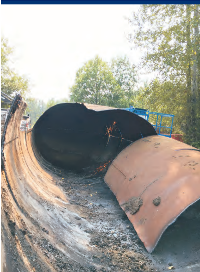
Photo 56 Cutting of Tank 50.
