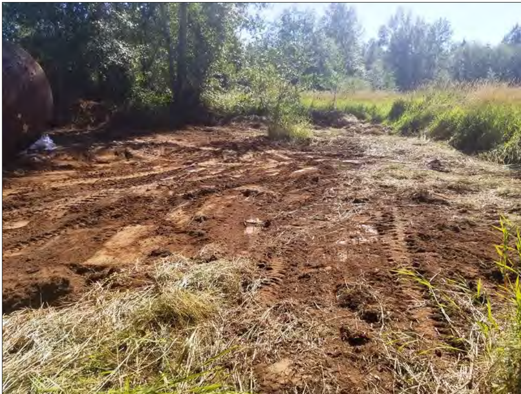
Figure 3. View looking west of APE at completion of excavations.
