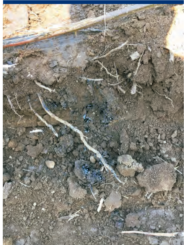
Photo 52 Weeps of oil from excavated soil walls.
