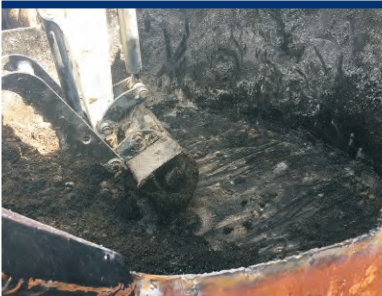
Photo 40 Final solidification of contents in Tank T-18.
