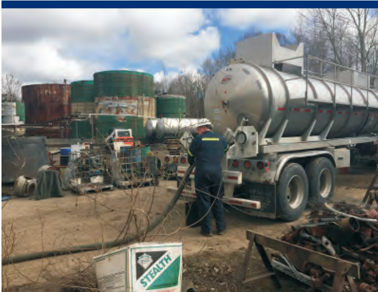
Photo 38 Oil is pumped into Vacuum Truck for disposal.
