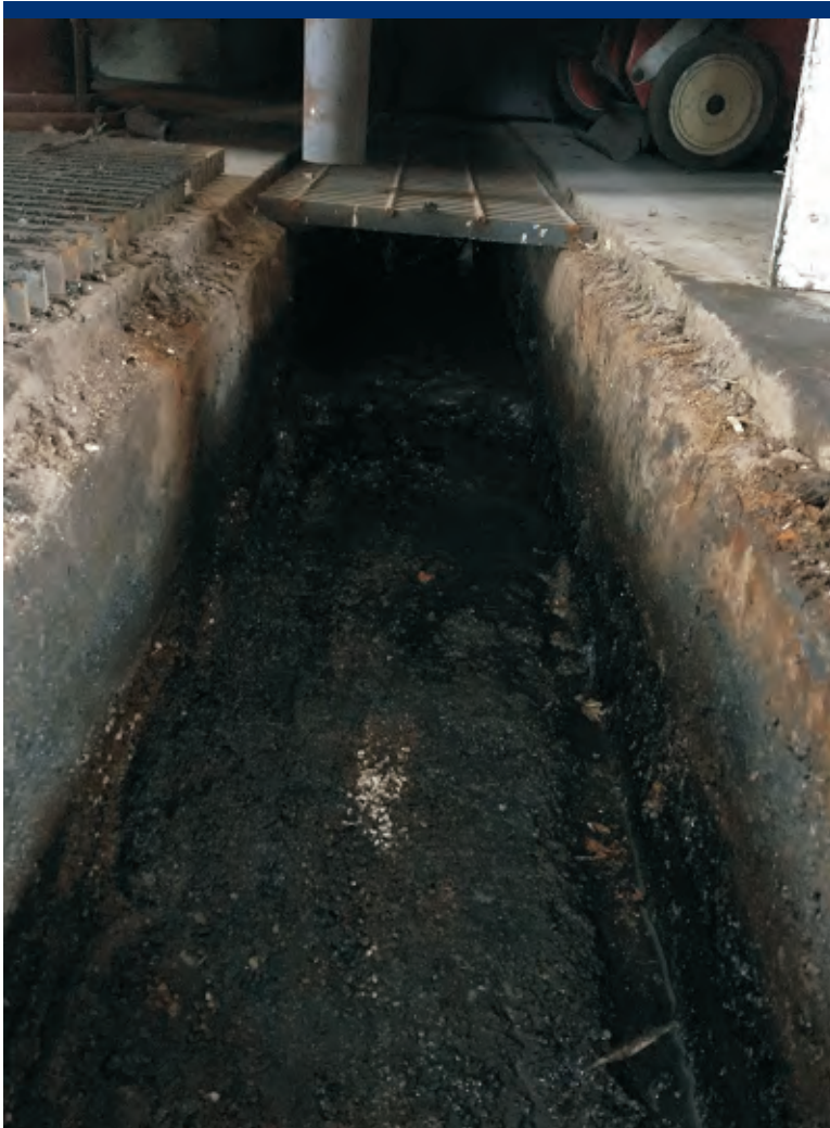
Photo 19 Empty trench in Warehouse A.
