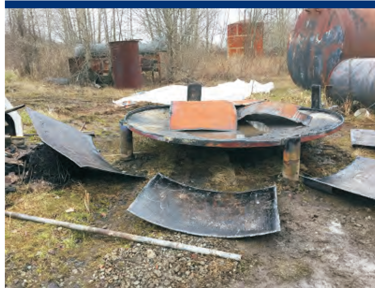
Photo 43 Final demolition of Tank T-18.
