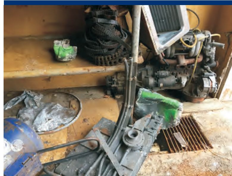
Photo 12 Pipe insulation in Warehouse B.
