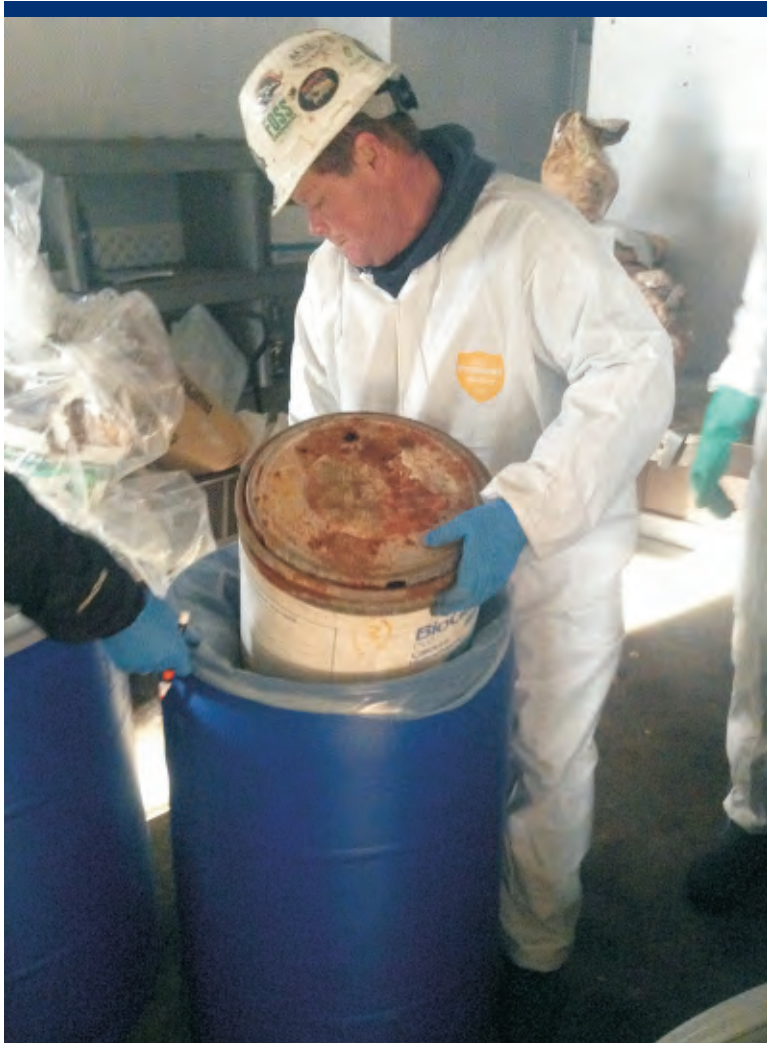
Photo 14 ERRS puts hazardous chemicals into lab packs for disposal.
