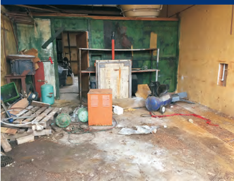
Photo 17 Warehouse B segregation room after removal of ACM.
