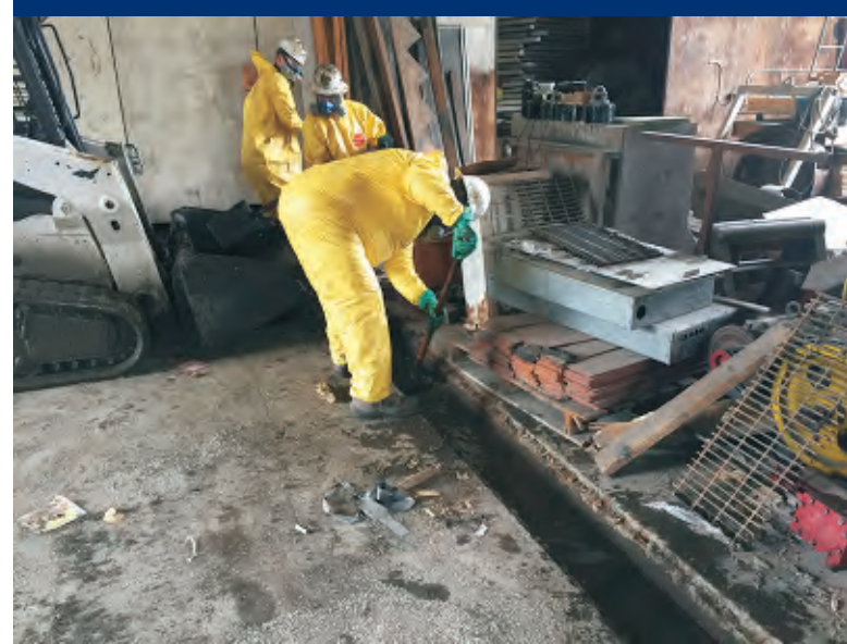
Photo 18 Removal of sediments from trench.
