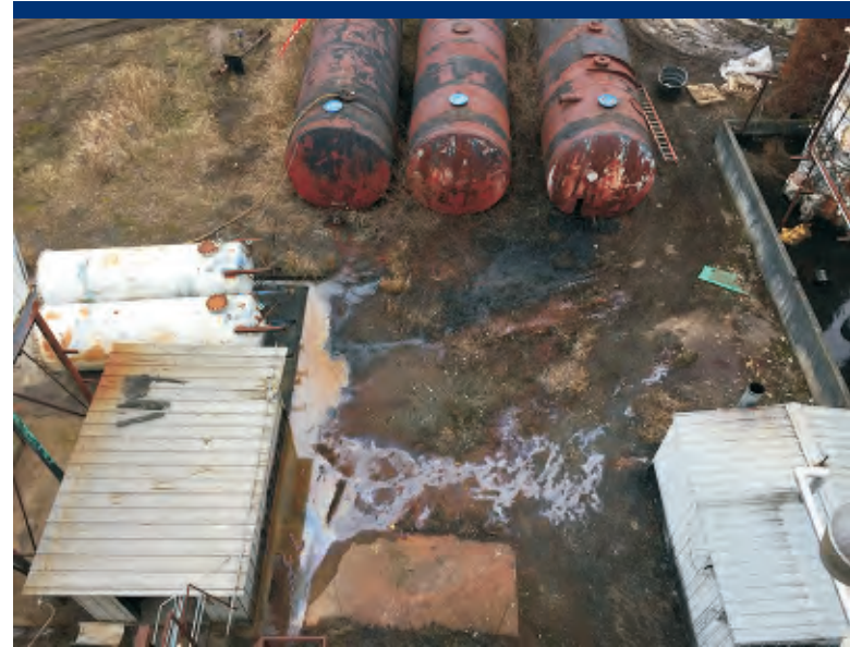
Photo 10 Impacted soil around Warehouse B and tanks T-1, T-2, and T-3.
