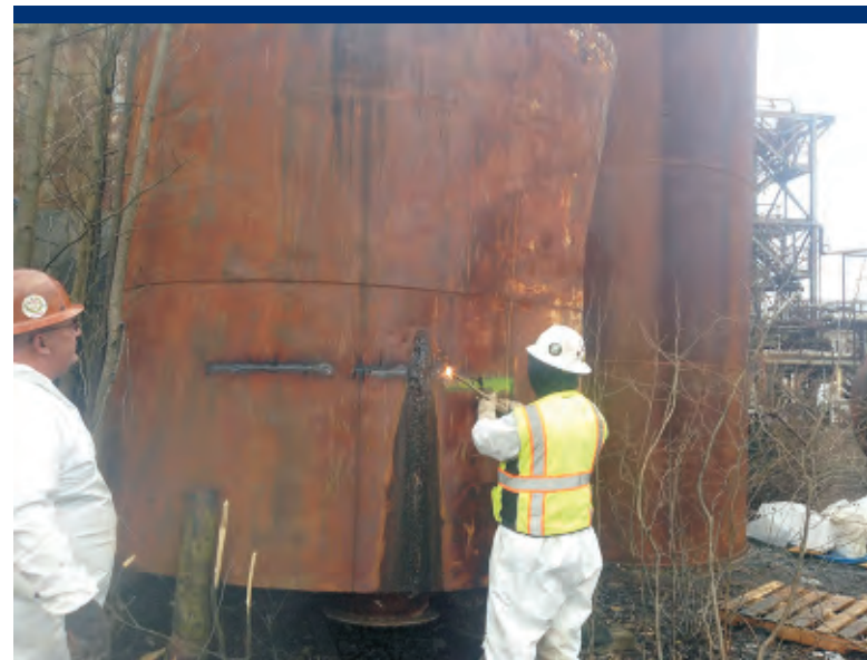
Photo 33 ERRS cutting tank for removal of drums.
