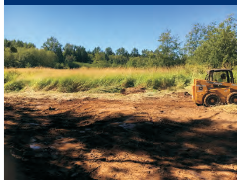
Photo 54 Post excavation of soil by ERRS.
