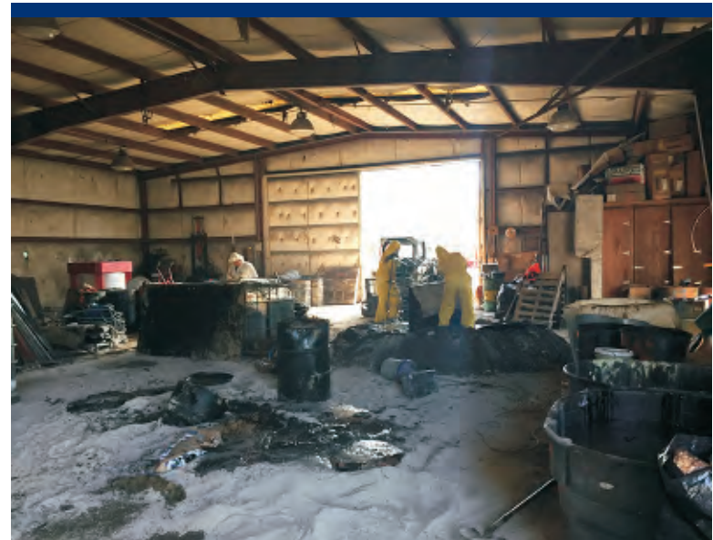
Photo 37 Sludge solidification activities in Warehouse A.
