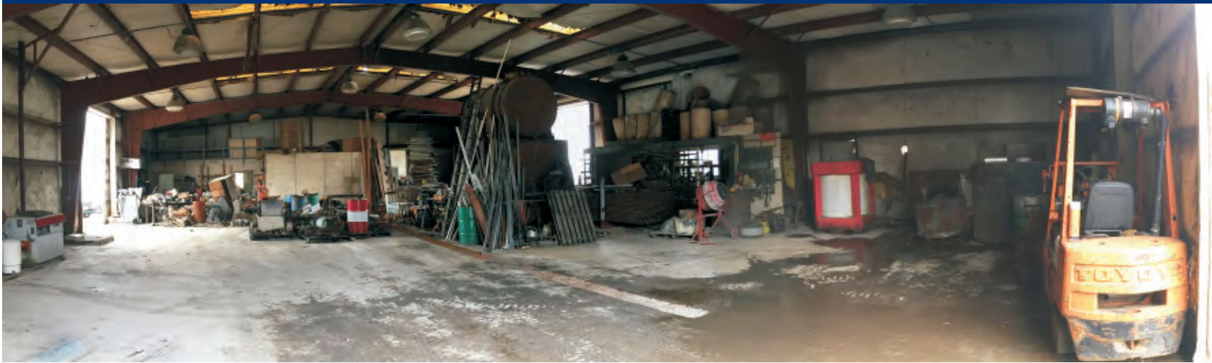
Photo 45 Final disposition of Warehouse A after removal of all OPA and CERCLA related materials.
