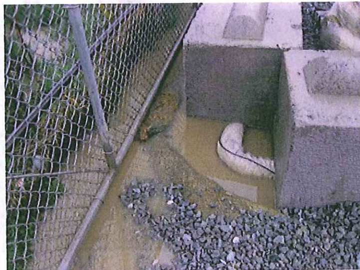
#10. DESCRIPTION: The stormwater flows from the ecology blocks to the chain link fence and then onto Myrtle Street. The quality of the stormwater was not noticeably improved on the discharge side of the fence.
