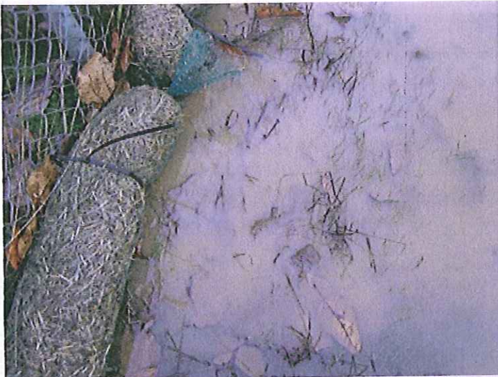
#3. DESCRIPTION: These straw wattles are on the outside (downstream) side of the fence. The wattles do not appear to improve the turbidity of the stormwater run-off.
