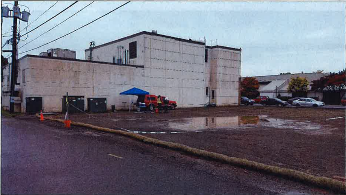
Photo 17. North and east portion site conditions at time of visit. Looking southeast from alley.
