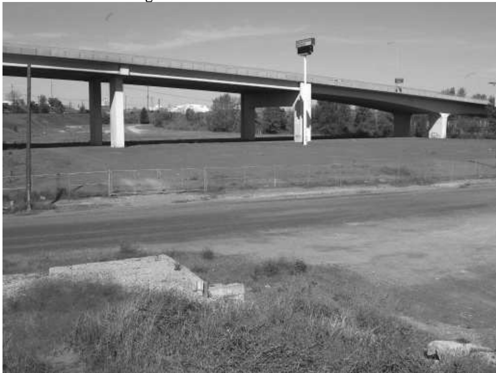
Photo 2: Hamilton Street Bridge Site – from the east
