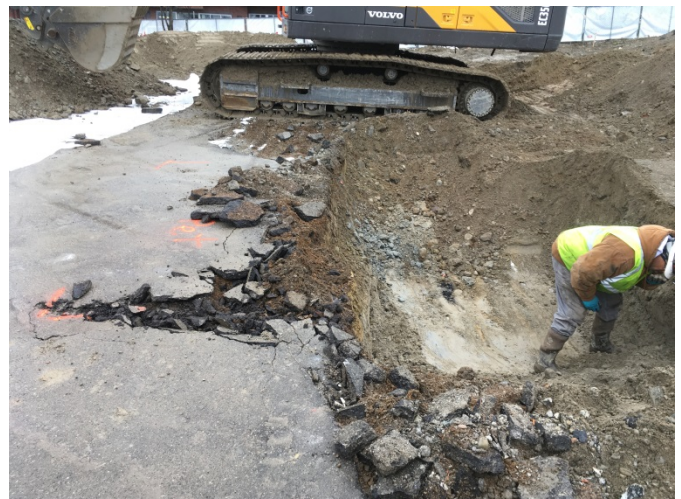
Photograph 6. Looking north. Gray-stained PCS visible on northwestern sidewall of remedial excavation area EX03.
