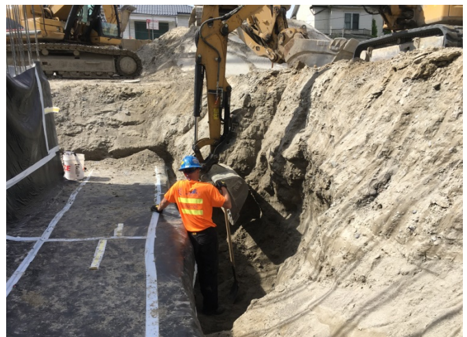
Photograph 12. Looking south. Removal of remaining PCS on west sidewall of elevator pit once elevator footing is in place.
