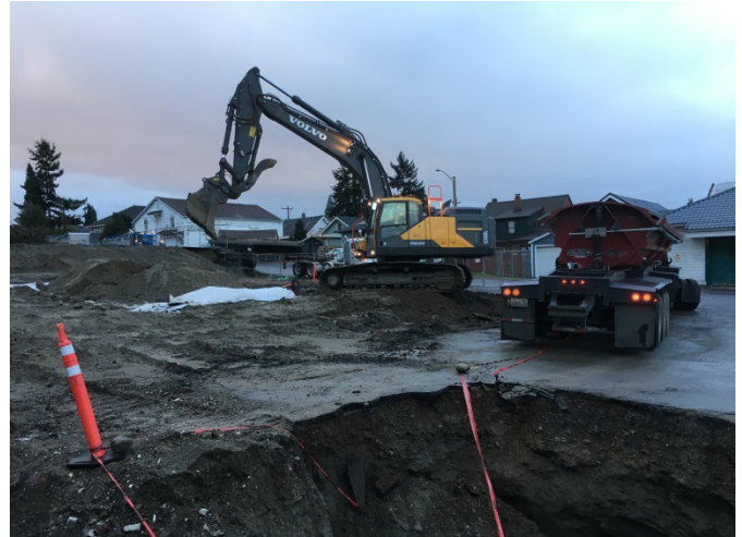
Photograph 8. Looking southeast. Loading out stockpiled class III soil from remedial excavation area EX03.
