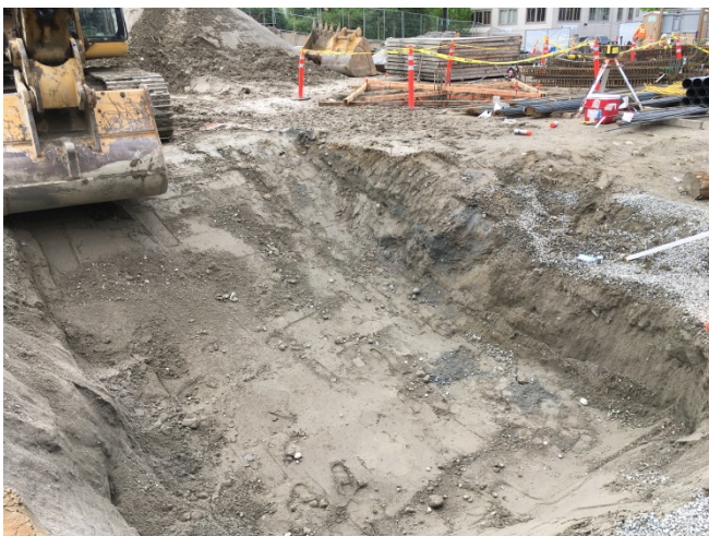
Photograph 11. Looking southwest. Gray-stained PCS visible on bottom and west sidewall of elevator pit area.
