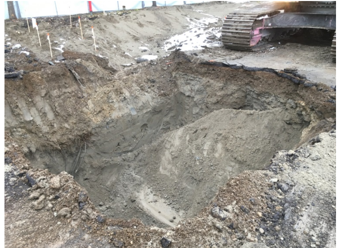
Photograph 4. Looking northeast. Final extent of remedial excavation area EX01. No PCS observed.
