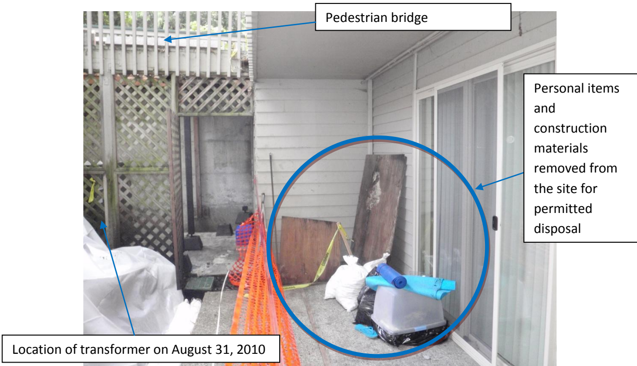
Original transformer location on September 1, 2010; after initial spill cleanup activities.
