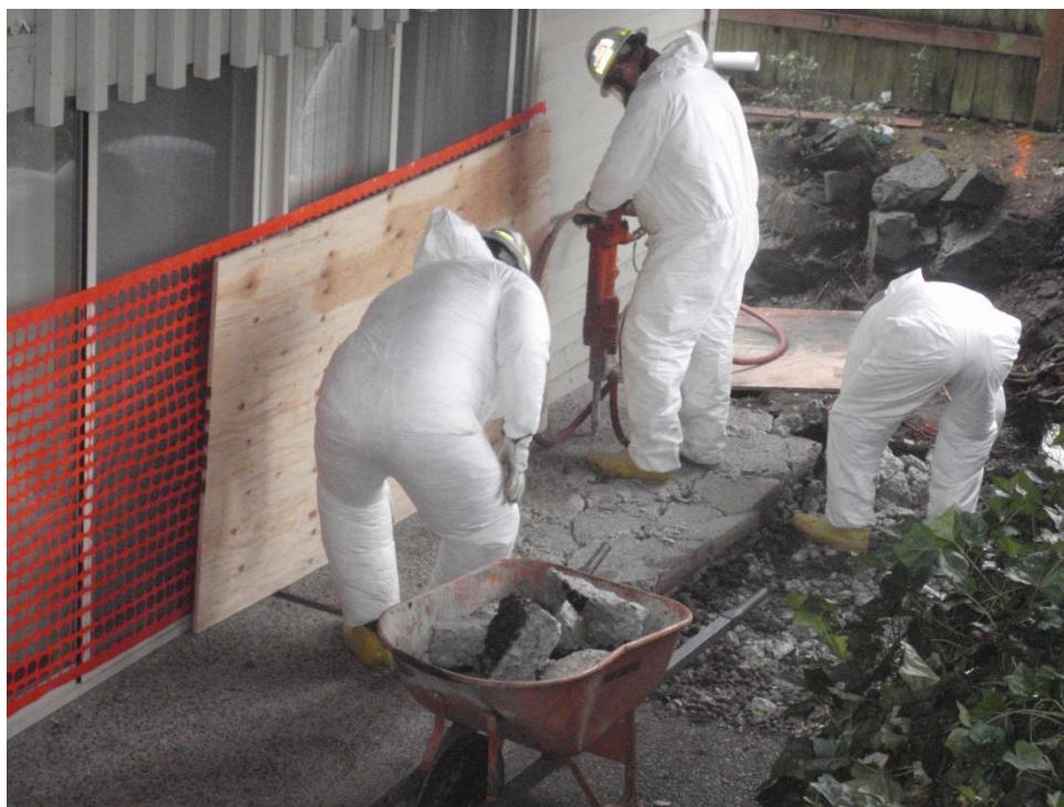
Concrete removal at patio decks during remedial activities; September 16, 2010.
