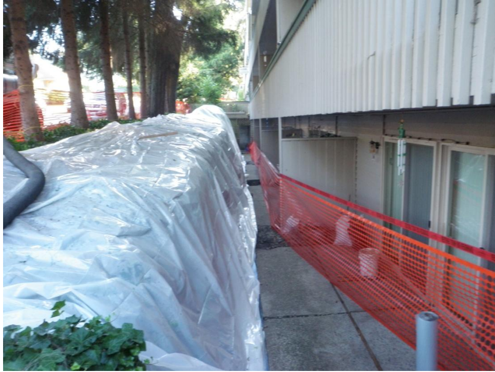
Exclusion zone to help isolate casual contact with potentially contaminated materials at the site; September 1, 2010.
