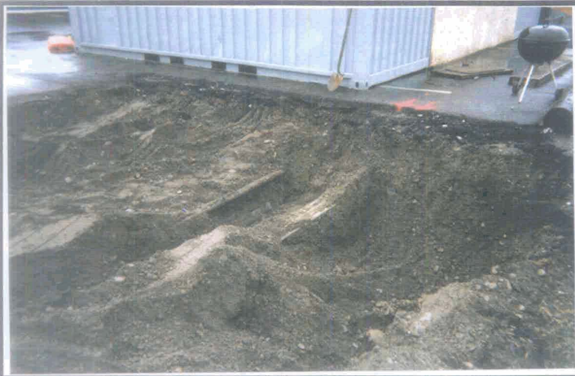
Photo 3 - Photo of the over-excavation of AST storage area (view to west)
