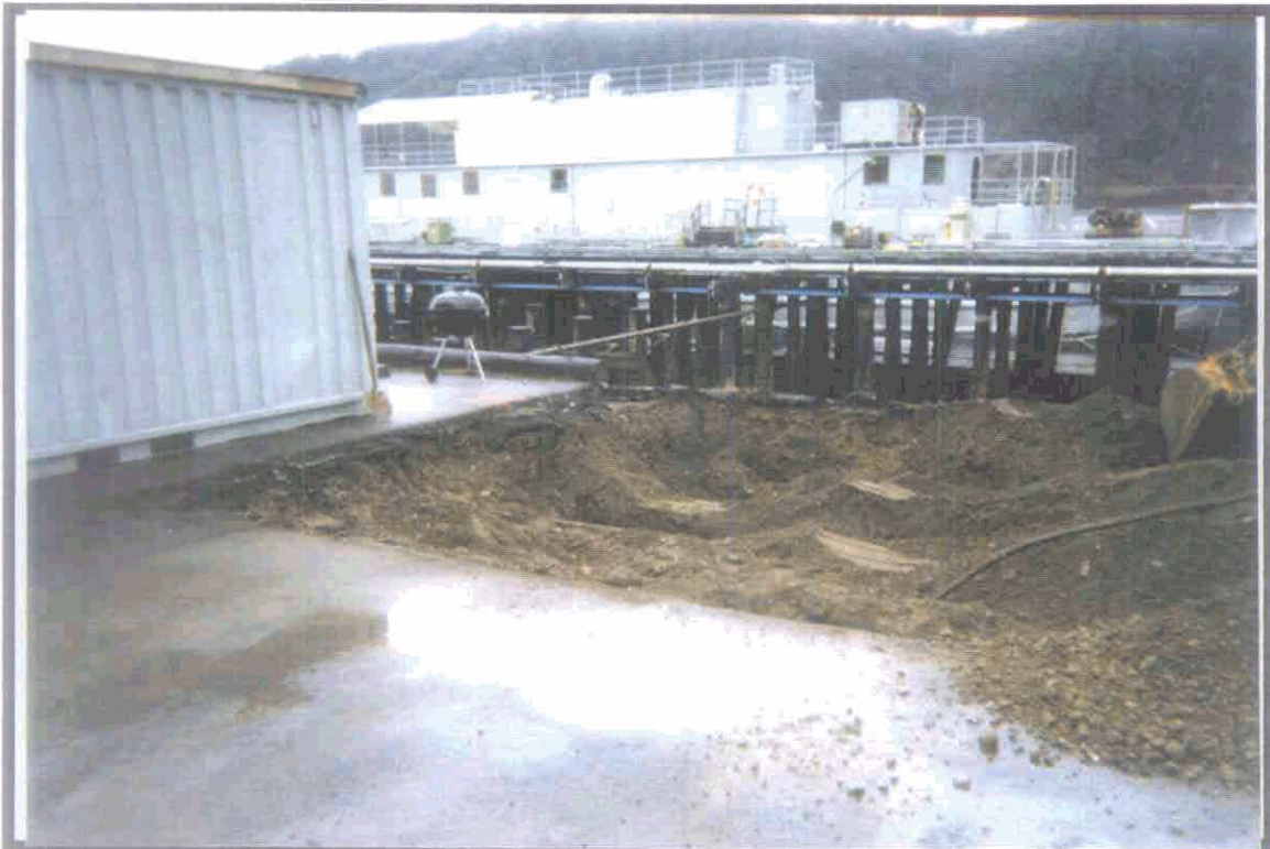
Photo 2 - Photo of the over-excavation of AST storage area (view to northwest)
