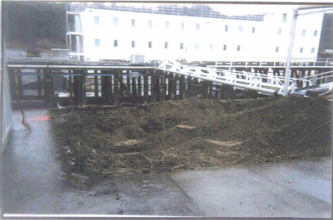
Photo 1 - Photo of the over-excavation of AST storage area (view to northeast)
