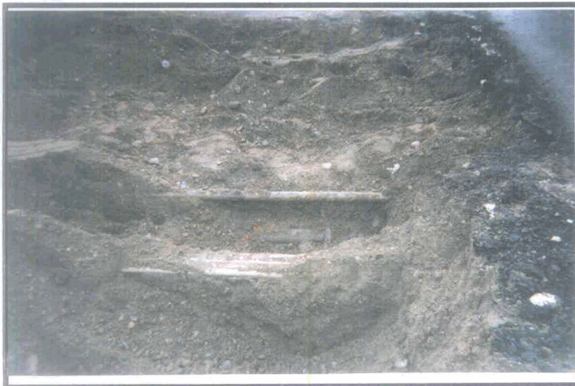
Photo 4 - Photo of the over-excavation of AST storage area (note u/g piping)
