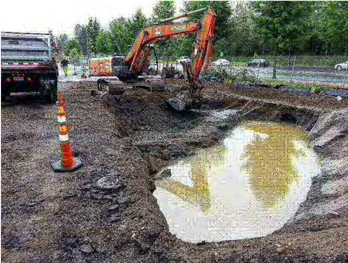
Photo #5. The leaking storm water pipe flooded the remedial excavation.
