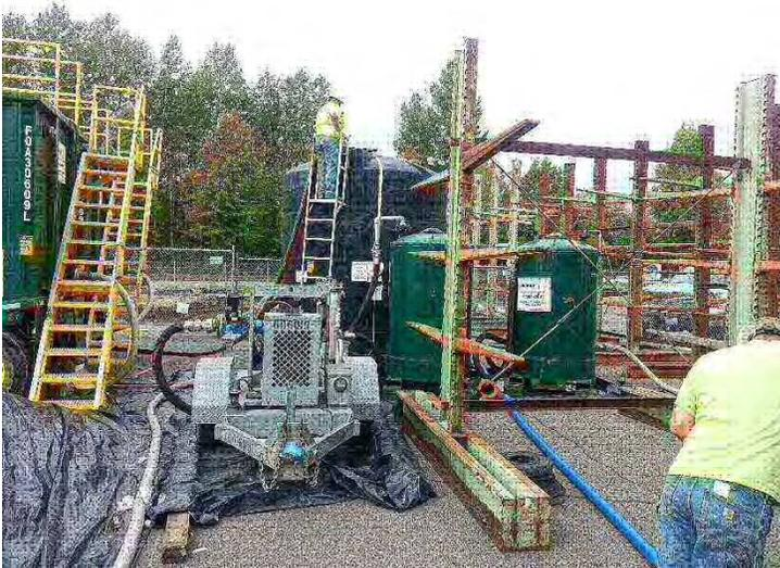
Photo #9. Dewatering effluent was treated with a sand filter and activated carbon, sampled and analyzed for TPH and BTEX, and discharged to the sanitary sewer under a King County permit.
