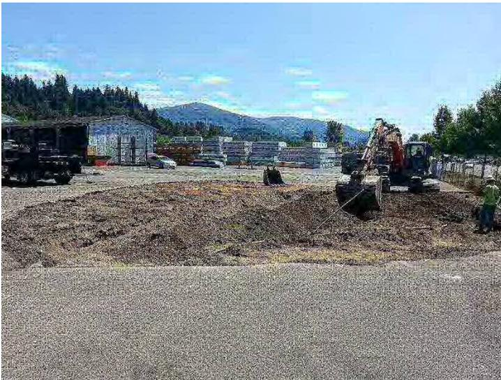
Photo #2. Removal of clean overburden fill soils.
