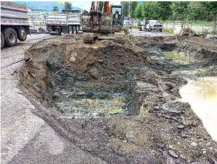
Photo #6. Impacted soil continued to be removed using temporary soil berms to retain the storm water pipe water.
