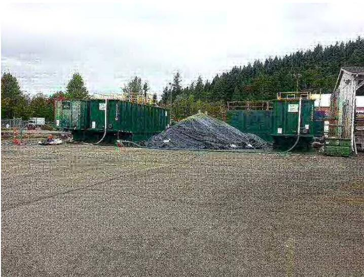
Photo #8. Dewatering effluent was stored in a series of four Baker tanks.
