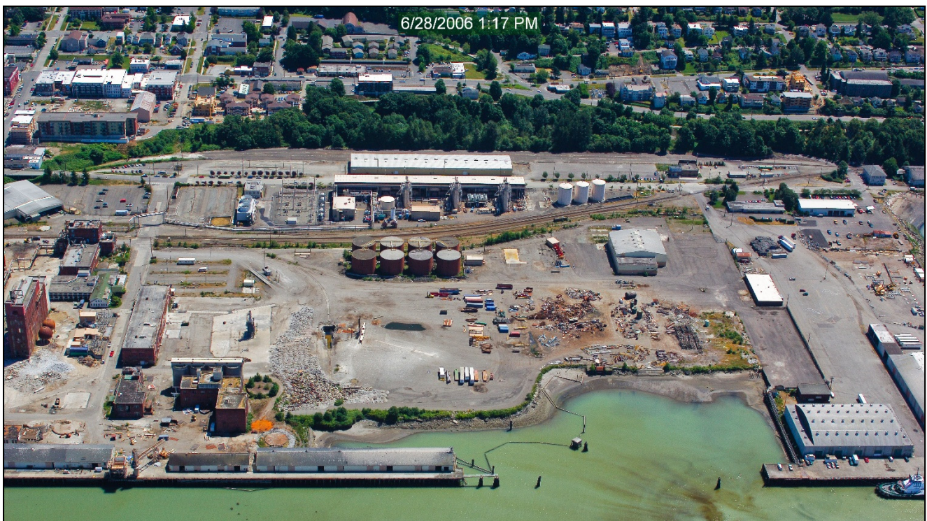
Georgia Pacific West Site, Chlor-Alkali Area facing southeast. June, 2006.
