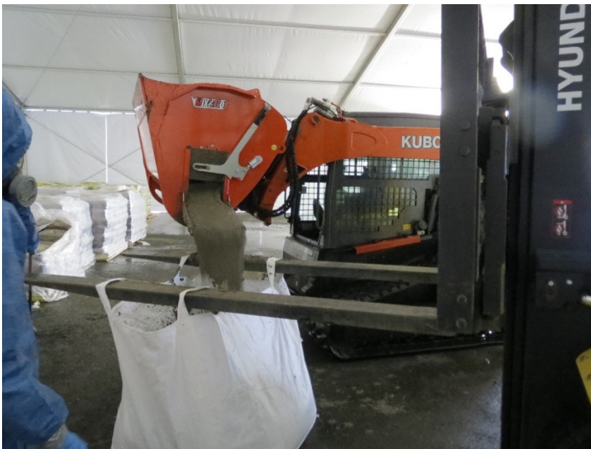
Photo 6. Discharging treated soil from mixer into Super Sack.
