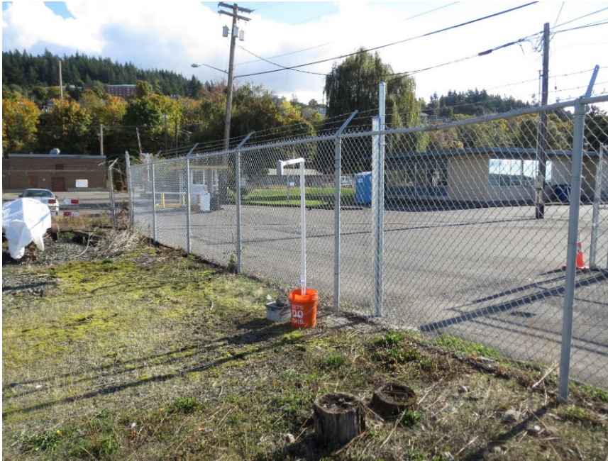
Photo 1. Perimeter air monitoring station A.
