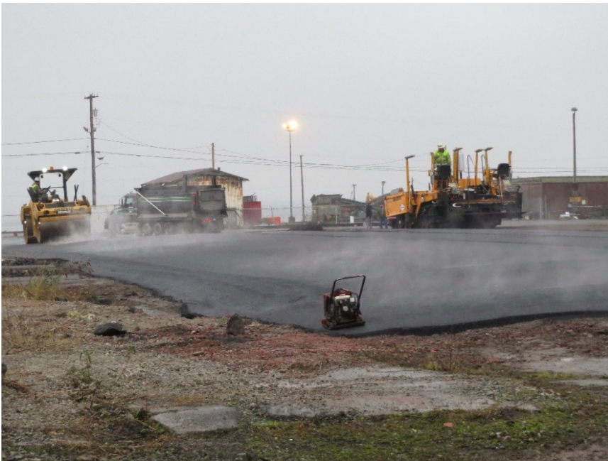
Photo 8. Paving in progress (1 st view).
