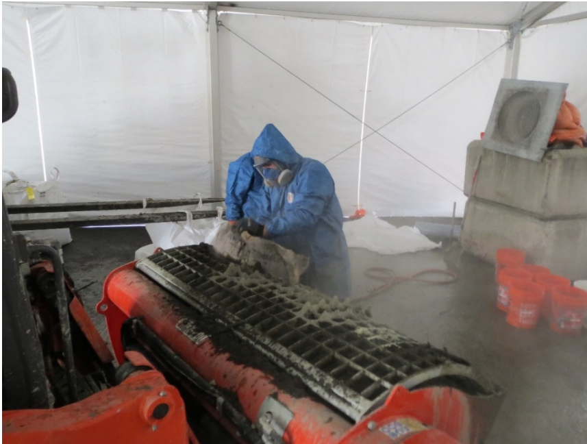
Photo 5. Adding treatment reagent (Portland cement) to soil batch in mixer.
