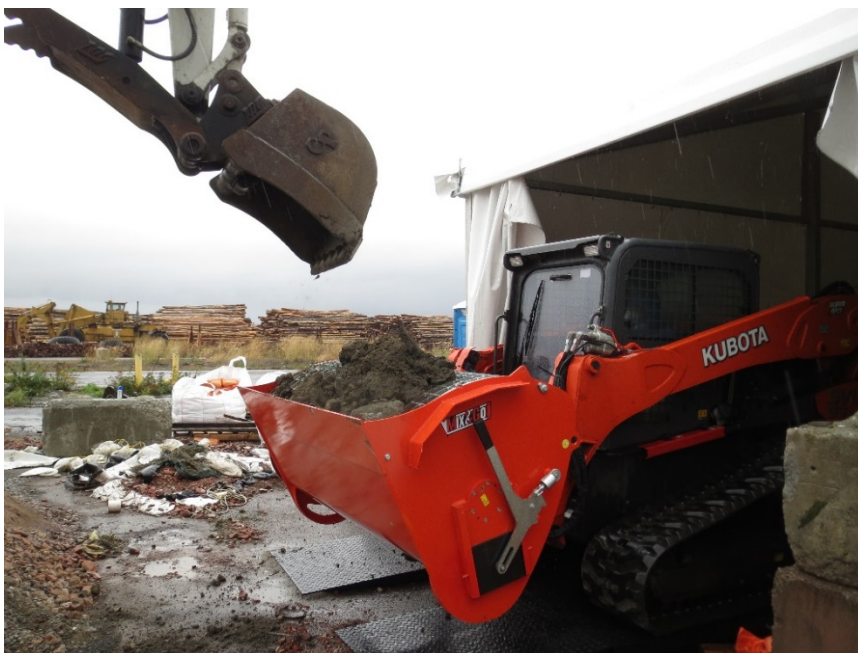
Photo 4. Loading soil/debris onto mixer mounted on skid-steer. (3-inch screen on mixer screens out oversize debris.)
