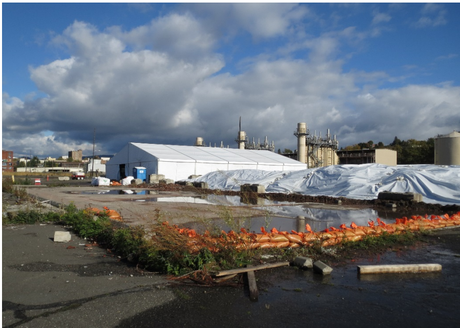
Photo 2. Contaminated soil/debris pile under white polyethylene cover, with treatment enclosure (tent) in background.
