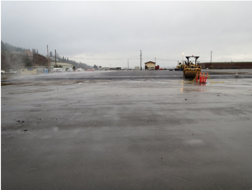
Photo 9. Paving in progress (2 nd view).
