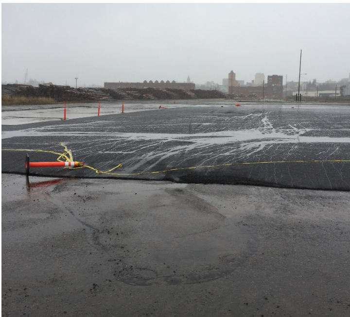
Photo 10. Finished paved surface.
