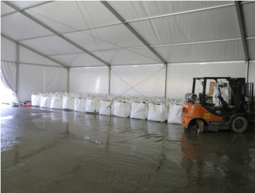
Photo 7. Treated soil curing in Super Sacks.
