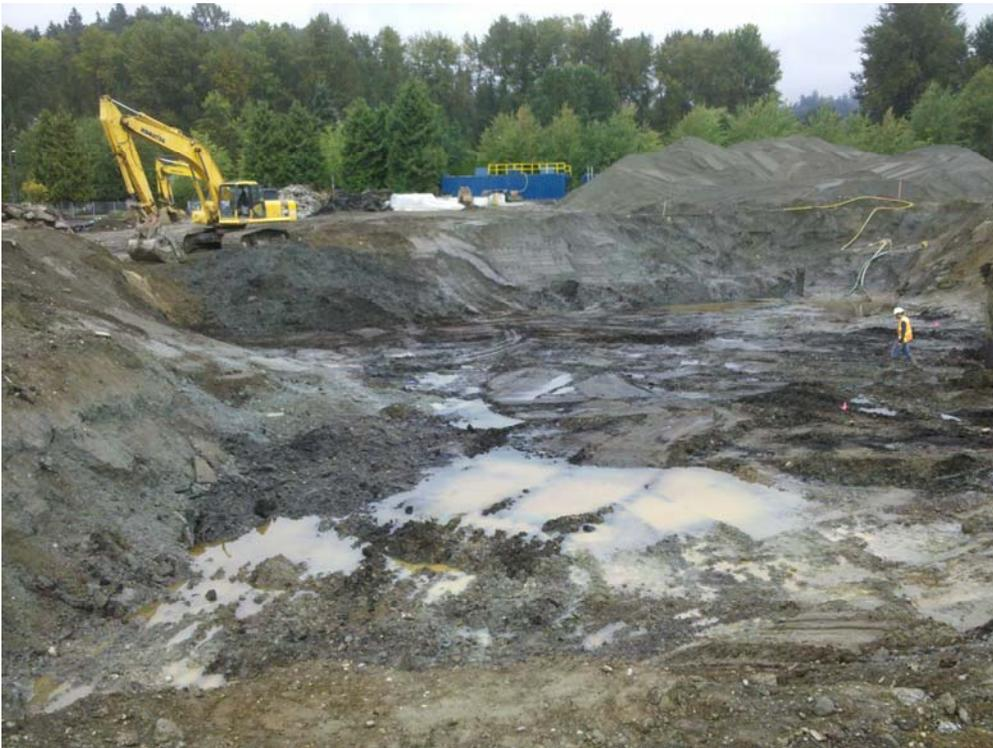
Photo 2 – Peat layer and water table exposed in southern extent of excavation (looking to south) on September 17, 2010.
