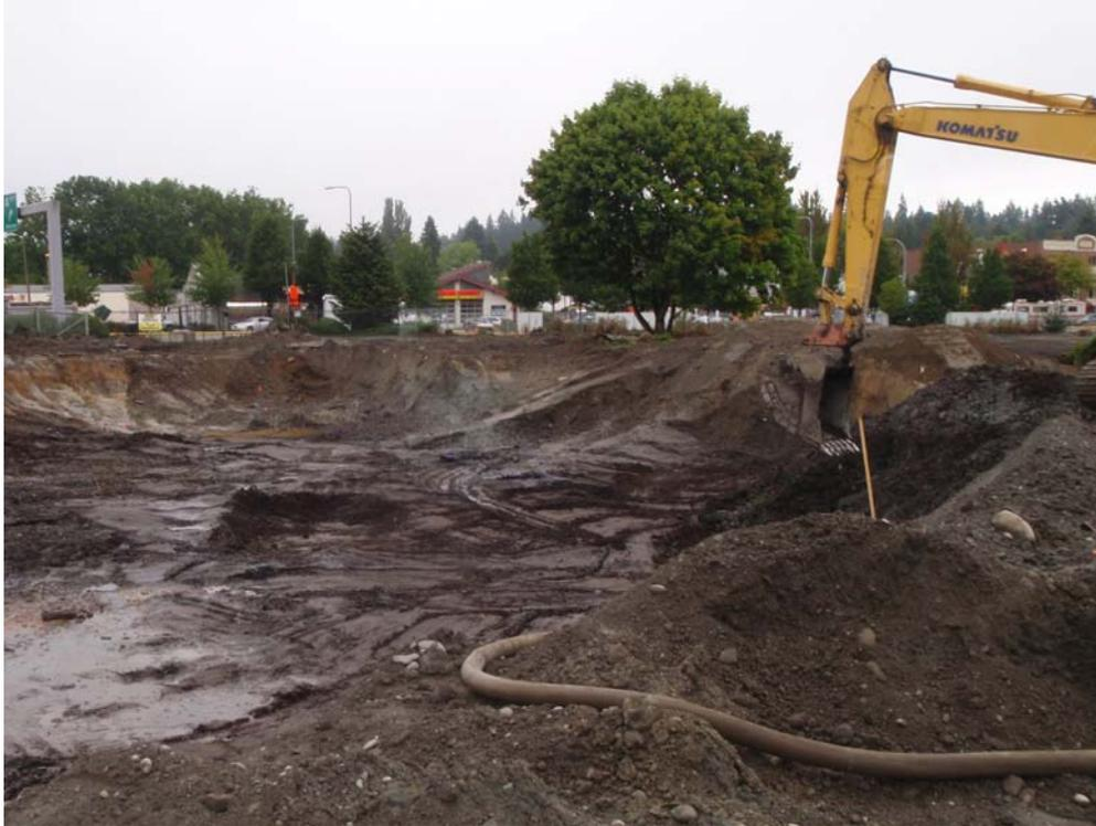
Photo 3 – Peat layer and water table exposed in northern extent of excavation (looking to north) on September 17, 2010.
