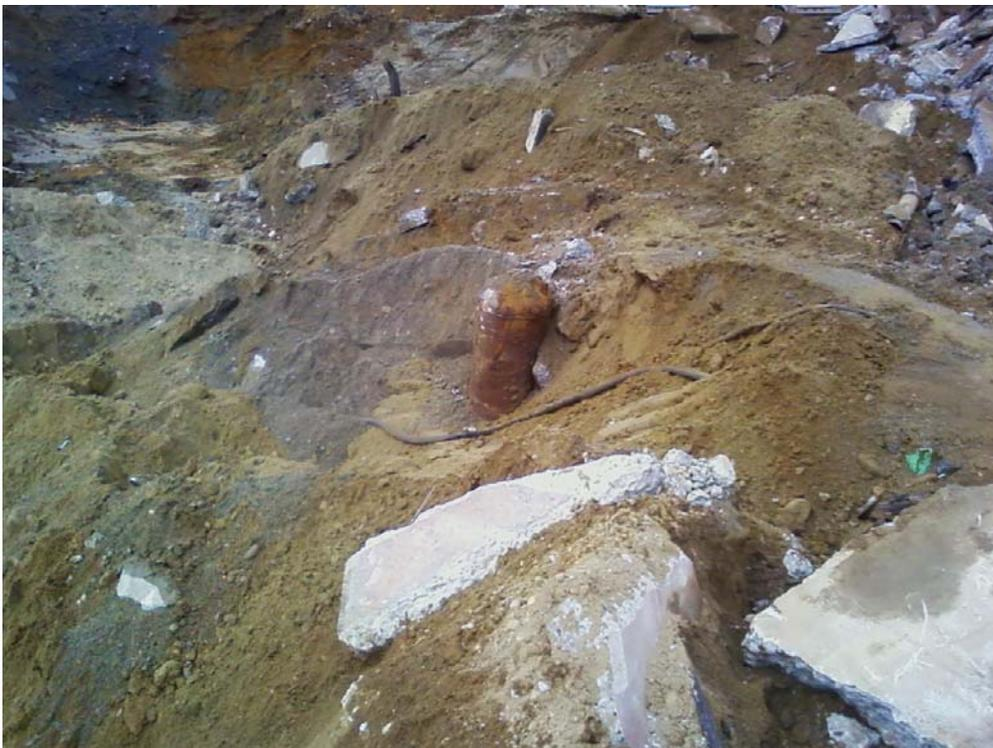
Photo 4 – Old hydraulic lift exposed on September 7, 2010.
