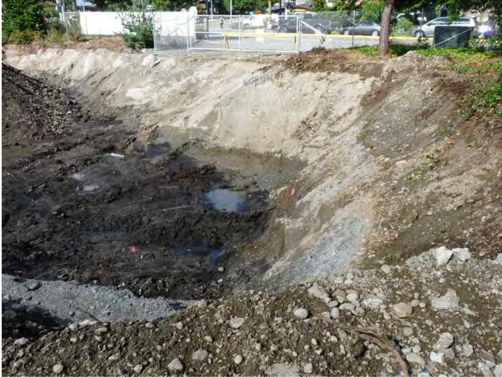
Photo 1 – Excavation limit looking north to SR 522. Note peat layer on excavation floor. Extent of excavation was limited to maintain the structural integrity of SR 522 and related sidewalk and utilities
