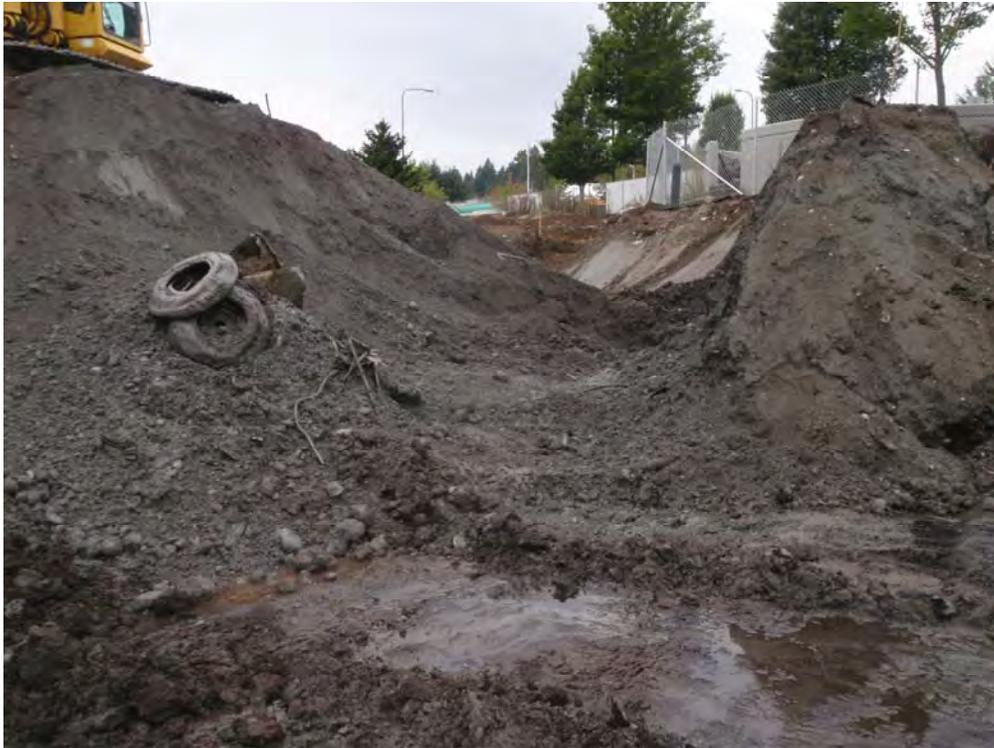
Photo 3 – Buried debris in west end of excavation below Rotunda Park (looking to northwest)
