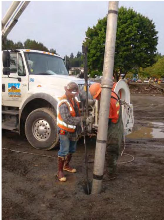
Photo 6 – Using a vactor truck to excavate an exploration borehole adjacent to Horse Creek culvert
