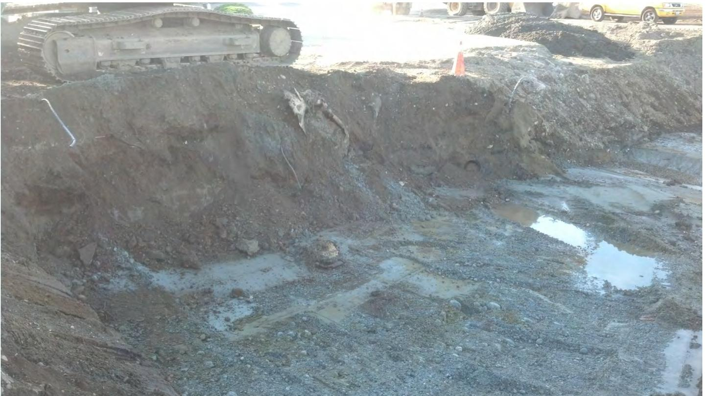
Photo 21 – UST exposed during remedial soil excavation. Tank end is visible in sidewall below excavator track.
