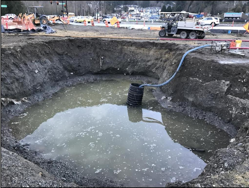
Photograph 1: View facing west toward the final boundaries of the 2017 Bothell Landing remedial excavation. Photograph taken prior to pumping water that had accumulated in the excavation.
