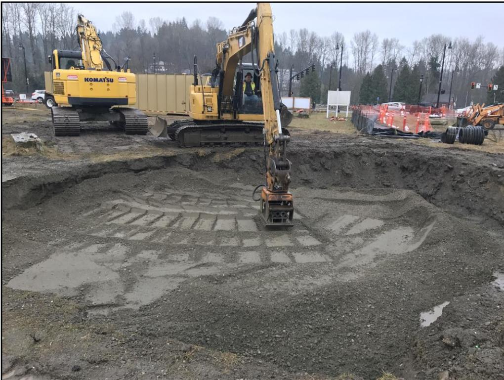
Photograph 2: View facing south toward the 2017 Bothell Landing remedial excavation during backfilling activities. Brown Baker tank utilized for storing water pumped from the excavation visible in the background.
