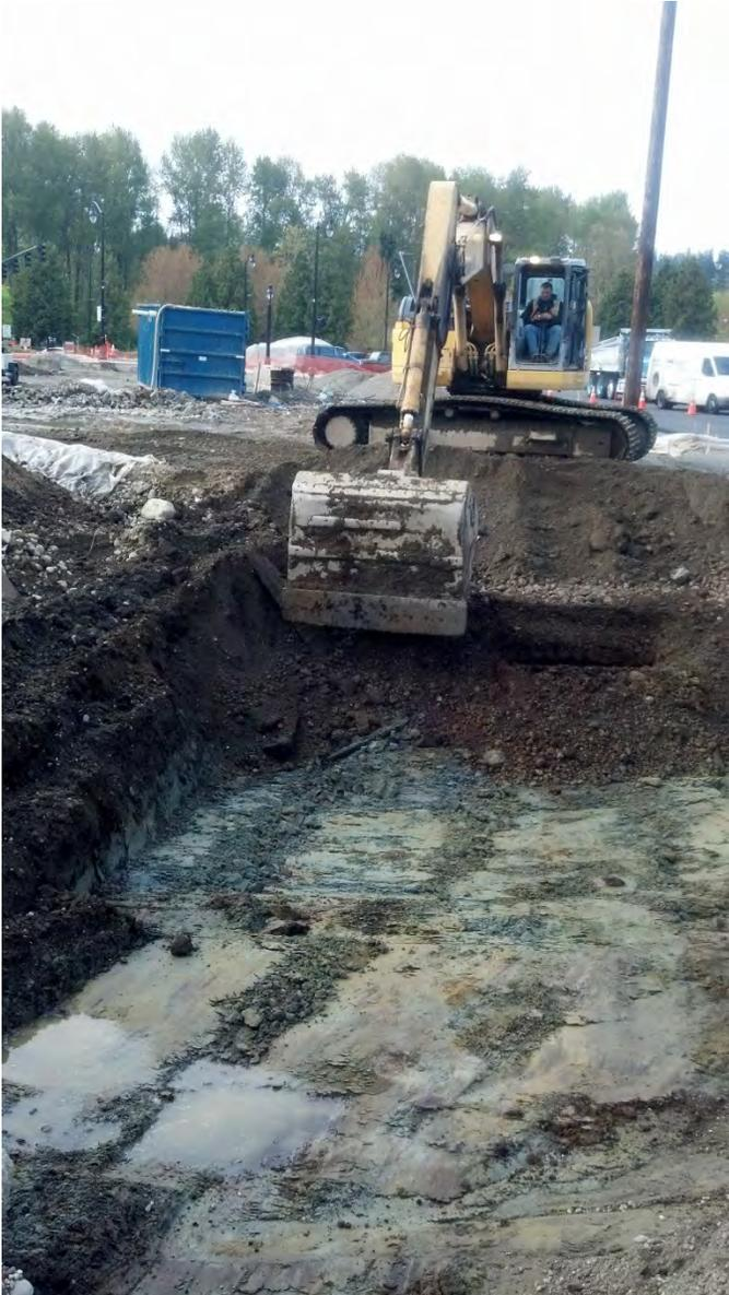
Photo 16 – Excavation along east side of SR-527, showing native soils
