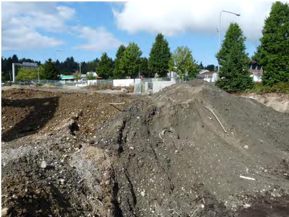
Photo 4 – Buried debris in west end of excavation below Rotunda Park (looking to northwest)
