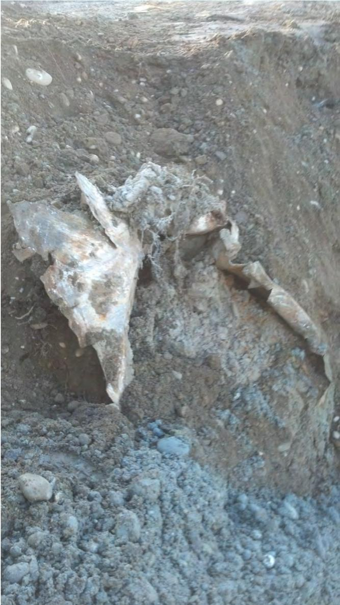
Photo 22 – Detail of UST end and underlying soils
