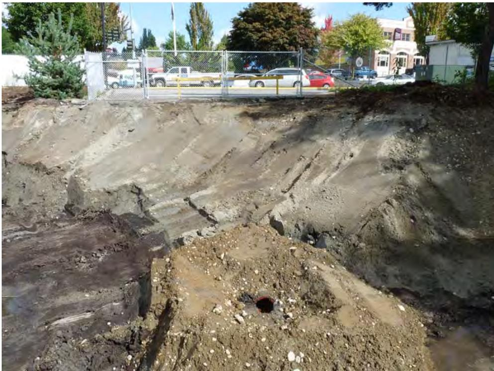
Photo 2 – Uncovered abandoned storm drain pipe in northeast corner of excavation
