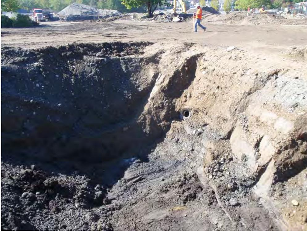
Photo 5 – Exposed abandoned storm drain side connection to Horse Creek Culvert in western extent of excavation (looking southwest)
