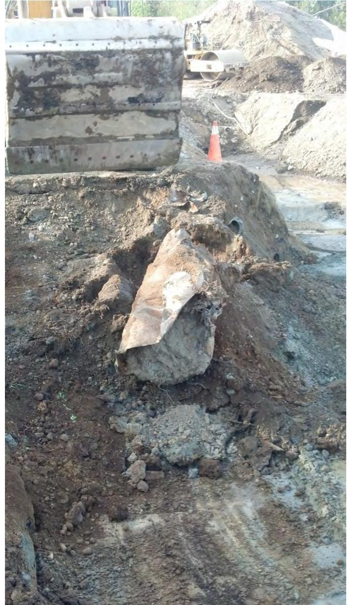
Photo 23 – UST during removal for ongoing soil excavation
