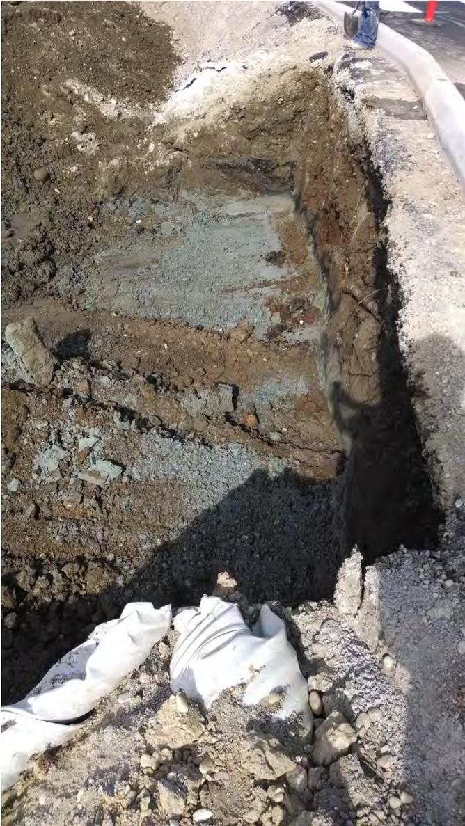
Photo 26 – Overexcavation of soils adjacent to and underlying Main Street
