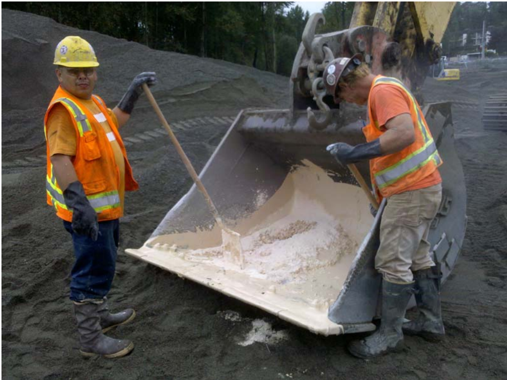
Photo 6 – Mixing ORC in an excavator bucket.
