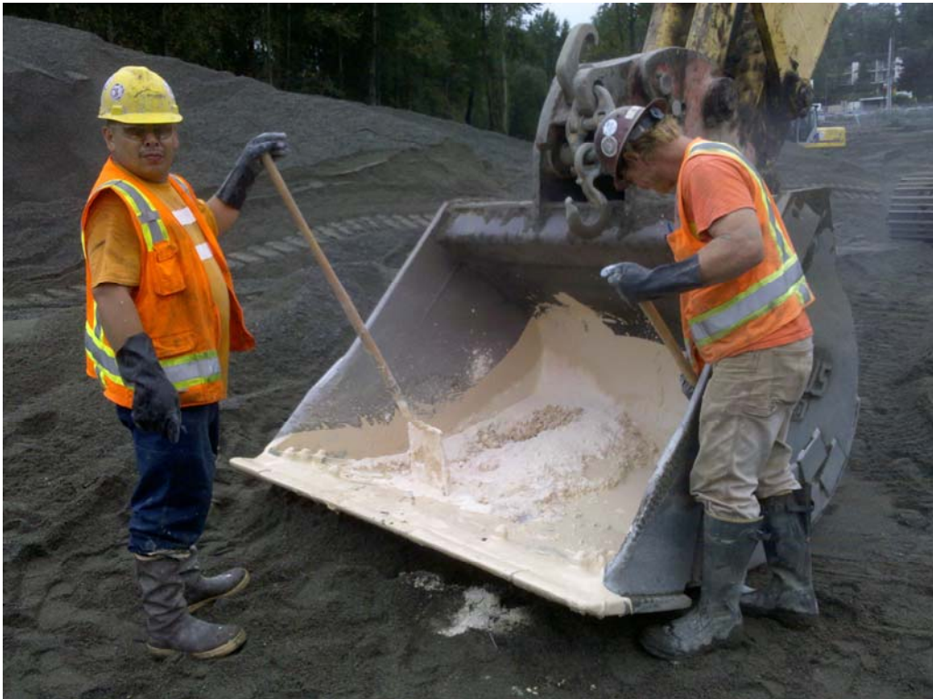
Photo 6 – Mixing ORC in an excavator bucket.
