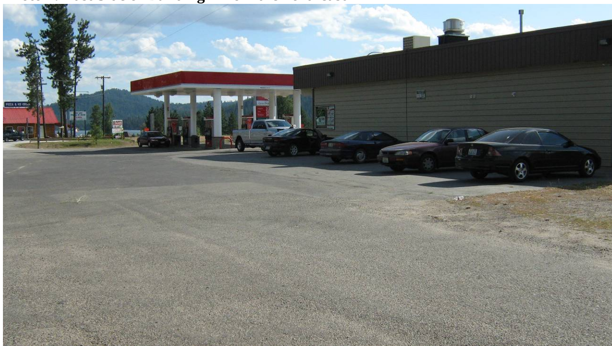
Photo 4: East Side of Building – from the northeast
