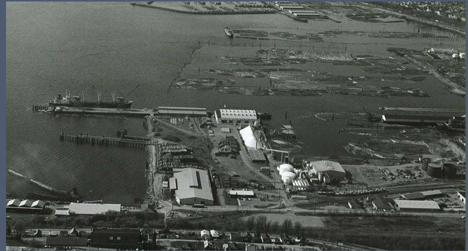
GP West Site, Chlor-Alkali Area facing northwest, 1969.
