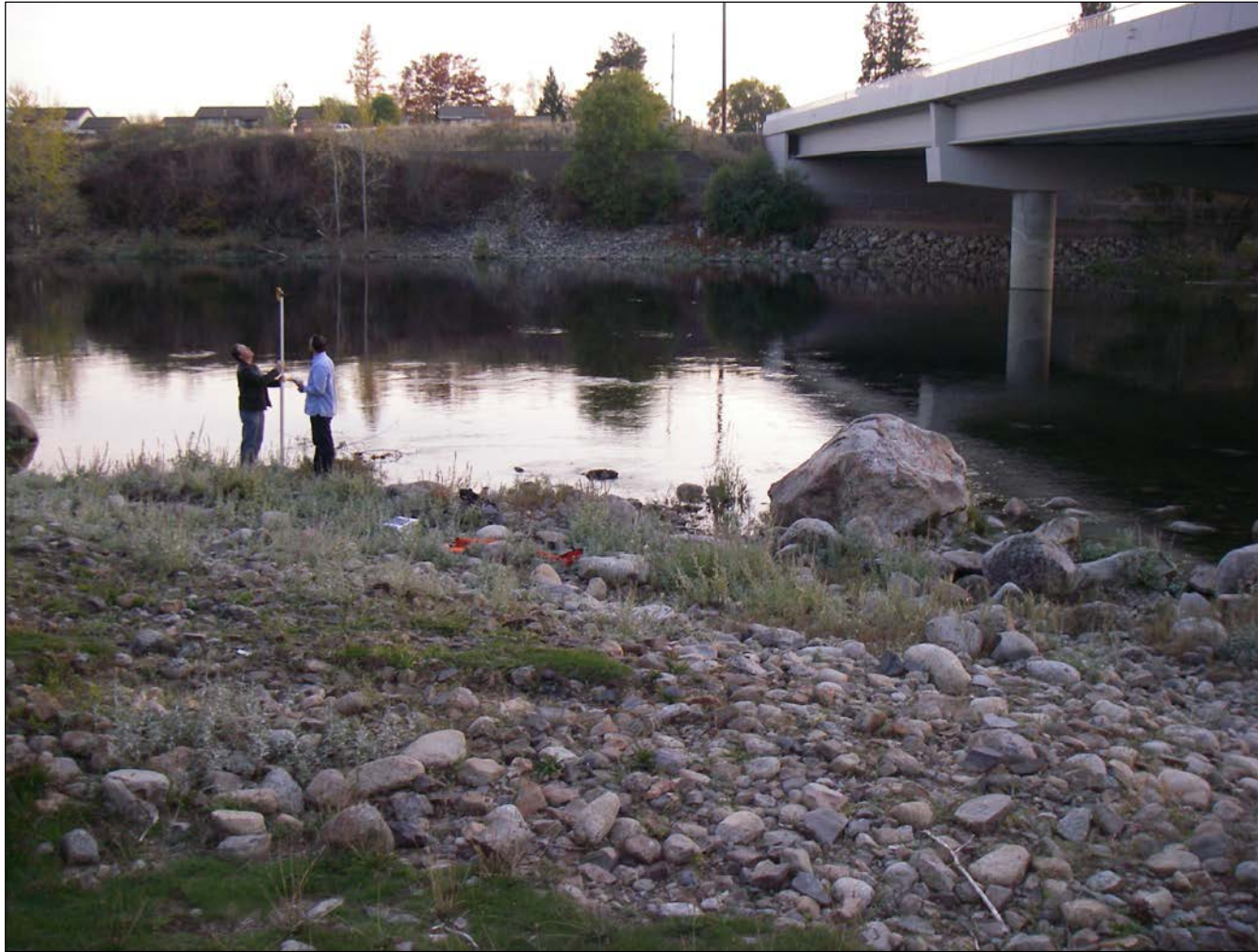
View of project site and Barker Road Bridge. Photo taken from north bank of the Spokane River, facing south.
