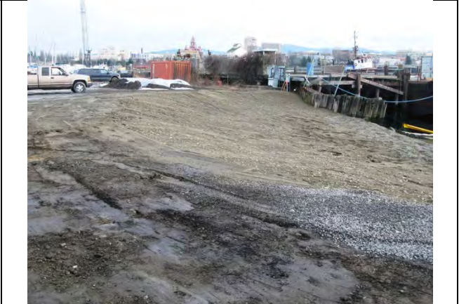
Comment: Final grade looking northeast.
