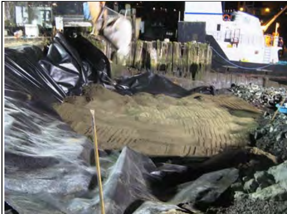
Comment: Crew placing sand cap.
