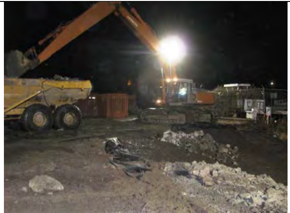
Comment: Placing armor rock on filter gravel.
