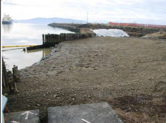
Comment: Final grade looking southwest.
