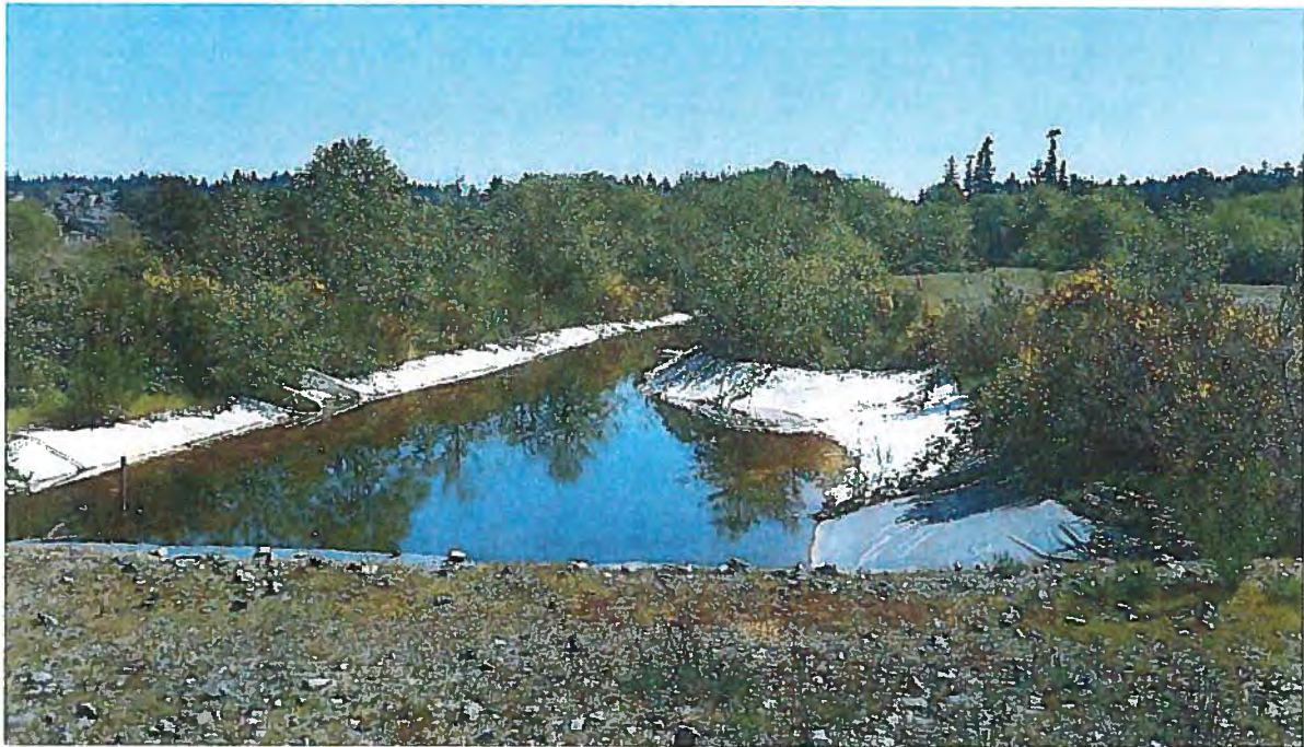
Detention Basin No. 2
