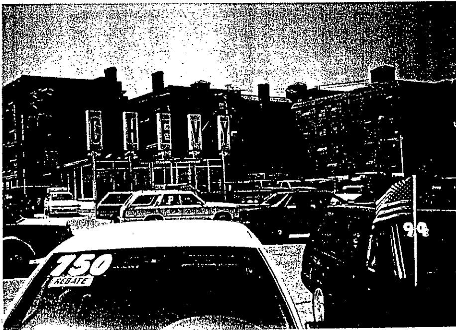
SITE PHOTOS BISON ENVIRONMENTAL NORTHWEST, INC. PROJECT# 94481 AUGUST 1994
