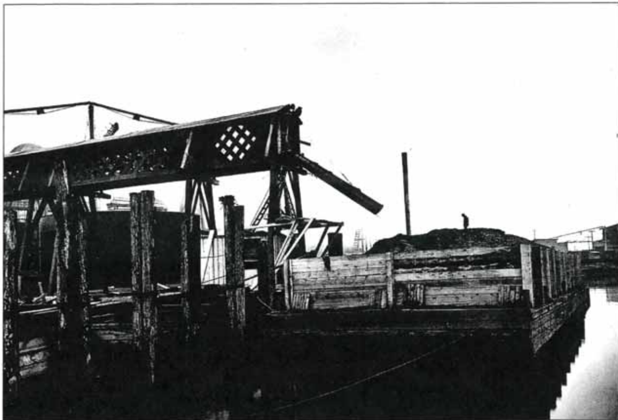
Photo 1920A. Storage tank (left half of photo) at the former creosoting plant site.
