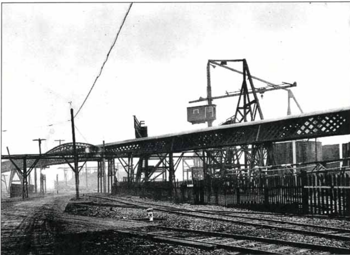
Photo 1920B. Former creosoting plant site tanks and structures (right half of photo)
