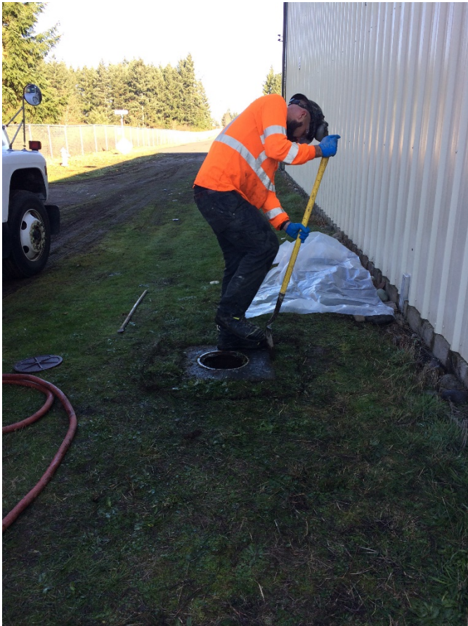
Removal of steel monument
