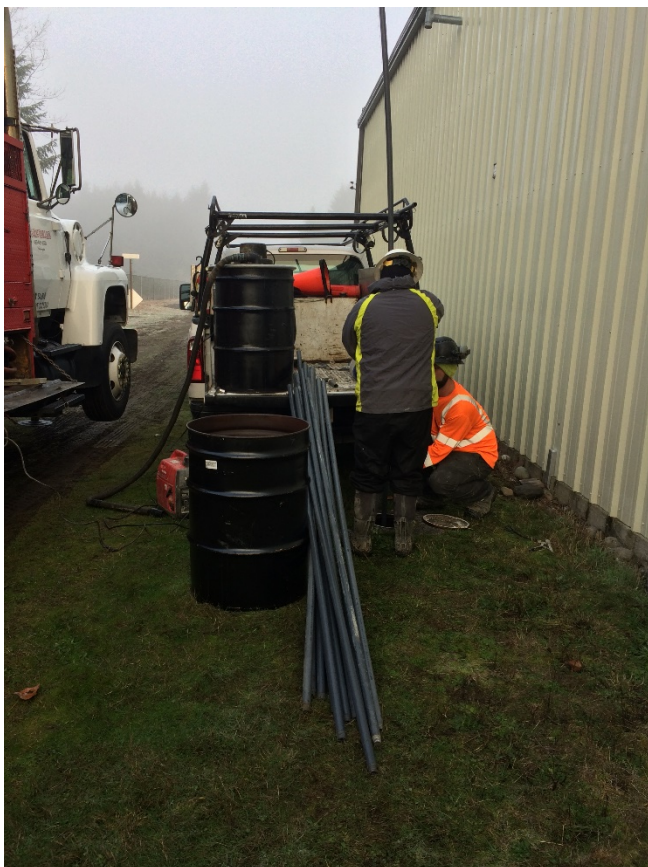
Placing tremie pipe
