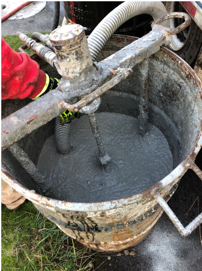
Mixing bentonite grout slurry for well abandonments
