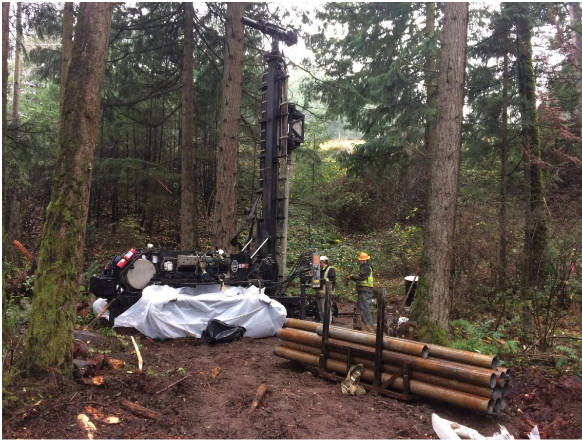
Drilling location for new monitoring well MW-29S
