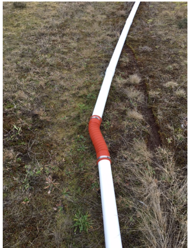
Replaced flex hose at N-13
