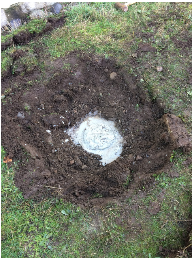
MW-25D with steel monument removed
