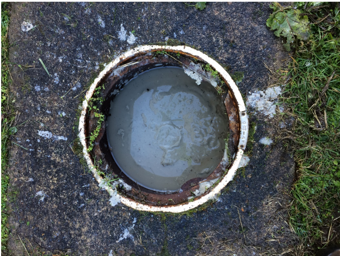
MW-25D after grouting
