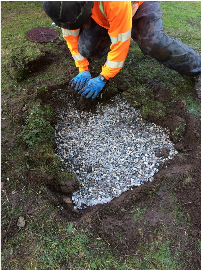
Placement of gravel underneath surface material
