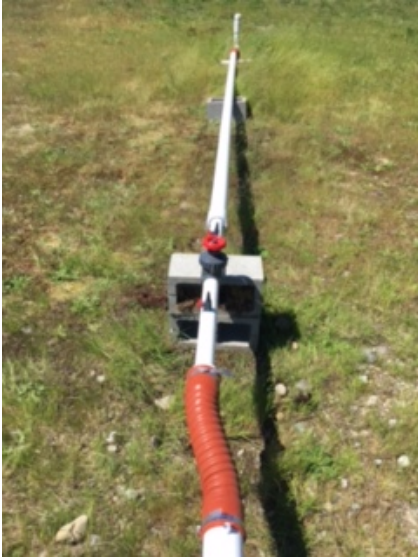
Repairs at E-42
