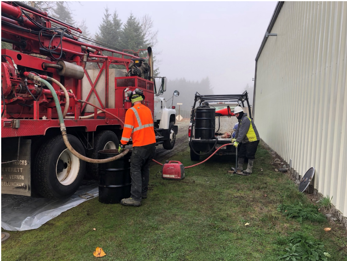
Grouting MW-25D using tremie pipe
