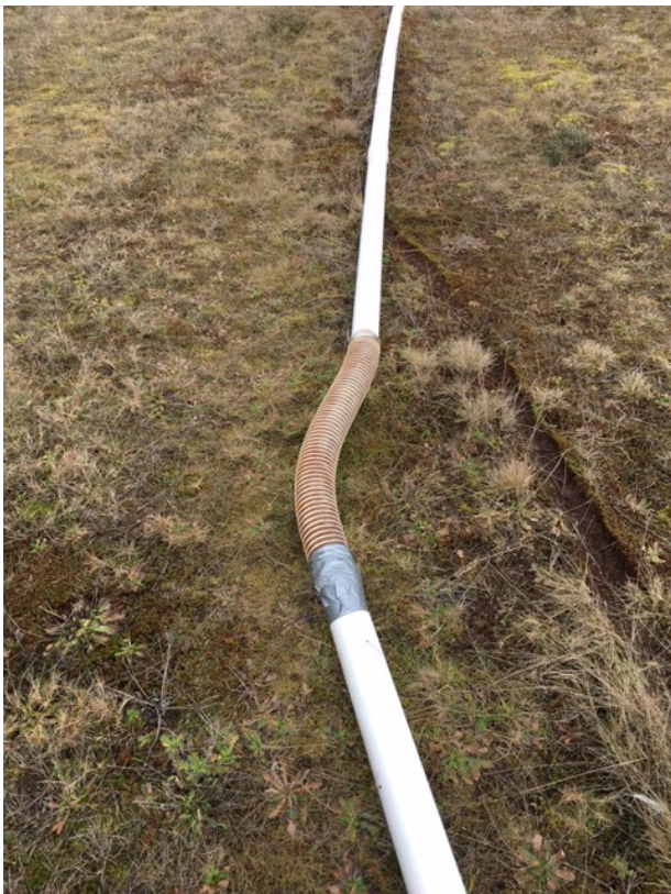
Replaced flex hose at N-13
