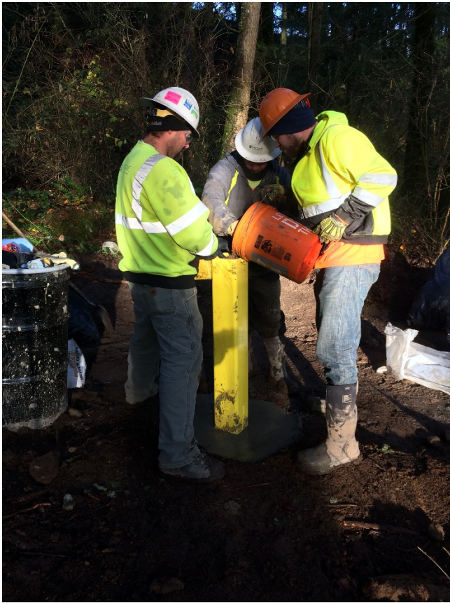
Construction of monitoring well MW-29S
