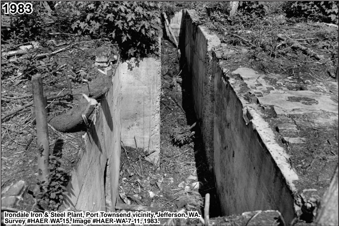
14-inch Rolling Mill Fly Wheel Pit Foundation.
