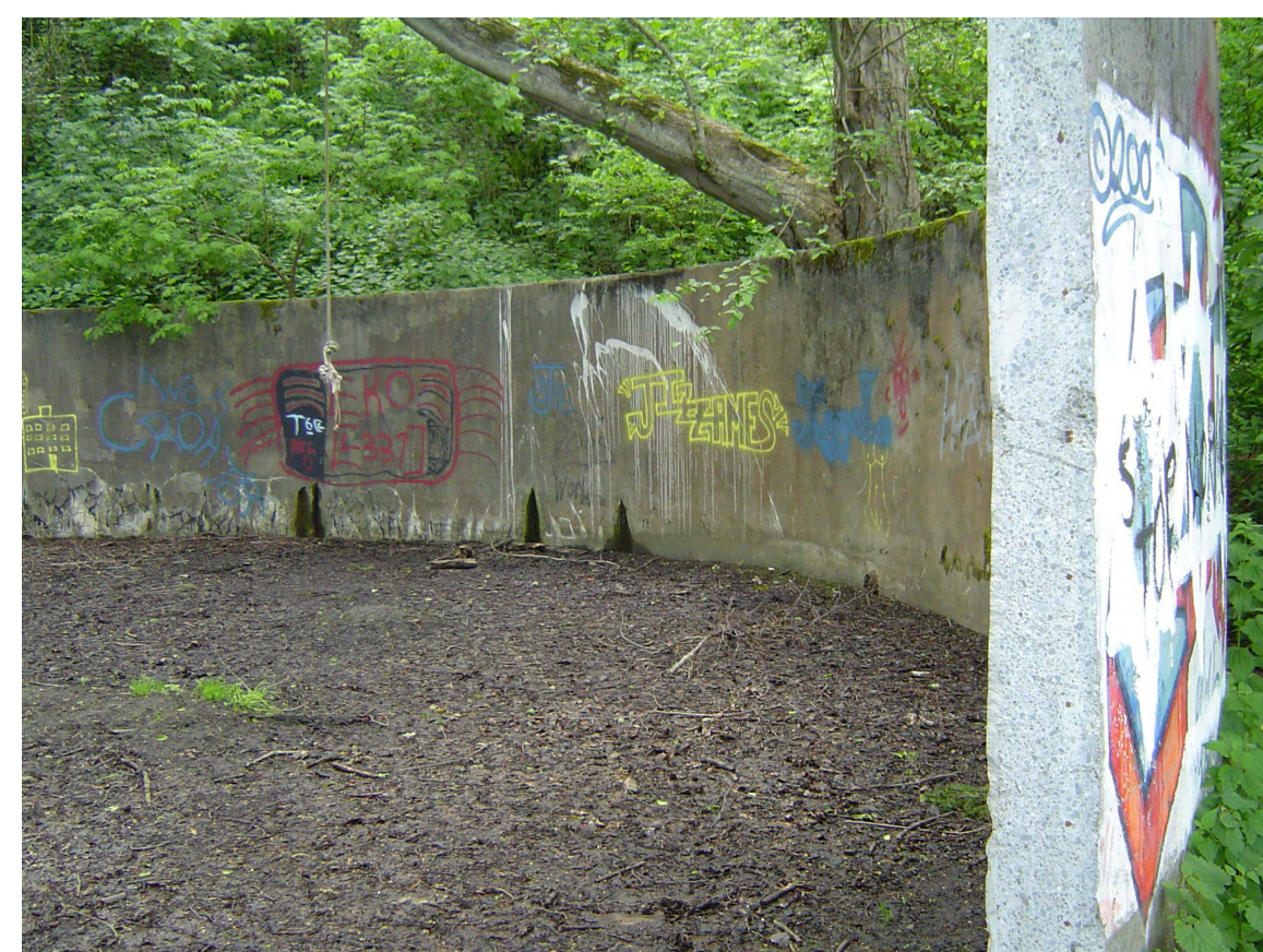
P-11 VIEW OF CONCRETE TANK WALL.
