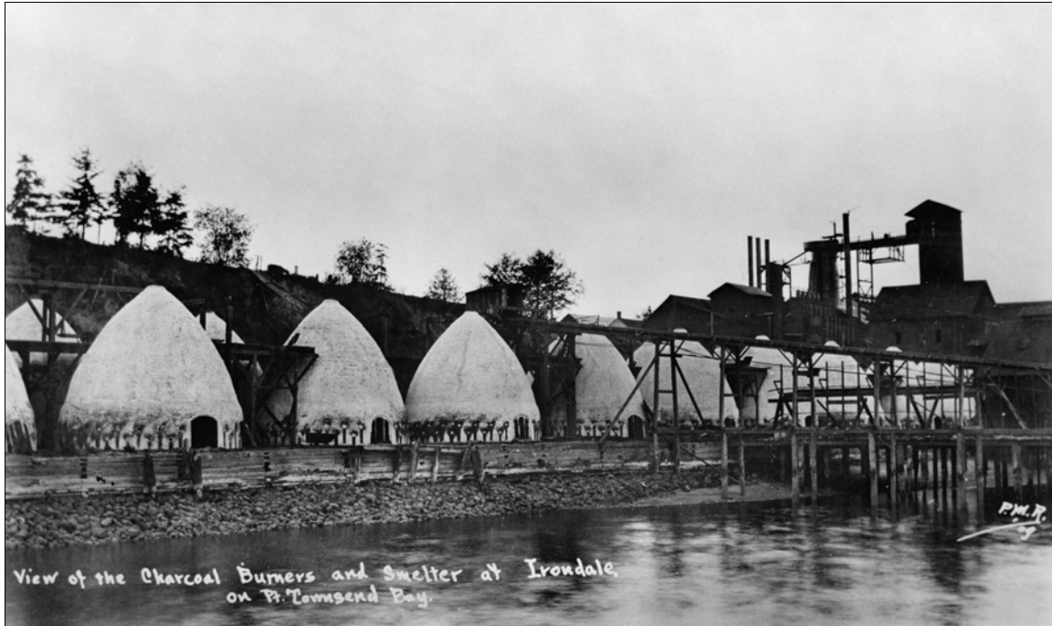
Figure 11. Overview of the Irondale charcoal kilns, view to the northwest (Britton and Britton 1983: Photograph 24).
