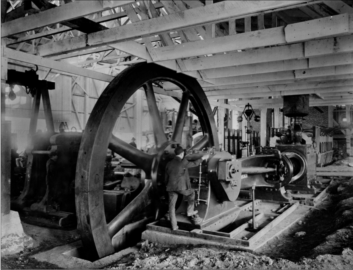
Figure 4. Overview of the 1800 horsepower Corliss steam engine and flywheel for the 22-inch Rolling Mill, 1910.
