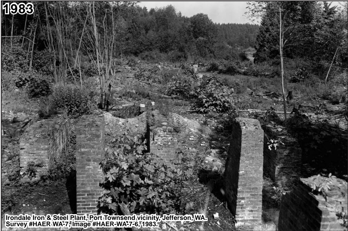
Steel Plant Site, view to North.
