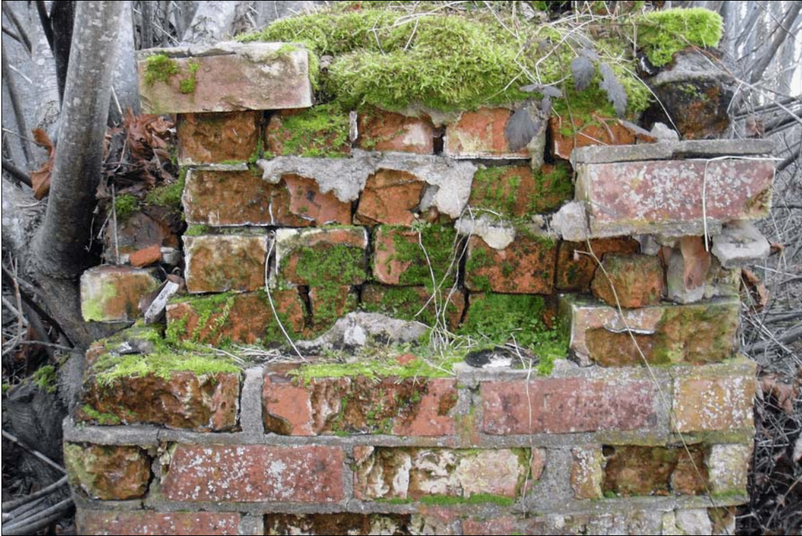
Figure 22. The west side of a brick and mortar masonry foundation at Unidentified Foundation Feature #2, west side of Steel Production Building.
