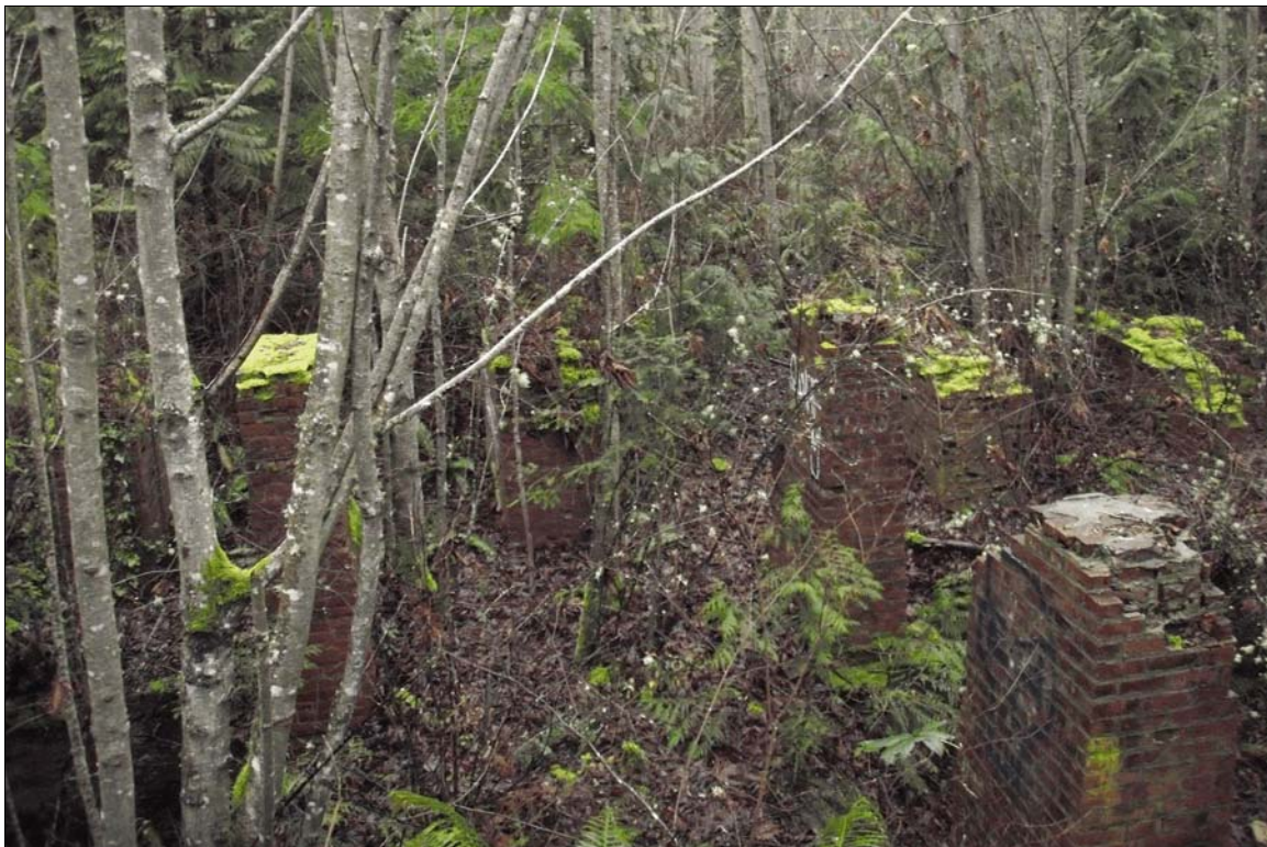
Figure 13. Overview of the charging aisle and open hearth furnace foundations, view to the north.
