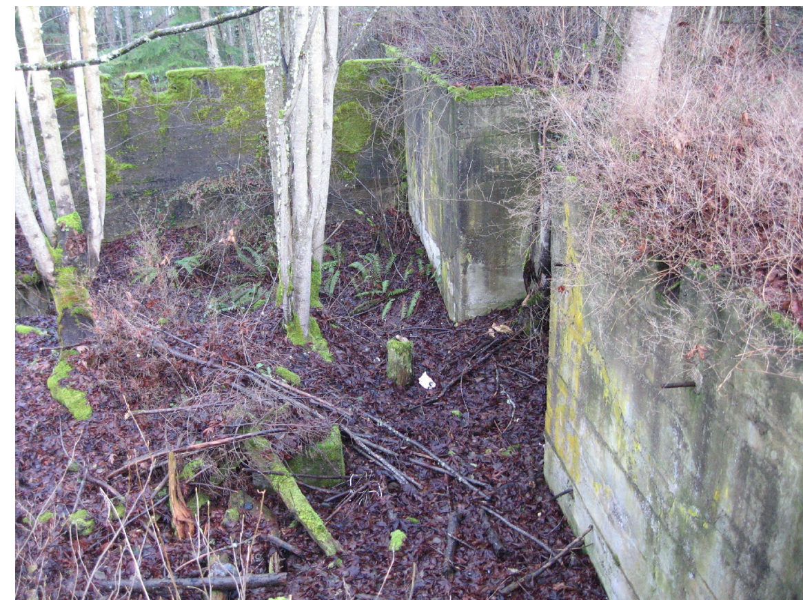
P-6 VIEW INSIDE STEEL PRODUCTION BUILDING TO BE CAPPED.
