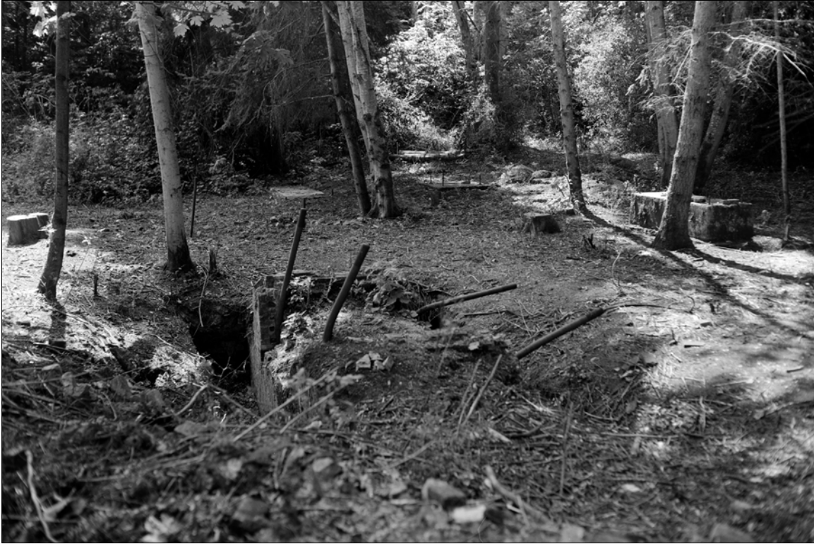
Figure 7. Overview, 1983, of the Engine House and Electric Power House areas (Britton and Britton 1983: Photograph 2).
