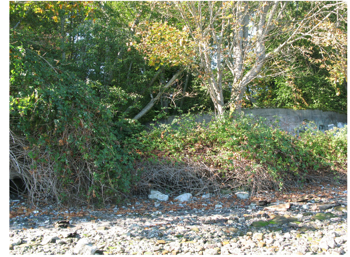
P-4 VIEW WEST AT REMEDIAL EXCAVATION AREA, SHOWING CONCRETE TANK.
