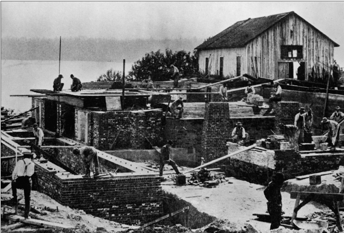
Figure 10. Overview of construction of the open hearth furnaces in the Steel Production Building, ca. 1909 (Britton and Britton 1983: Photograph 28).
