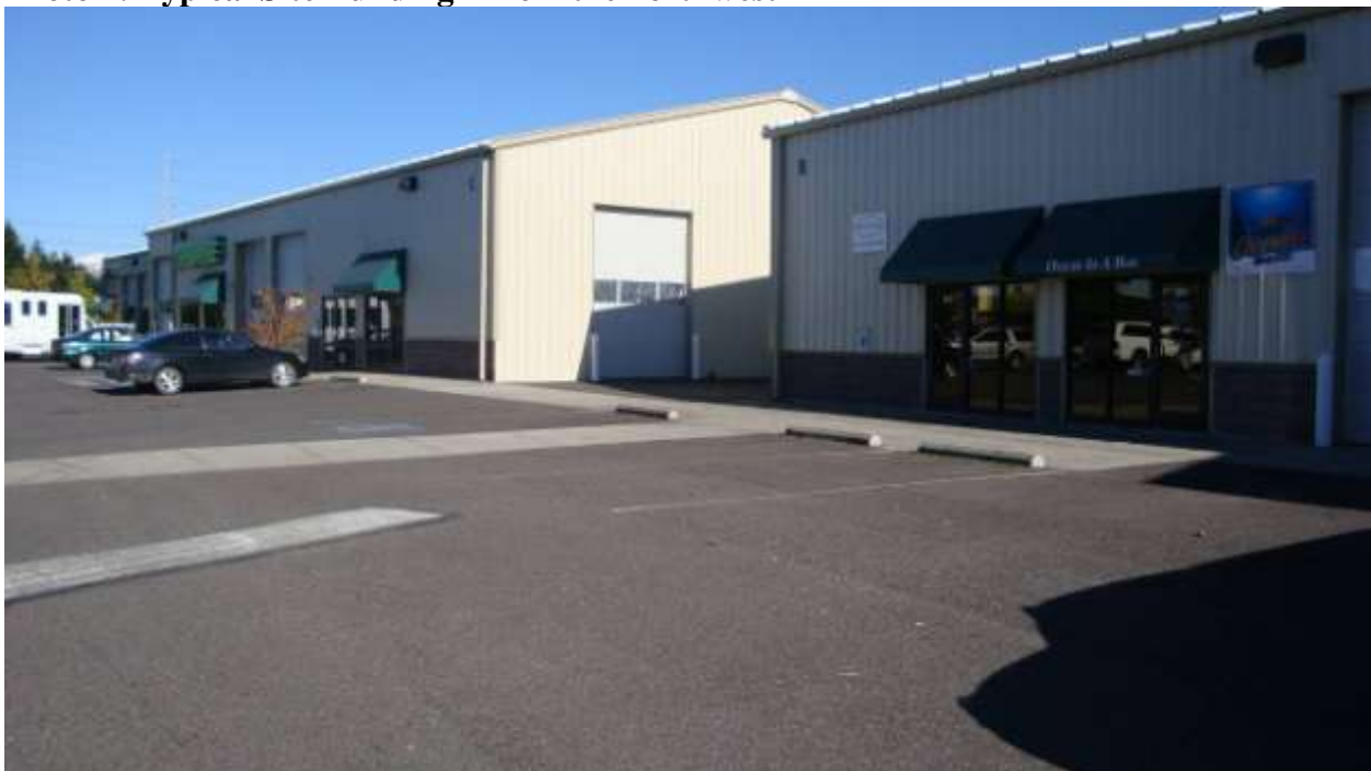
Photo 2: Typical Site Building – from the northwest
