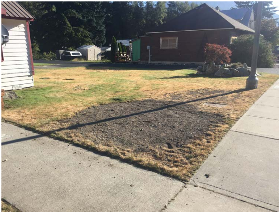
Photograph 2: Backfill following removal of the air sparge system vault.
