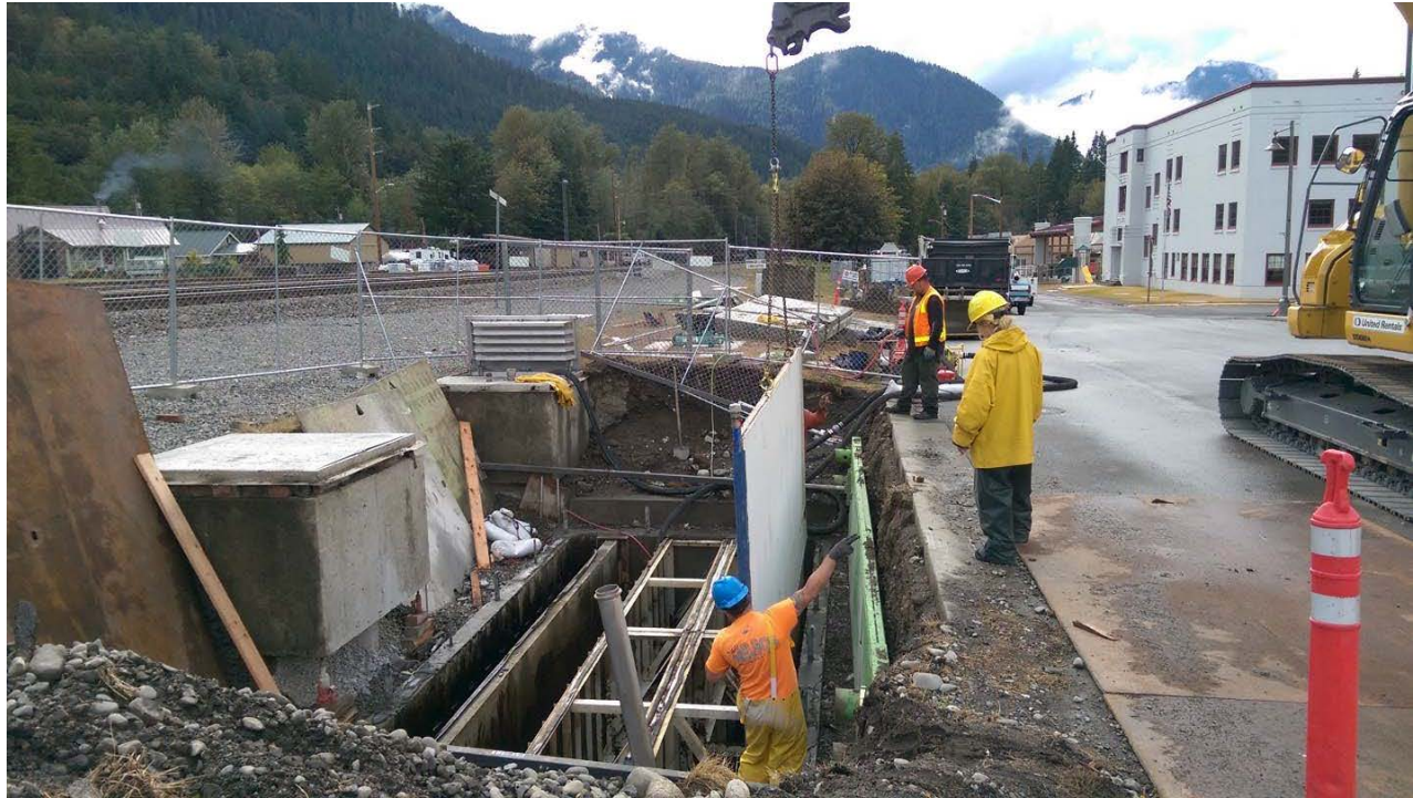
Photograph 17: Installation of water barriers.
