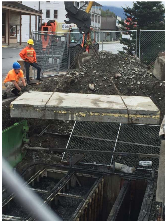
Photograph 28: Reinstallation of vault lid.
