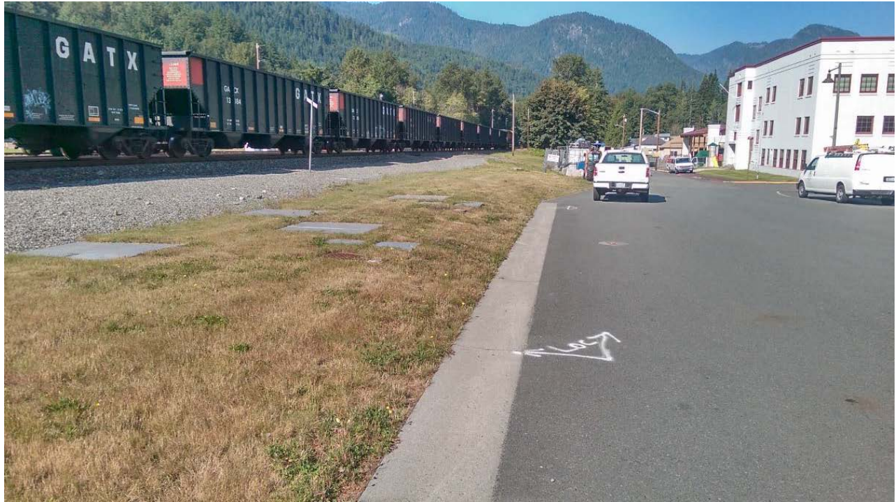
Photograph 1: Preconstruction Site conditions.
