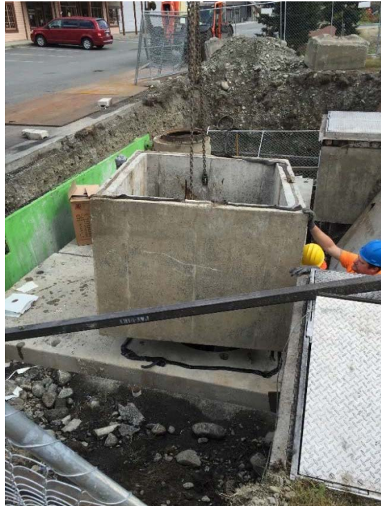
Photograph 31: Replacement of access riser.
