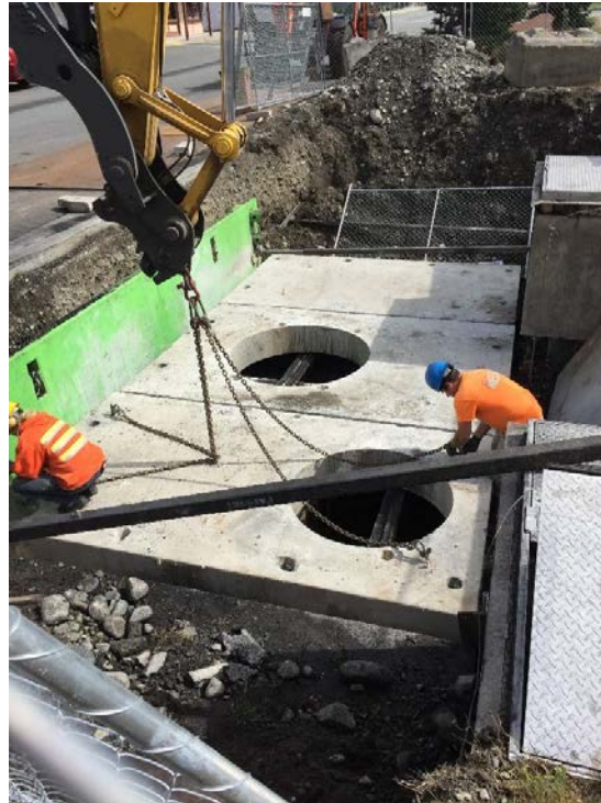
Photograph 29: Reinstallation of vault lids.
