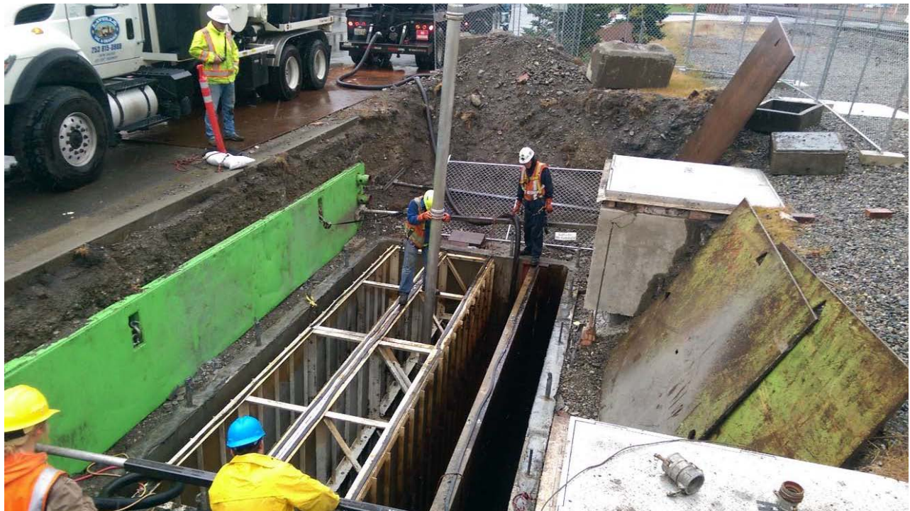
Photograph 22: Removal of saturated material with vector.
