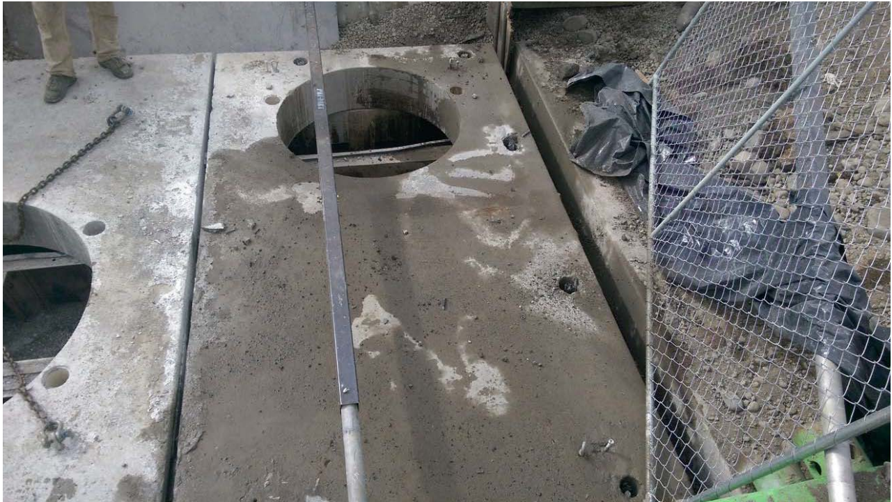
Photograph 9: Exposed vault lid.
