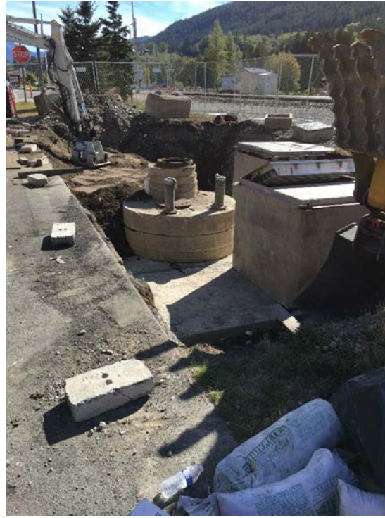
Photograph 33: Backfill and compaction.
