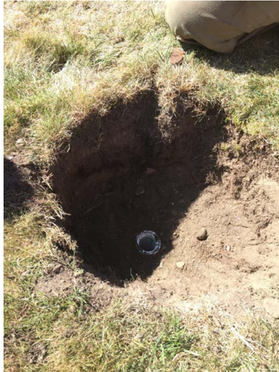
Photograph 3: Exposed air sparge well prior to decommissioning.
