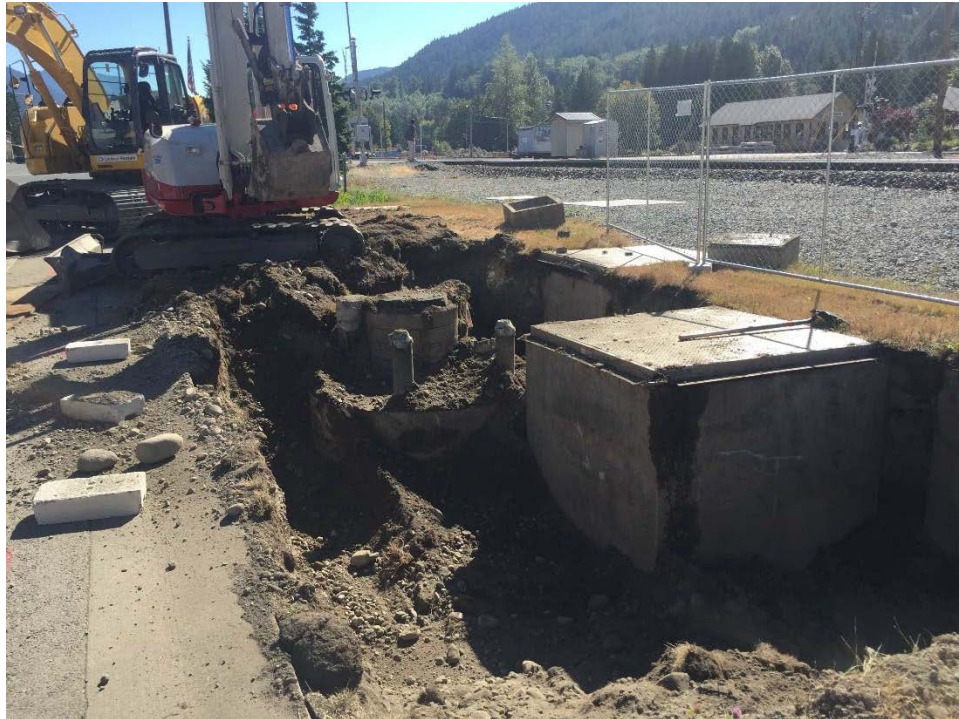
Photograph 3: Excavation to vault top.
