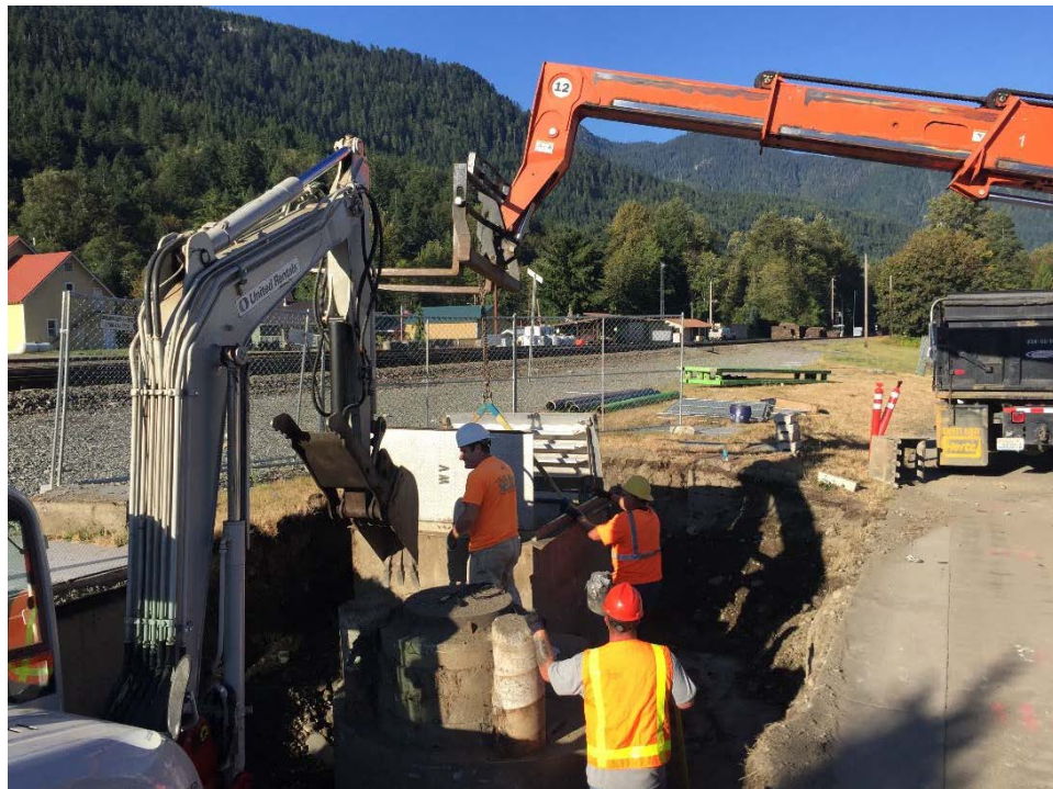
Photograph 4: Removal of Vault Access Hatch
