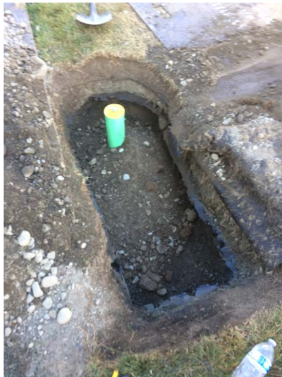
Photograph 24: Sewer cleanout installed southwest of the teacheage.
