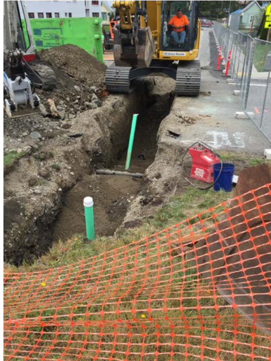
Photograph 21: Sewer installation activities at Railroad Avenue and Sixth Street.
