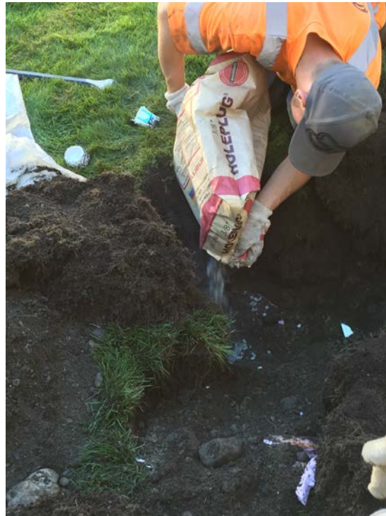
Photograph 5: Holt Drilling decommissioning air sparge well with bentonite chips.
