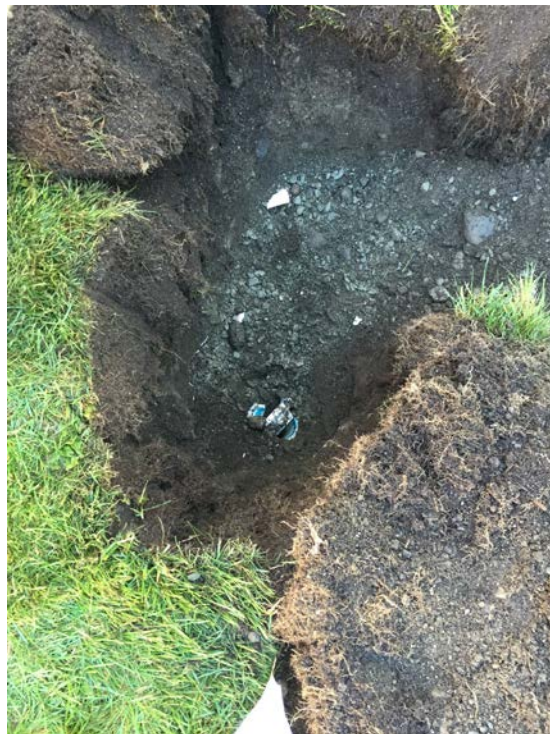
Photograph 4: Exposed air sparge well prior to decommissioning.
