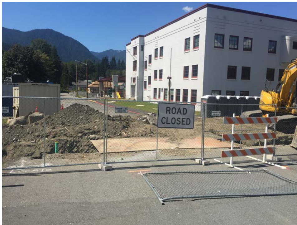
Photograph 18: Traffic control and fencing, looking west across Railroad Avenue.
