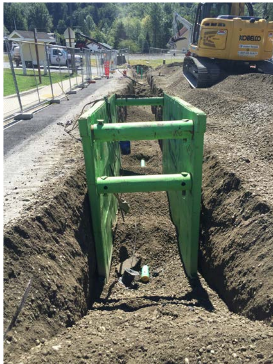
Photograph 22: Backfill and compaction activities south of Railroad Avenue.
