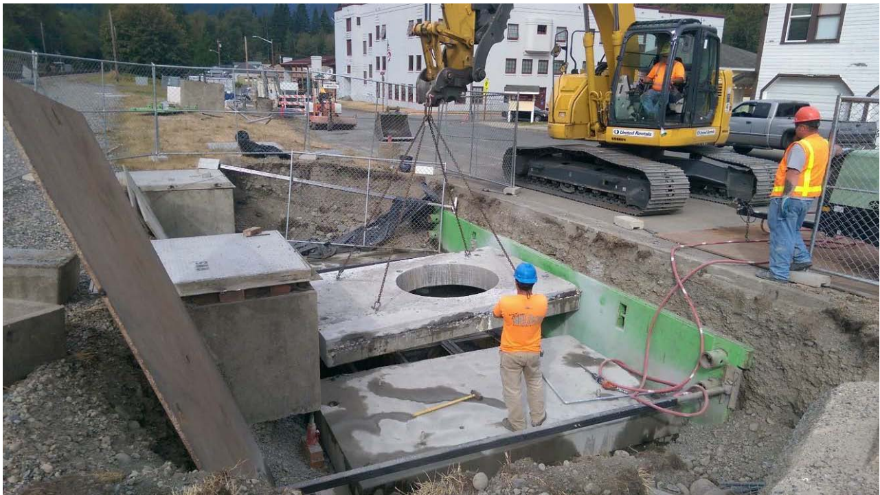
Photograph 10: Lifting concrete vault lid.
