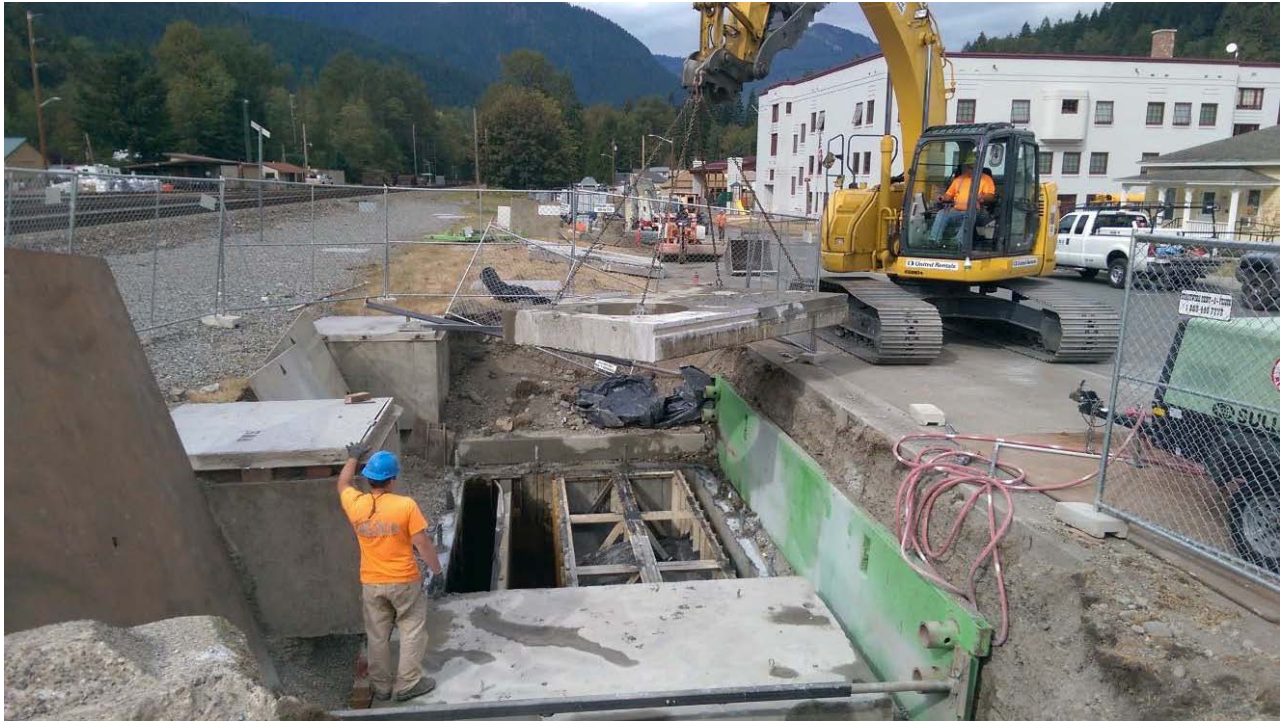
Photograph 11: Removal of concrete vault lid.
