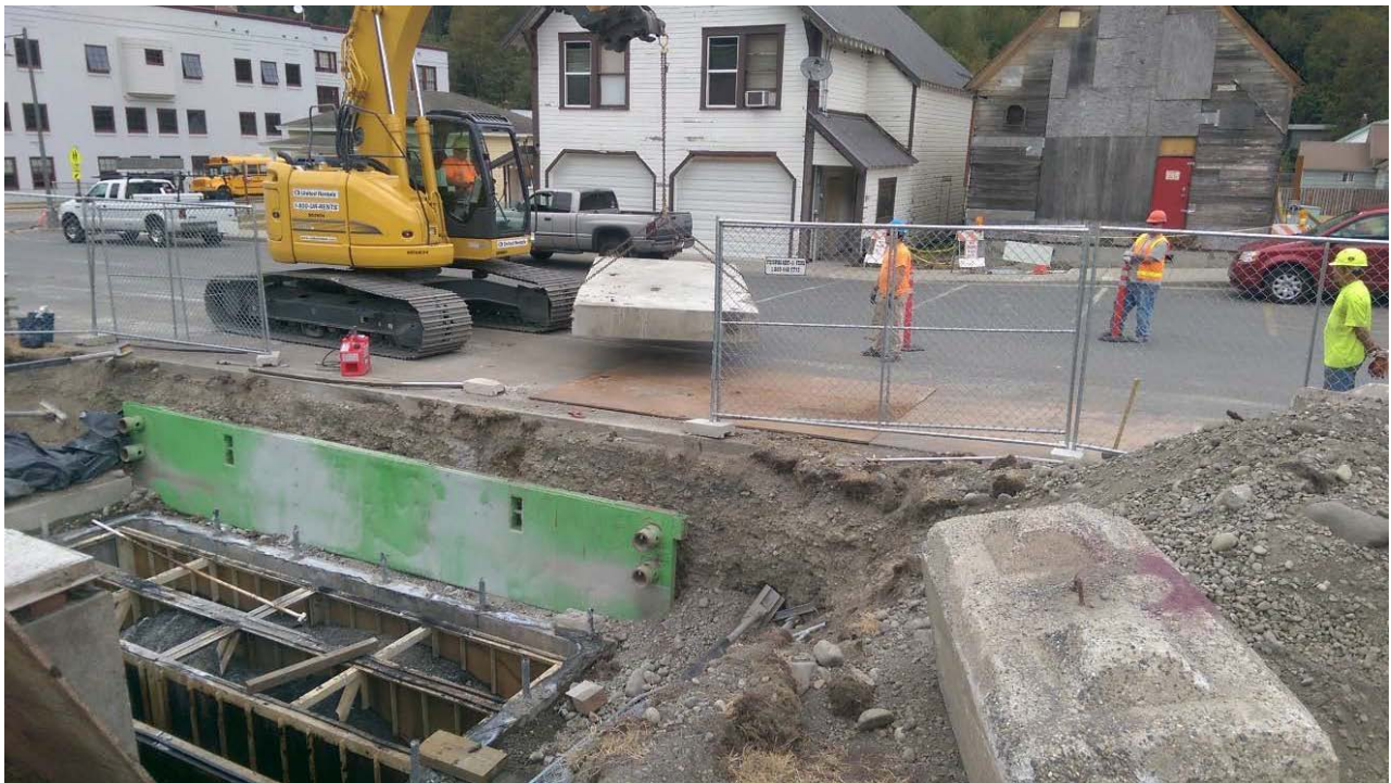
Photograph 14: Removal of final concrete lid.
