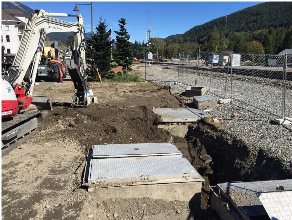
Photograph 34: Backfill and compaction.
