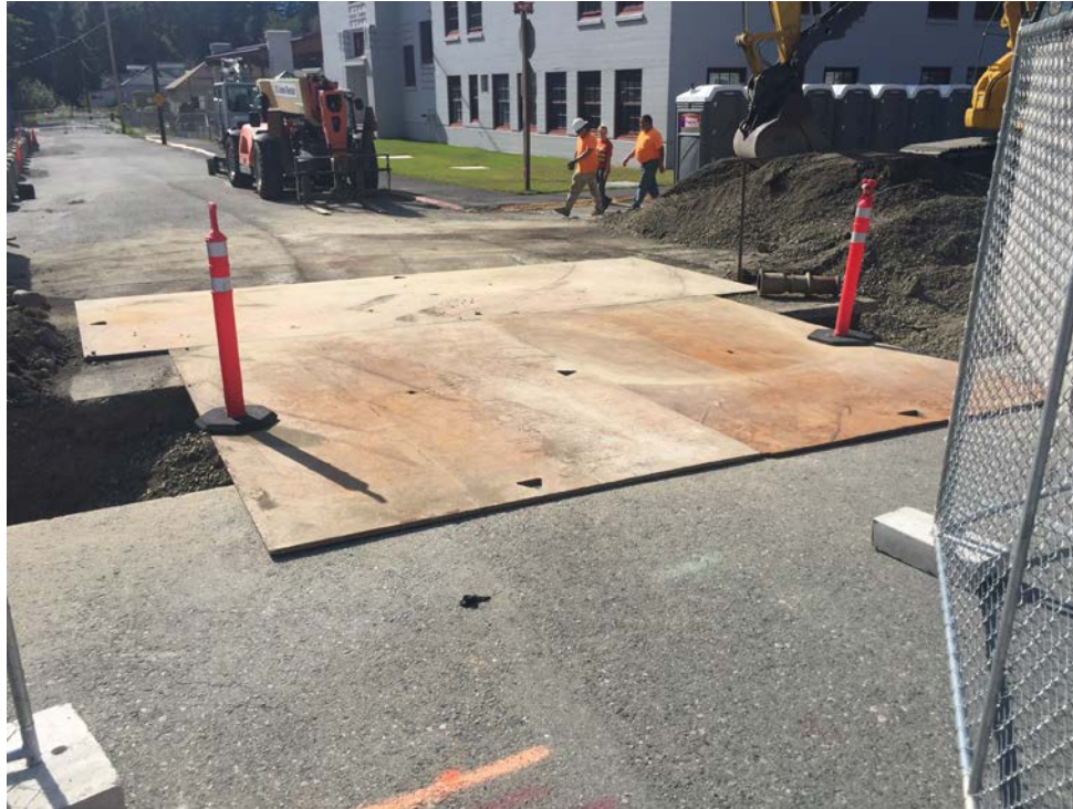
Photograph 19: Steel plates placed across trench for emergency access at Railroad Avenue.
