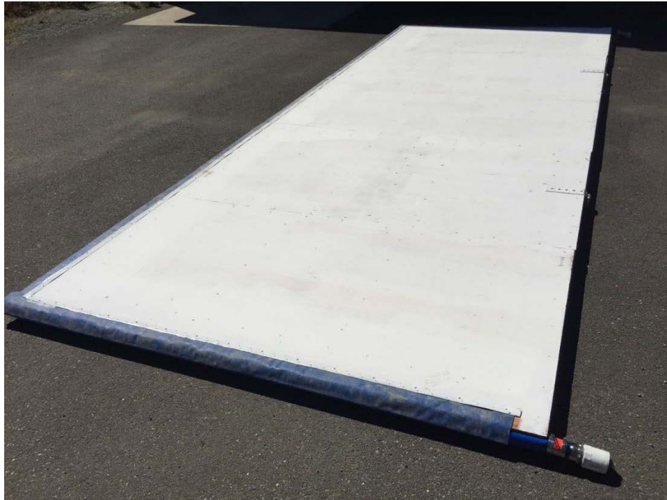
Photograph 19: Water barrier detail.
