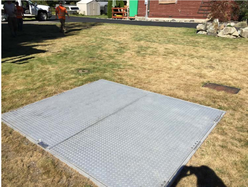
Photograph 1: Air sparge system vault prior to decommissioning activities.
