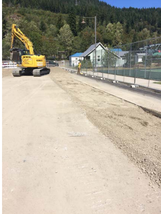
Photograph 25: Sixth Street following backfill and compaction, looking north.
