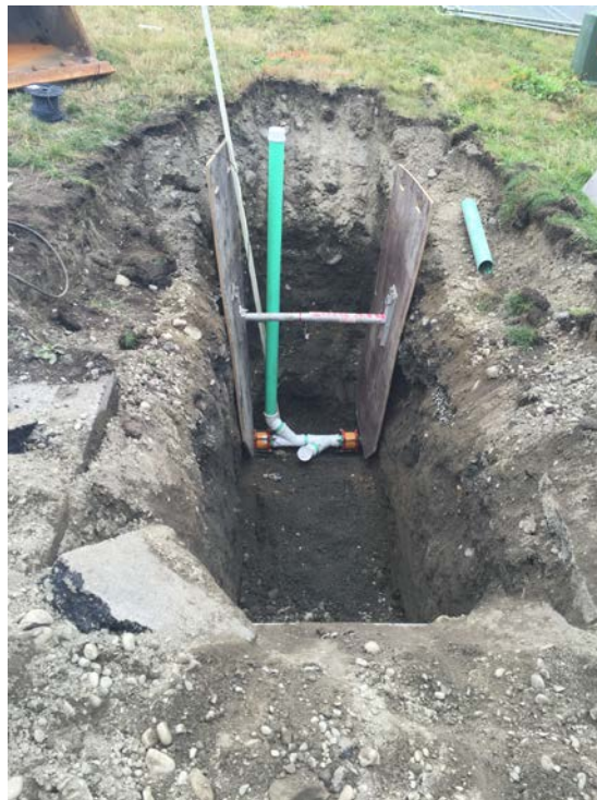
Photograph 20: Installed sewer cleanout south of Railroad Avenue, looking south.
