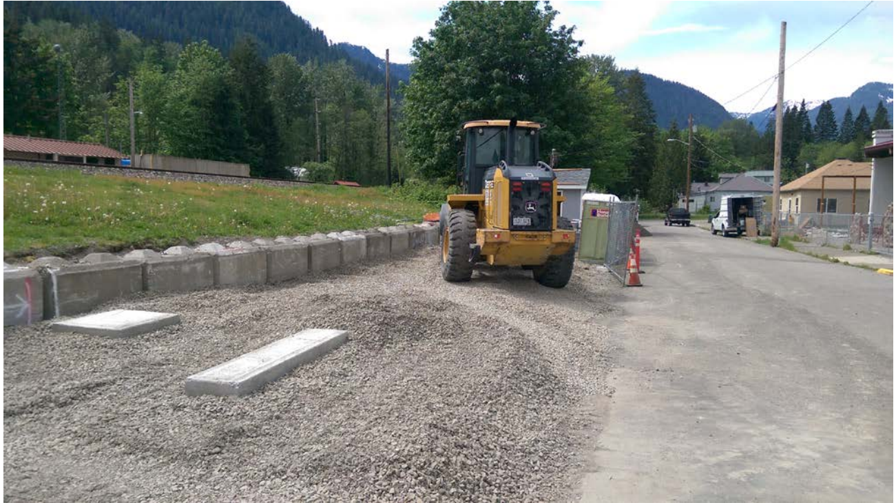
Photograph 7: Pad for the hot water flushing (HWF) treatment compound, looking west.
