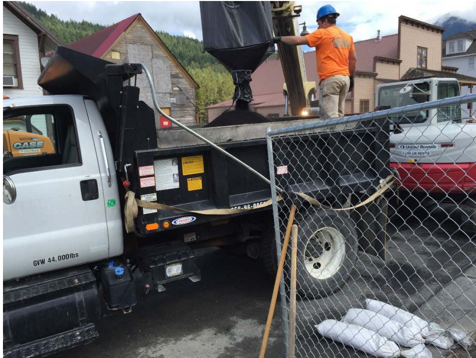
Photograph 23: Mixing GAC/pea gravel materials.
