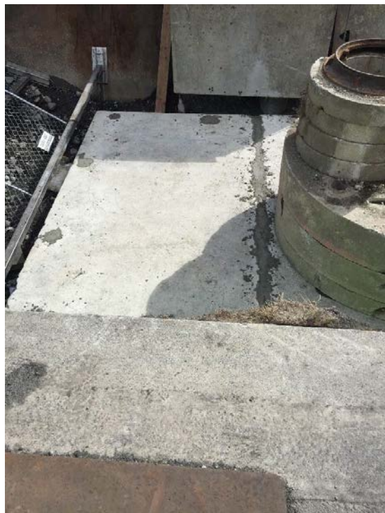
Photograph 32: Grouting rebar dowel holes and vault seam.
