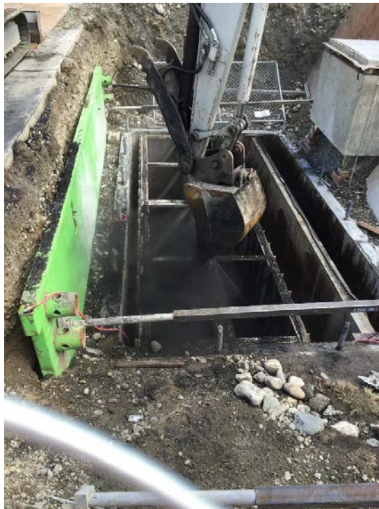
Photograph 26: Placement of GAC/pea gravel materials.
