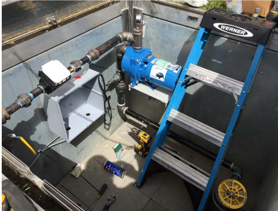
Photograph 17: Groundwater recovery sump at the School Site following pump installation.
