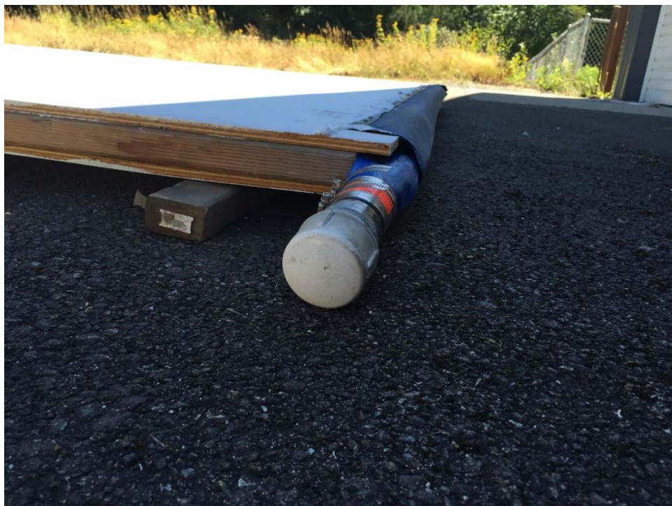
Photograph 20: Water barrier detail.
