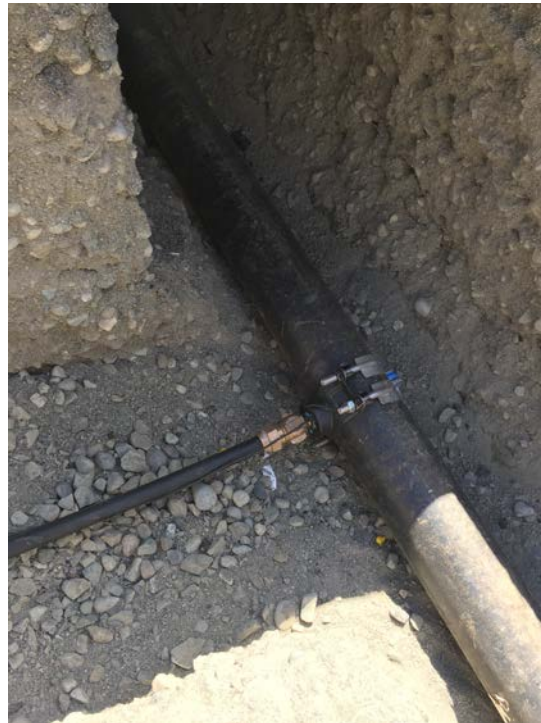
Photograph 6: Installation of water service laterals in Sixth Street.
