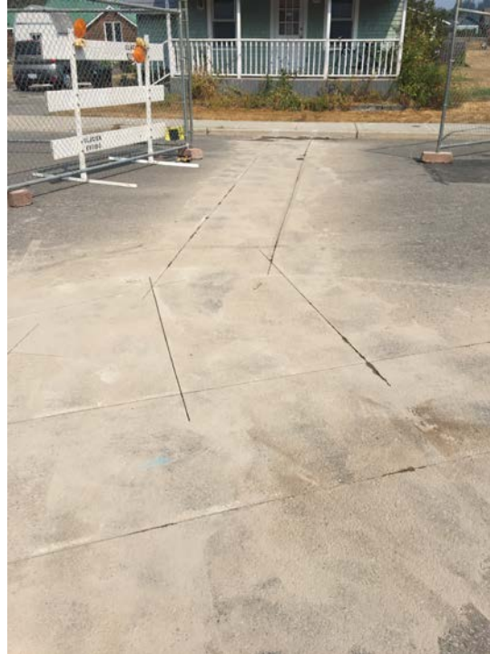
Photograph 1: Traffic control, fencing, and asphalt saw-cutting, looking east.
