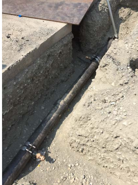
Photograph 5: Installation of lateral connection fittings on new water main.
