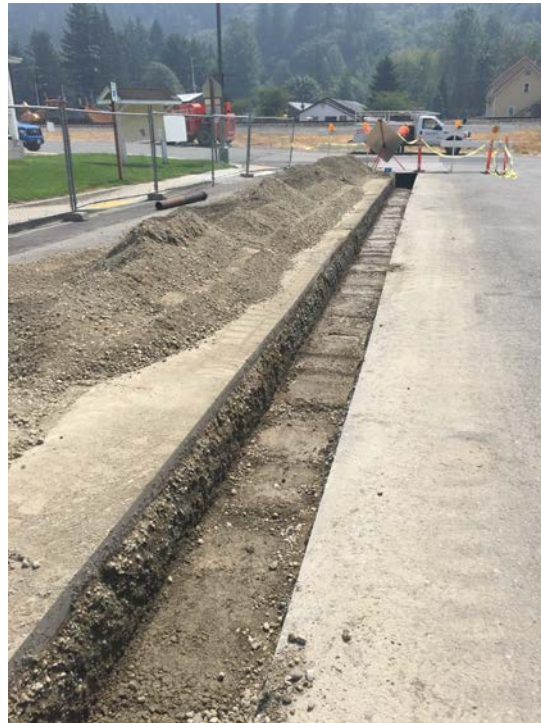
Photograph 4: Trench backfill and compaction activities at southern end of Sixth Street.
