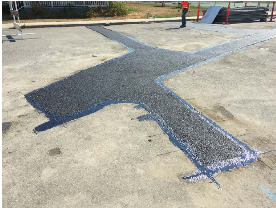
Photograph 8: New asphalt pavement and sealant, looking east.
