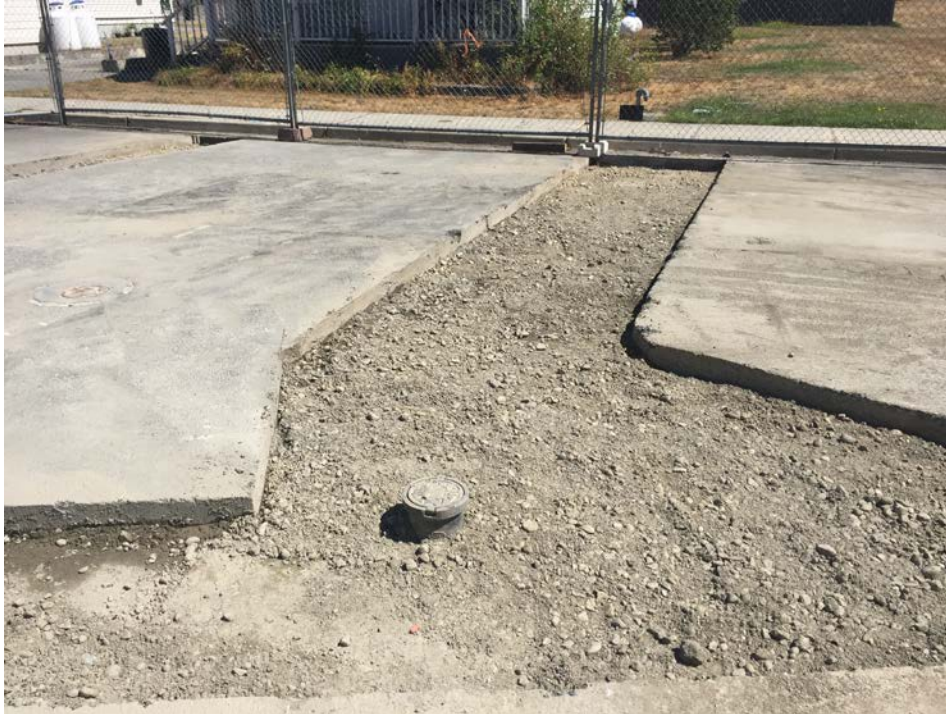
Photograph 7: Compacted backfill placement, looking east.
