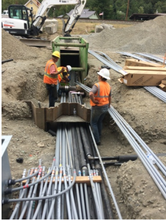
Description: Glacier and Town of Skykomish installing water service pipe on Railroad Avenue.
