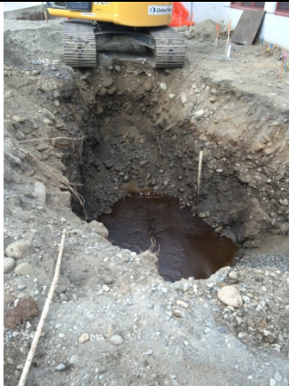
Description: Glacier excavating recovery trench northeast of school.
