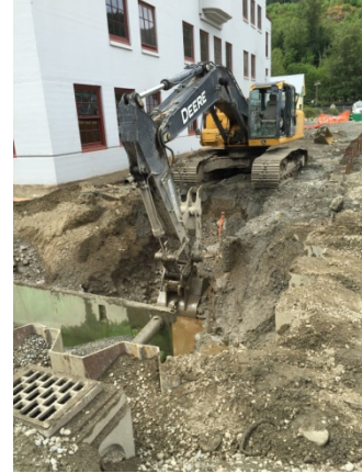
Description: Glacier excavating recovery trench east of school.
