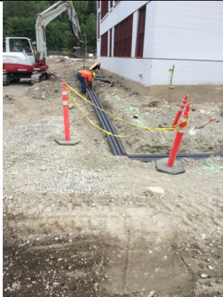
Description: Glacier installs HWF pipe insulation.
