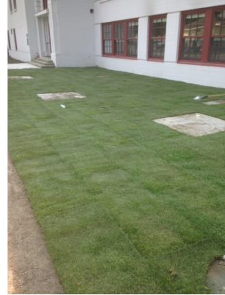
Description: Glacier placing sod along north and east side of school.
