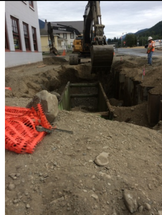
Description: Glacier excavating recovery trench southeast of school.
