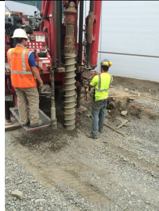
Description: Holt installs recovery wells.
