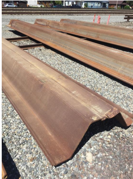
Photograph 1: Sheet piles sitting in rail yard prior to installation, facing north.
