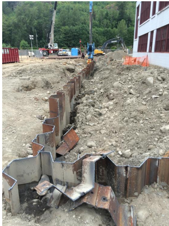
Photograph 12: Blue Iron installing sheet piles northwest of school, facing north.
