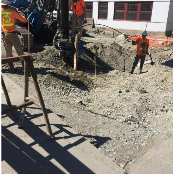
Photograph 15: Malcolm Drilling conducting permeation grouting, facing southwest.
