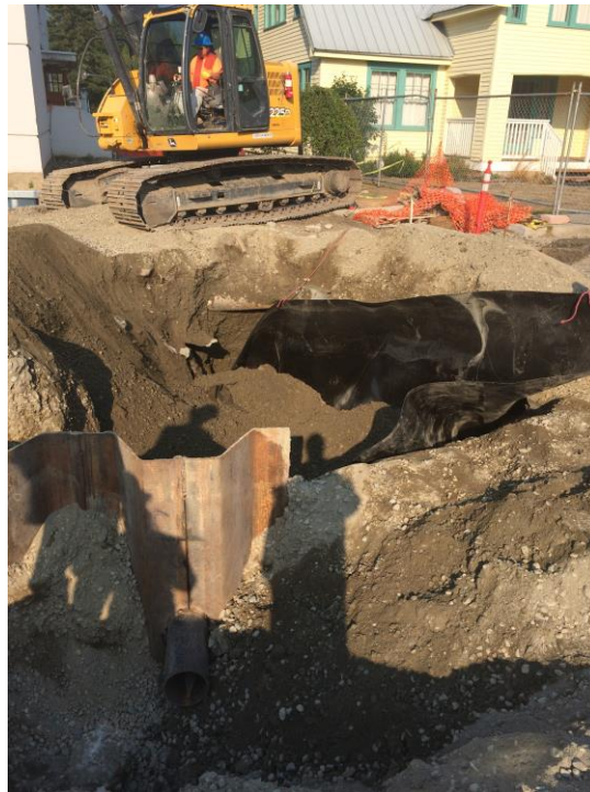
Photograph 14: Geomembrane liner near northeastern corner of Site, facing west.
