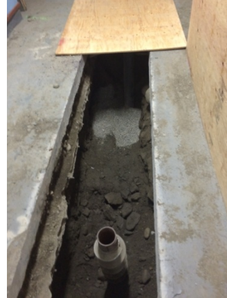
Description: Installation of injection well INJ-12 in hallway.
