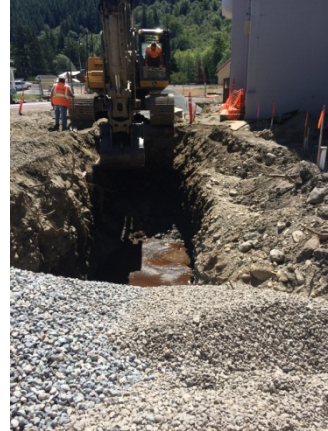
Description: Glacier installs recovery trench east of school.
