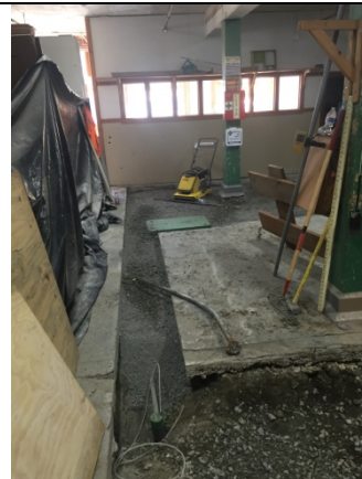
Description: Holt installs recovery wells.
