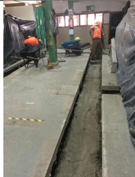
Description: Glacier demolishing concrete for trench inside school shop.
