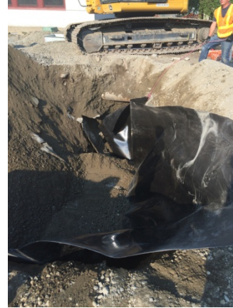
Description: Glacier installing liner for Change Order 12.
