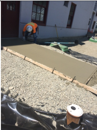
Description: Salinas Concrete placing concrete sidewalk east of school.
