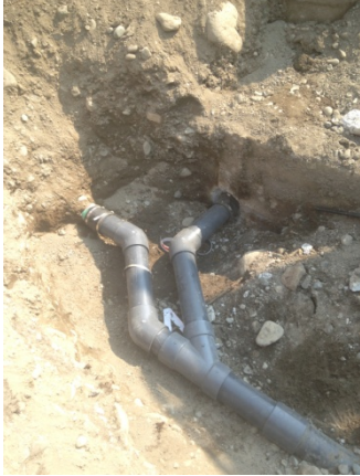
Description: Glacier removing distribution box and temporary sewer connection.
