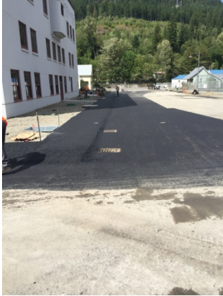
Description: Lakeridge Paving placing asphalt along 6 th Avenue.
