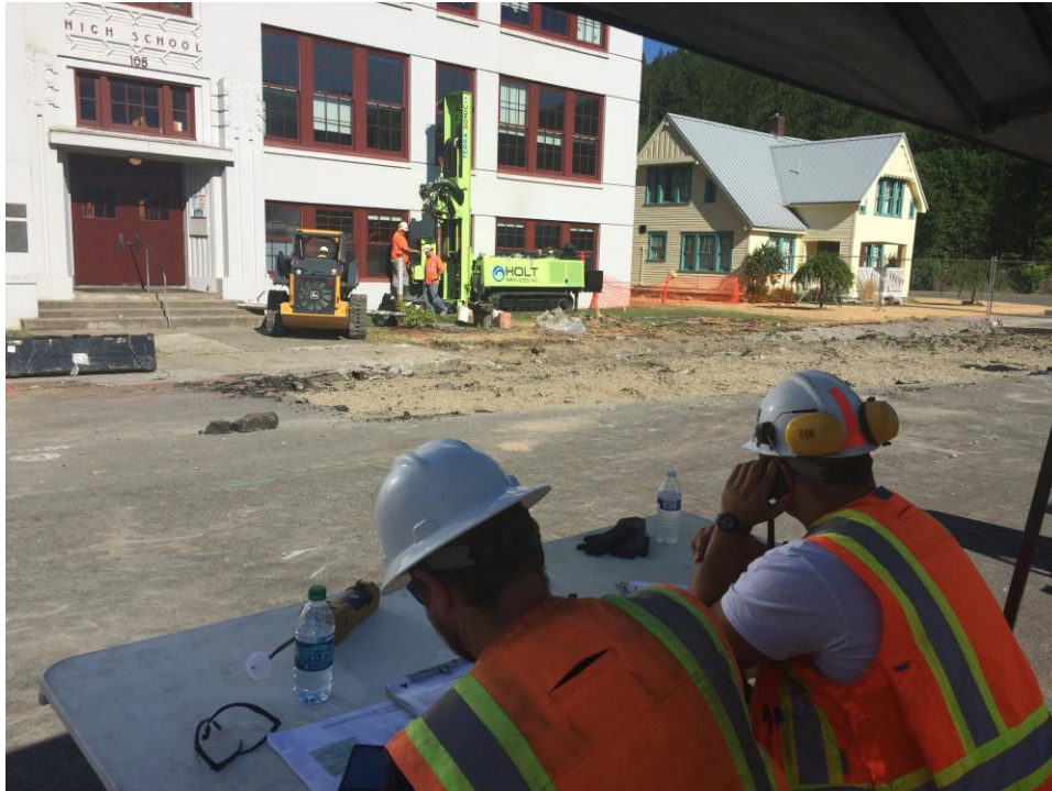
Photograph 3: Holt Services installing a hot water flushing system well, facing west.
