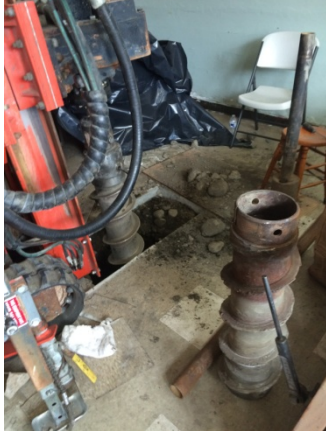
Description: Holt installing soil vapor extraction well SVE-1 in cafeteria.
