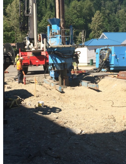
Description: Blue Iron installing sheet pile east of school.
