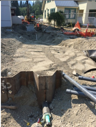
Description: Glacier and Town of Skykomish installing water service pipe on Railroad Avenue.
