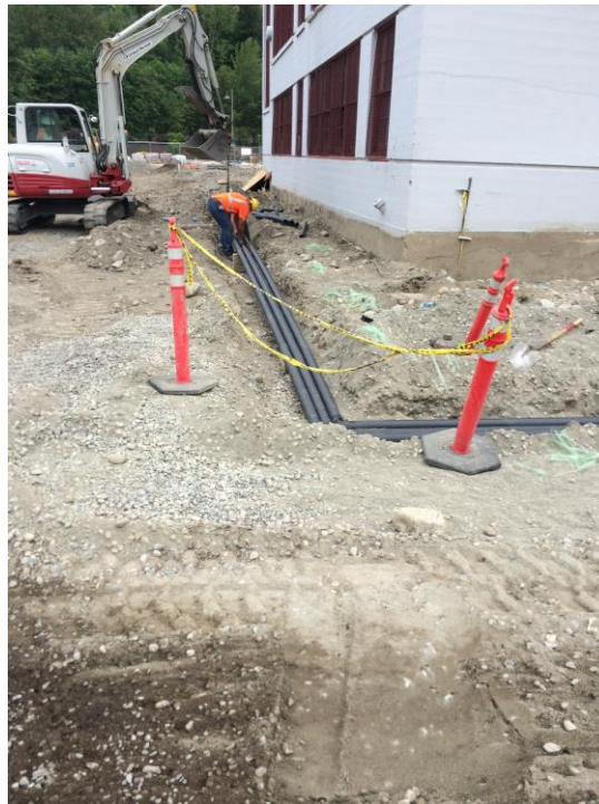
Photograph 18: Glacier Environmental installing hot water flushing system pipe insulation, facing north.
