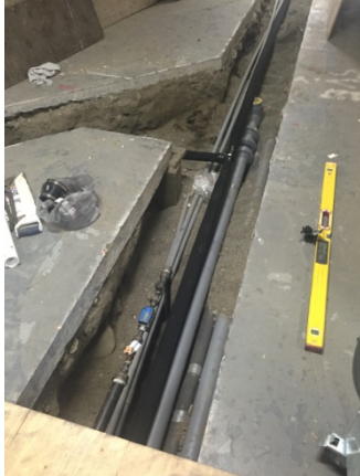
Description: Glacier installs HWF controls inside the basement of the school.
