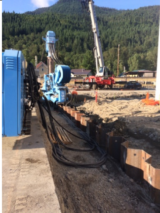
Description: Blue Iron installing sheet pile along 6 th Avenue.
