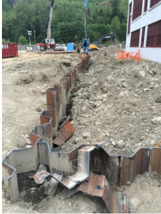
Description: Trimming sheet pile to design grade west of school.
