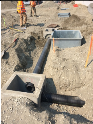
Description: Glacier installs storm drain system east of the school.
