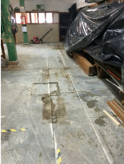
Description: Saw cuts in shop for interior trenching.
