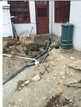
Description: Glacier installing FDC along Railroad Avenue.
