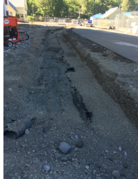
Description: Trenching for sheet pile installation.
