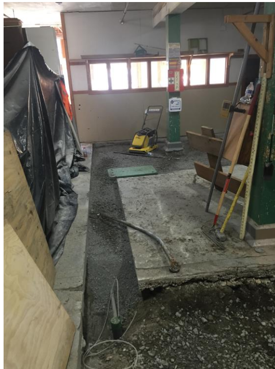
Photograph 10: School interior showing backfill and compaction, facing south.
