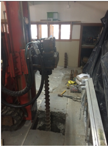
Description: Holt drilling installing system groundwater monitoring wells inside school shop.
