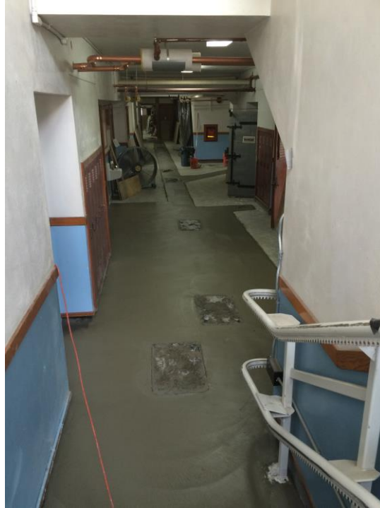
Photograph 9: School interior showing recently poured concrete, facing south.
