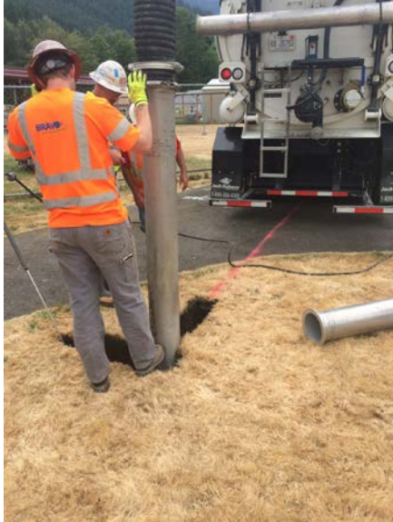
Description: Bravo Environmental locating MSE wall adjacent to sheet pile intersection.
