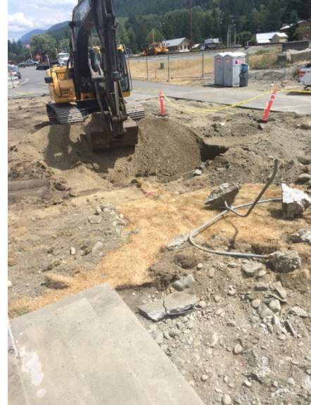
Description: Glacier excavator removing overburden soil from supplemental excavation area.
