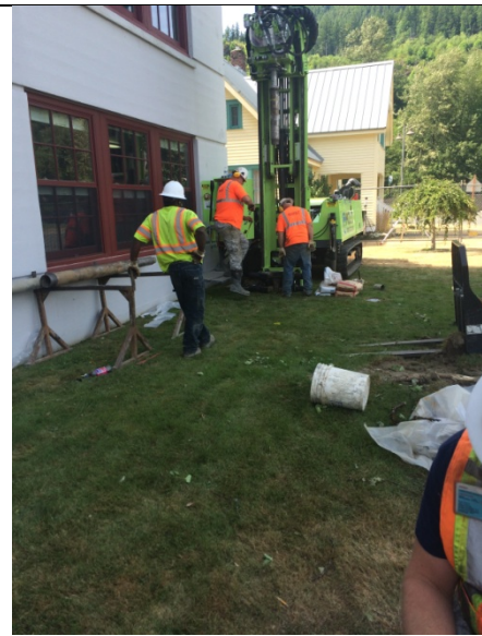
Description: Holt drilling installing system injections wells east of school.
