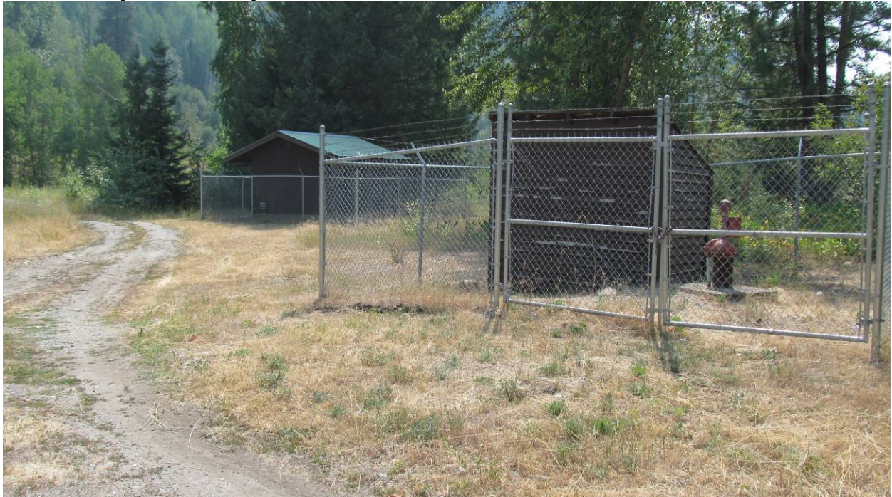
Photo 2: City Well Facility – from the northeast
