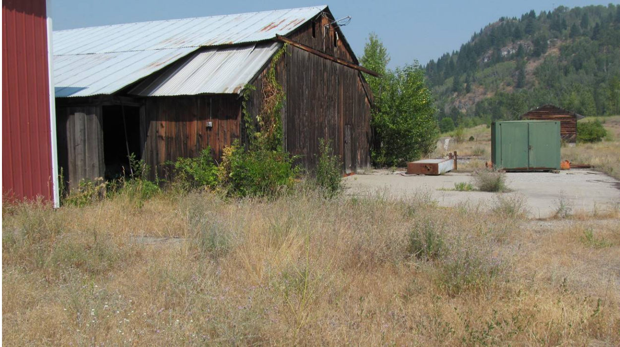
Photo 3: Former Lumberyard Structures – from the south
