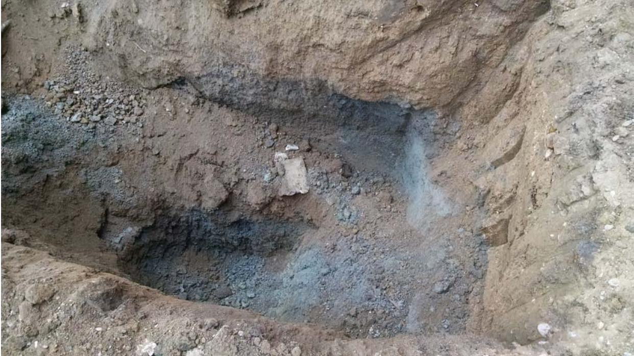
**Figure 4.** View of the excavation and soil around the former UST. Blue colored soil had odors indicative of release.
