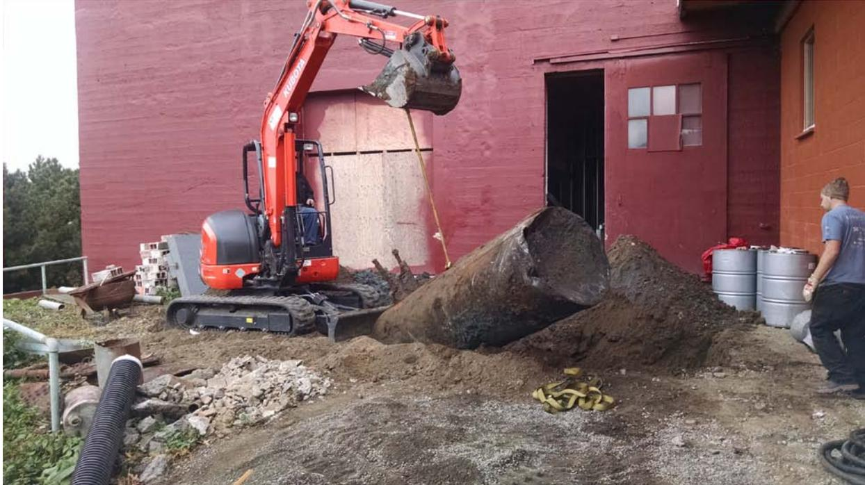
**Figure 3.** View of the UST removal
