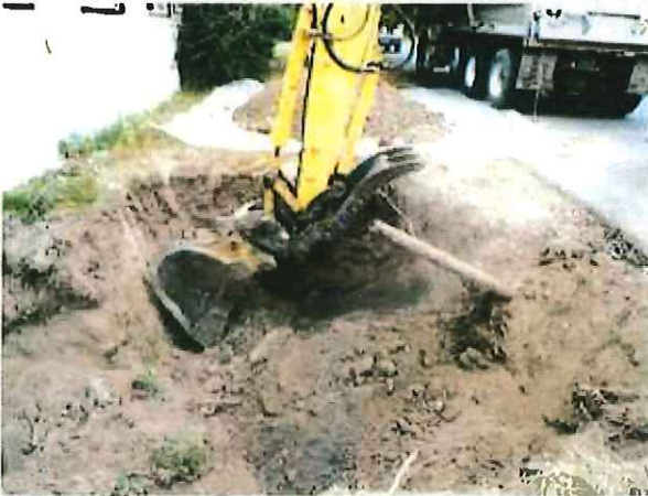
Photograph 15. UST #3 Excavating Petroleum-Impacted Soils
