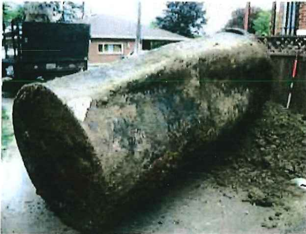
Photograph 1. Removed UST #1
