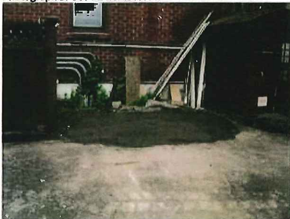
Photograph 5. Backfilled UST #1 Excavation
