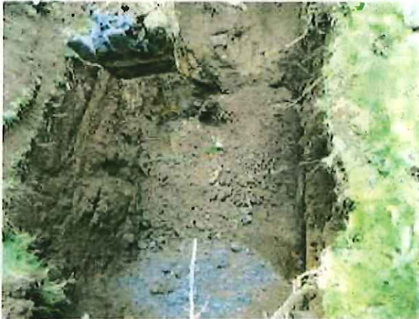
Photograph 9. UST #2 Removal Pit
