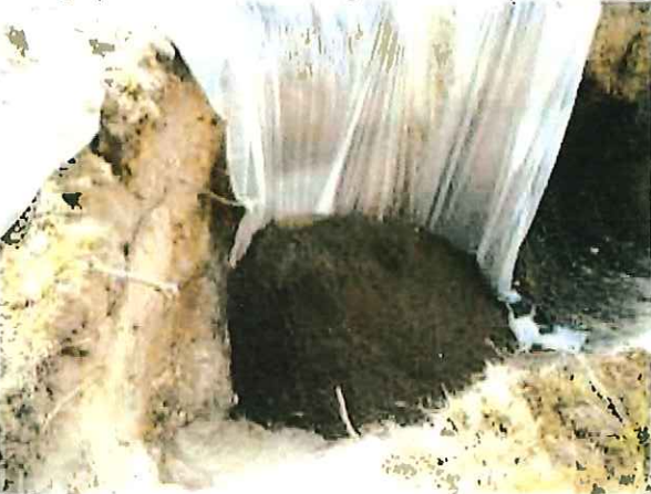
Photograph 17. Backfilling UST #3 Excavation
