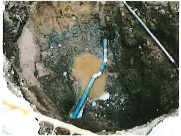
Photograph 4. UST #1 Final Excavation
