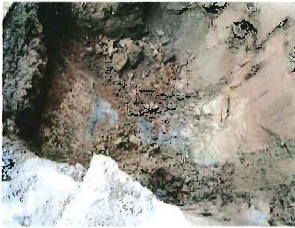
Photograph 3. UST #1 Removal Pit
