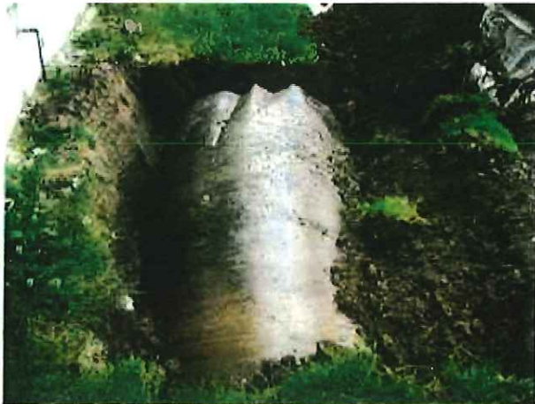
Photograph 13. Removing UST #3
