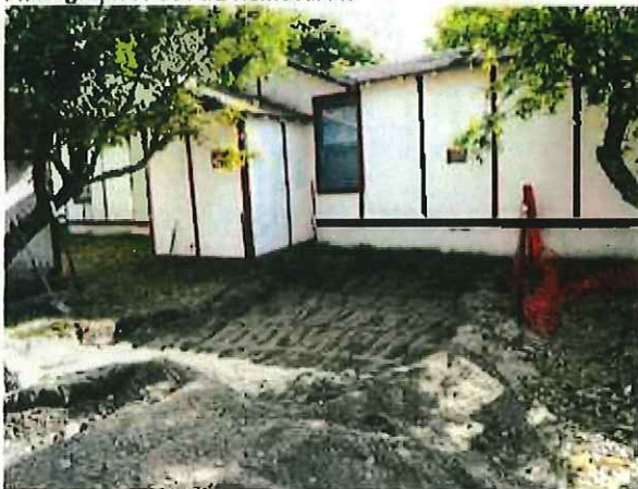
Photograph 11. Partially Backfilled UST #2 Excavation
