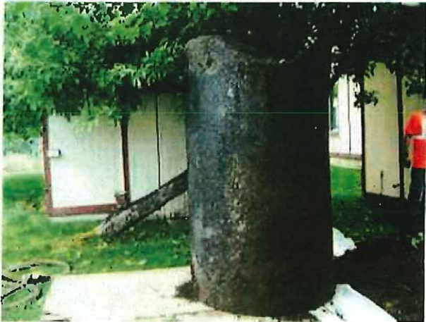
Photograph 7. Removed UST #2
