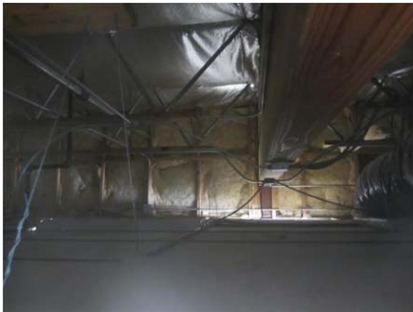
Photo 1. View to west of general view of wall separating Amy's and Hallmark suites. Above drop ceiling looking west. Note wall penetration by piping and conduits.
