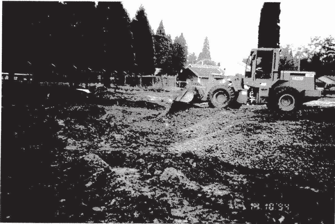
Photograph #10: Spreading pit run into shallow excavation. Photograph taken looking southwest.
