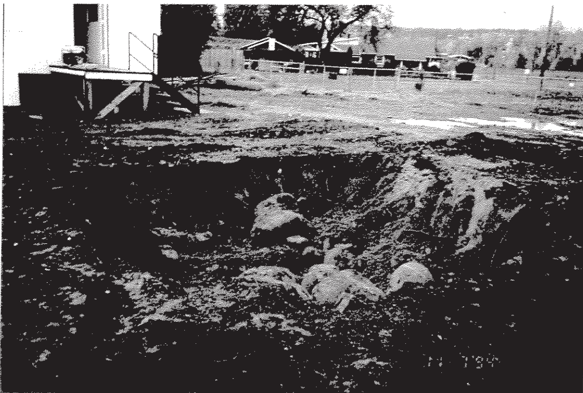
Photograph #5: Warehouse excavation nearest existing office building. Note silt in sidewalls. Boulders were encountered at bottom of excavation. Photograph taken looking west.
