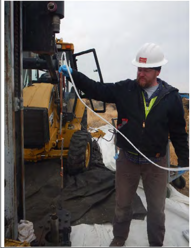
Groundwater sampling pump with weights at PP-2
