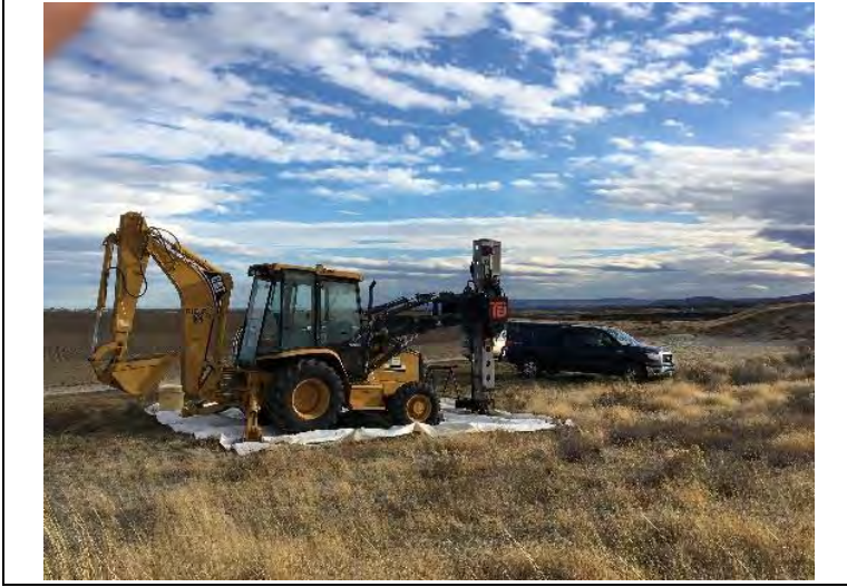
PP-5 View toward Southeast
