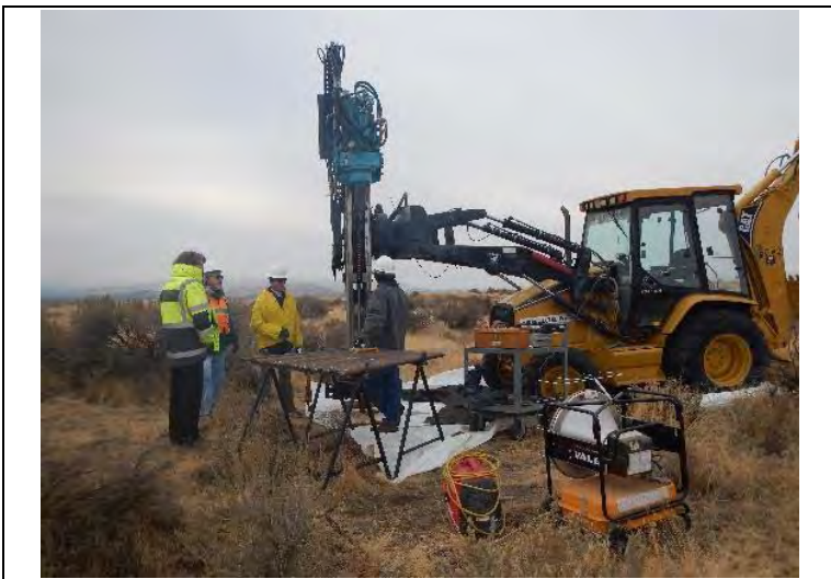
PP-2 Rig and Drill Pipe View toward South
