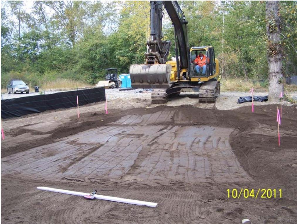
Photo 22. Grading and compacting low-permeable soil for wetland creation.
