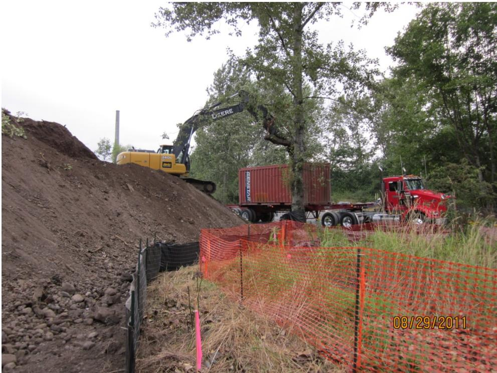
Photo 8. Loading container for transport to Roosevelt landfill.
