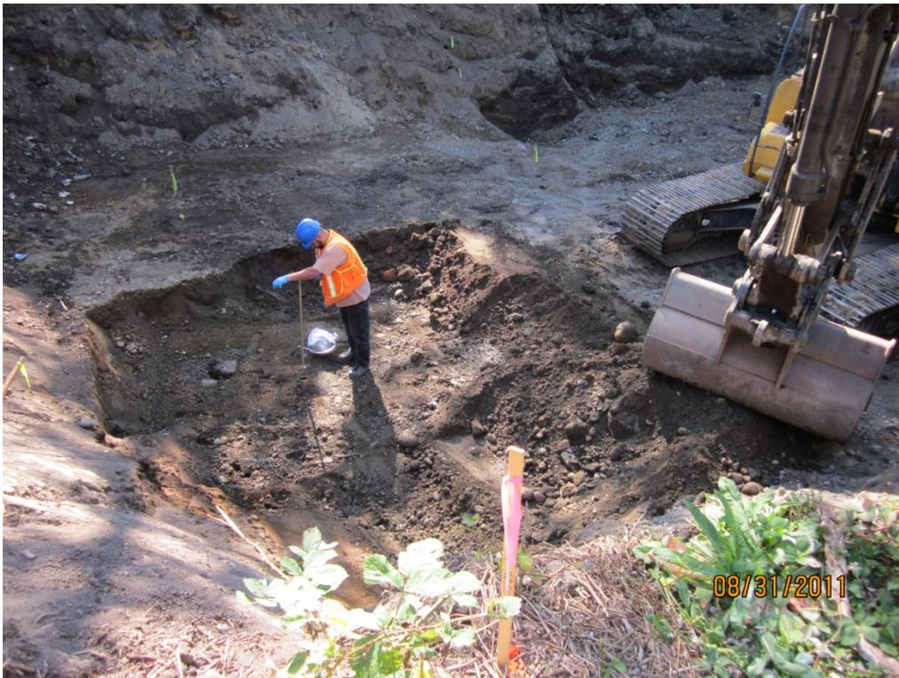
Photo 10. Confirmation sampling in Excavation Area 1.
