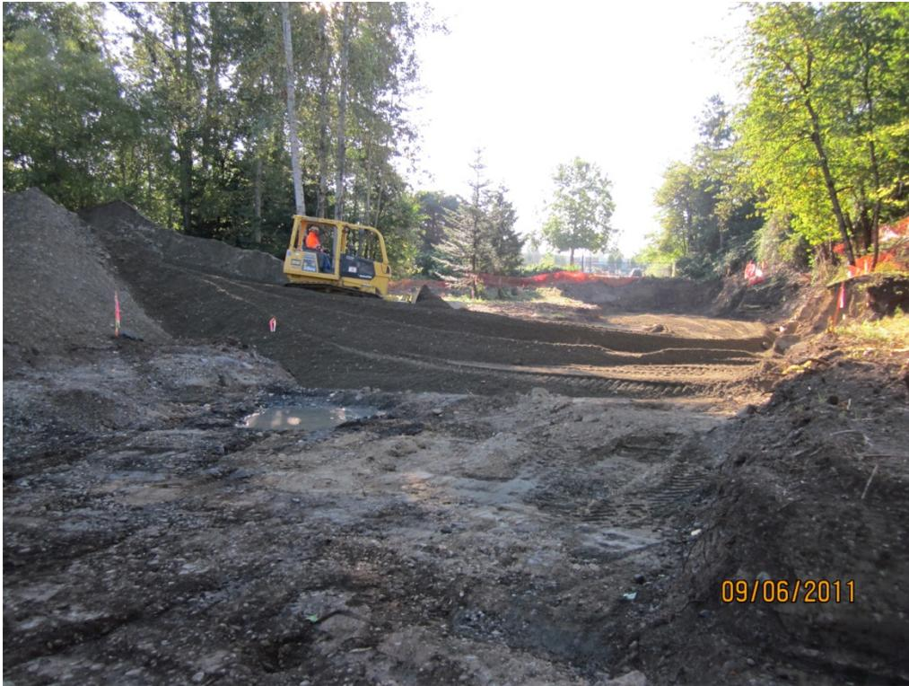
Photo 13. Filling excavation Area 1 with clean sand and gravel.
