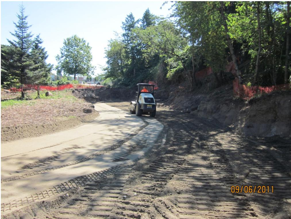
Photo 14. Compacting/rolling fill in Area 1.
