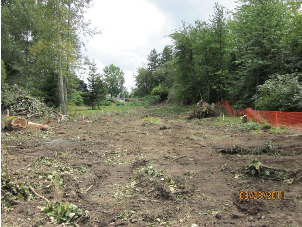
Photo 1. Clearing and grubbing Site.
