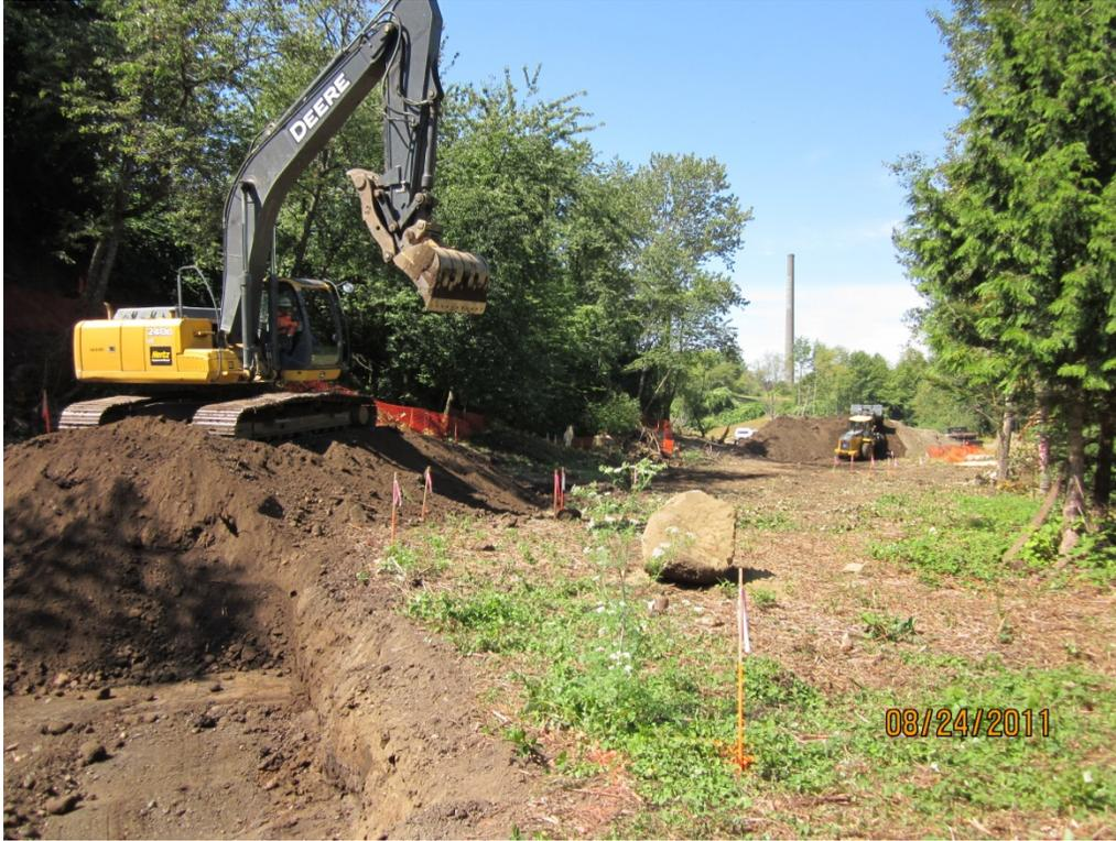
Photo 3. Excavation of Area 1, loading, and stockpiling within boundary of Site.
