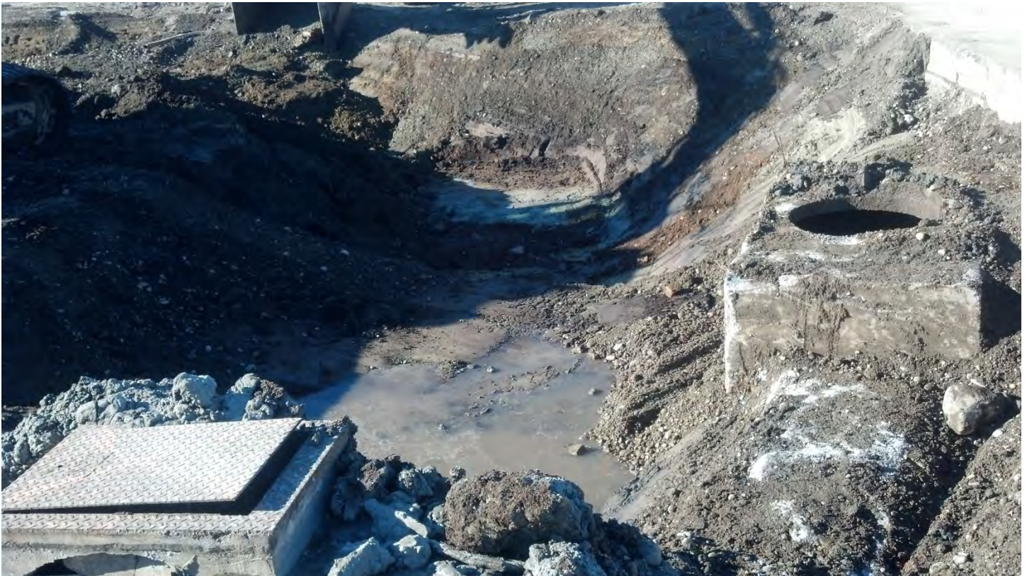
Photo 15 –Former duct bank (subsequently removed) south edge of Main Street.
