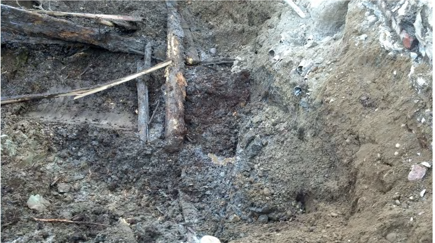
Photo 11 –Wooden cribbing uncovered and removed during excavation west of SR-527
