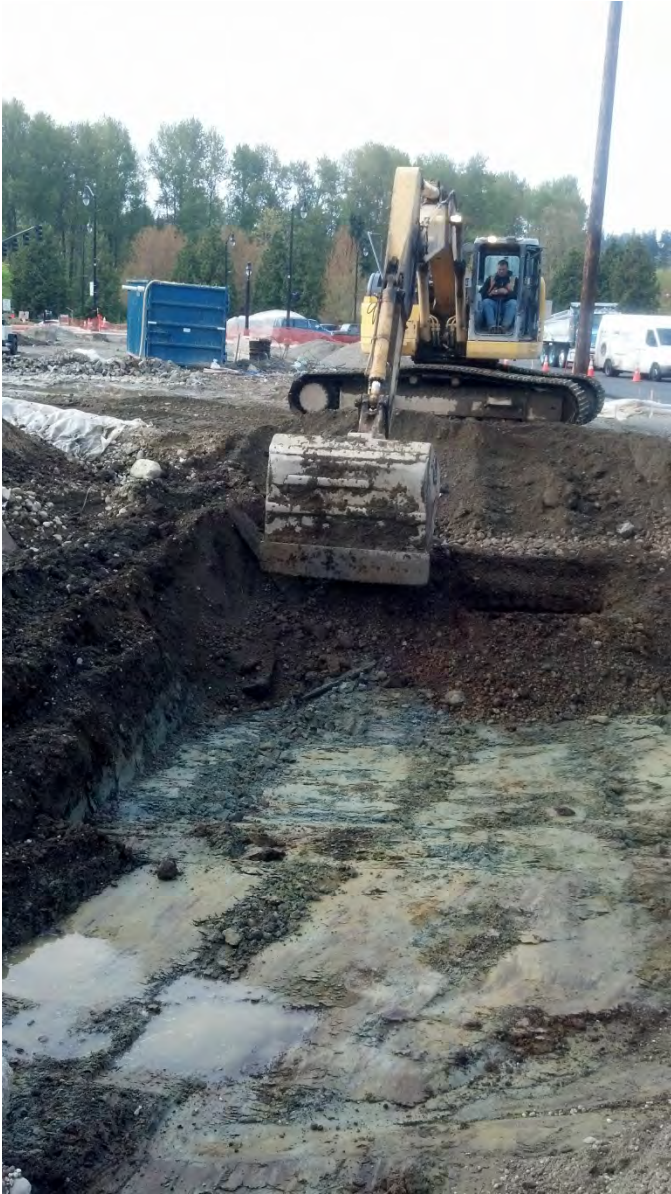
Photo 16 – Excavation along east side of SR-527, showing native soils
