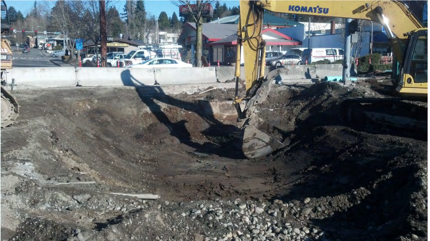
Photo 14 –Excavation along east side of SR-527 and Main Street
