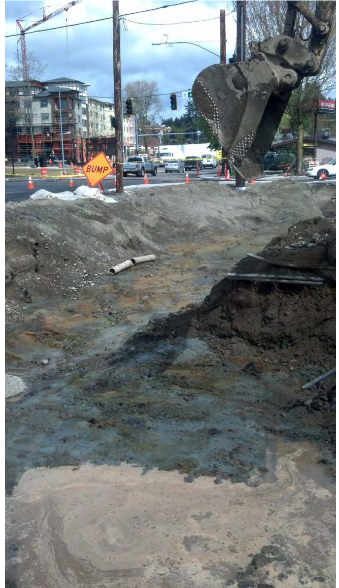
Photo 17 – Excavation along east side of SR-527, showing native soils
