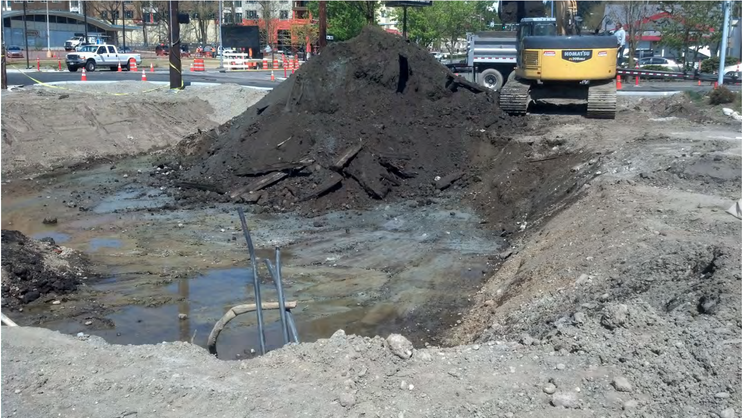
Photo 20 – Loading stockpiled soils excavated at Triangle Park vicinity
