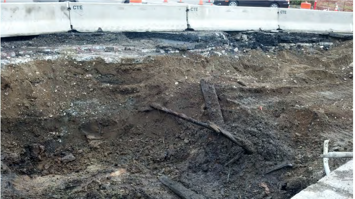
Photo 10 –Excavation along west side to SR-527, October 2013
