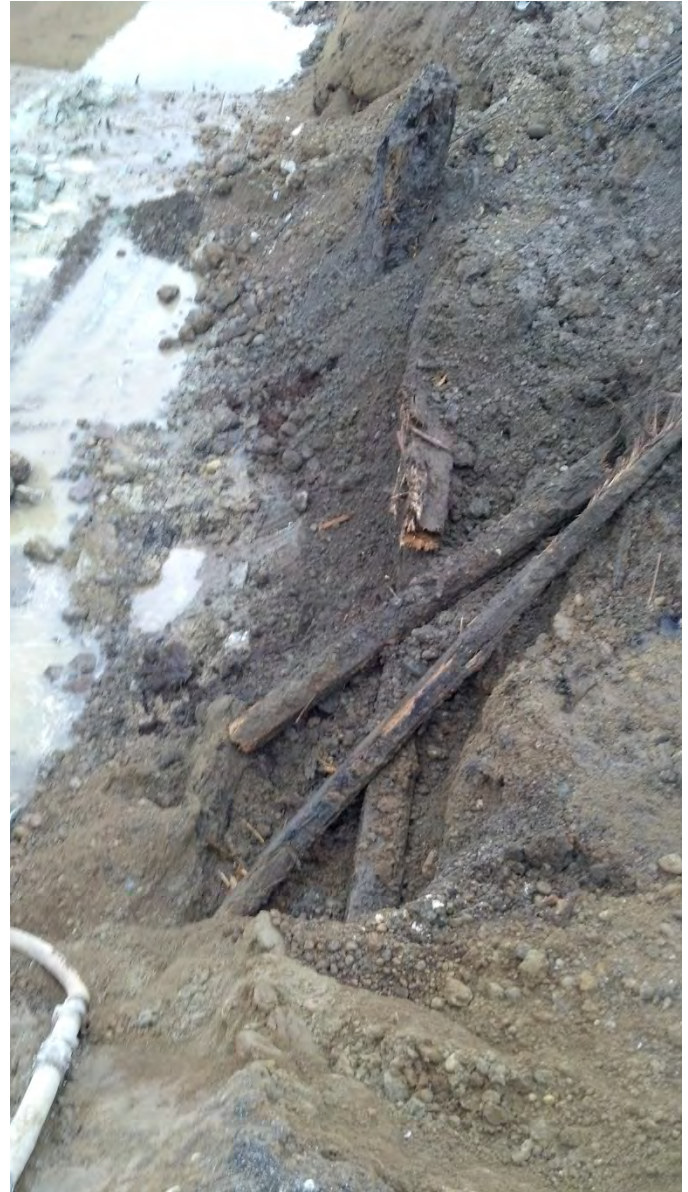
Photo 13 –Detail of cribbing and soils at base of excavation.
