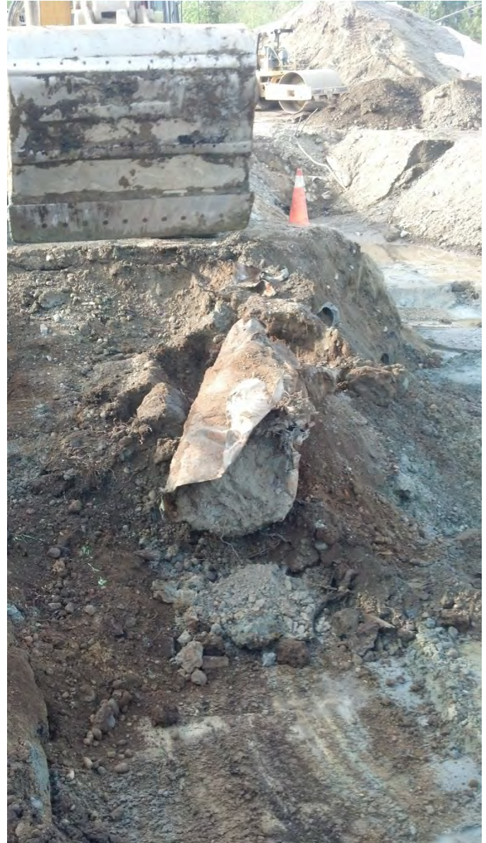
Photo 23 – UST during removal for ongoing soil excavation
