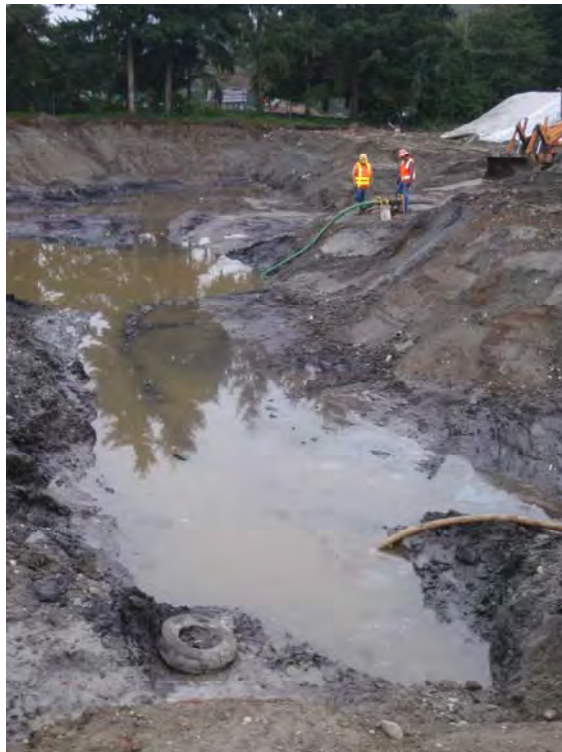
Photo 8 – Pumping ground water out of excavation (looking to east)
