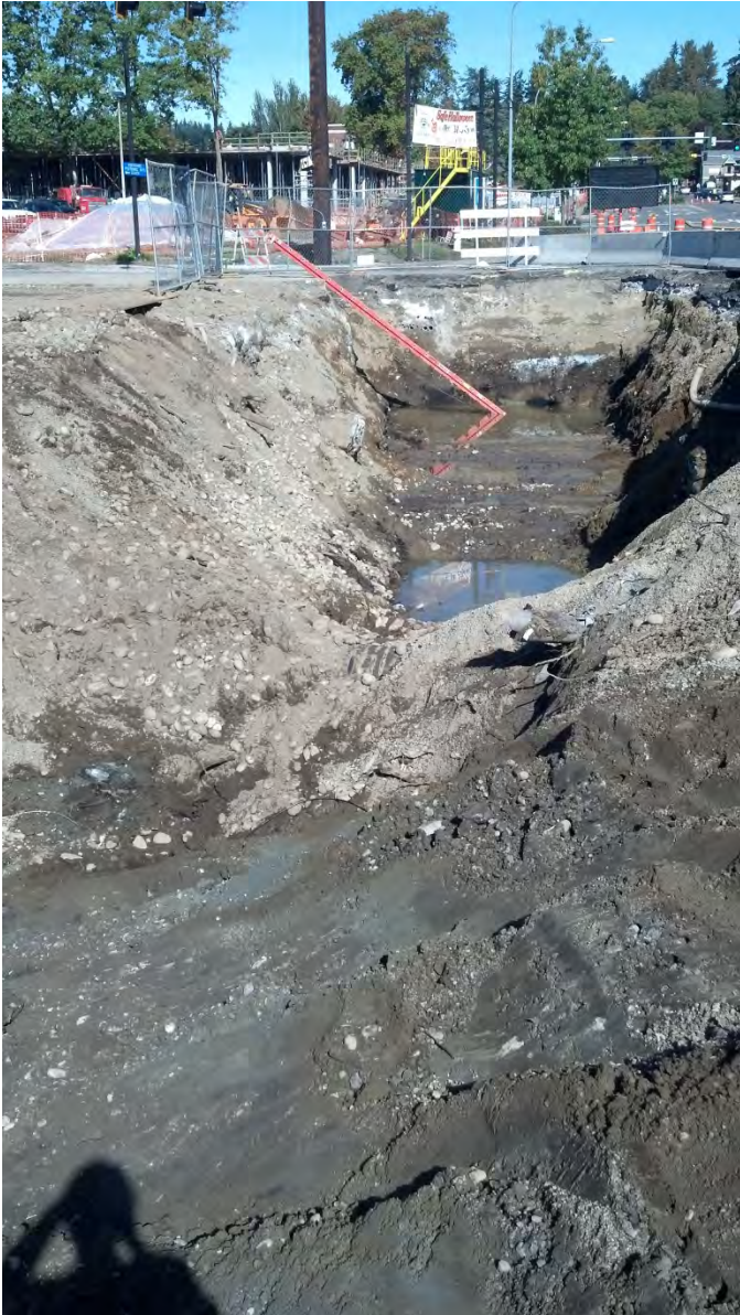
Photo 12 – Excavation along west side of SR-527, view north
