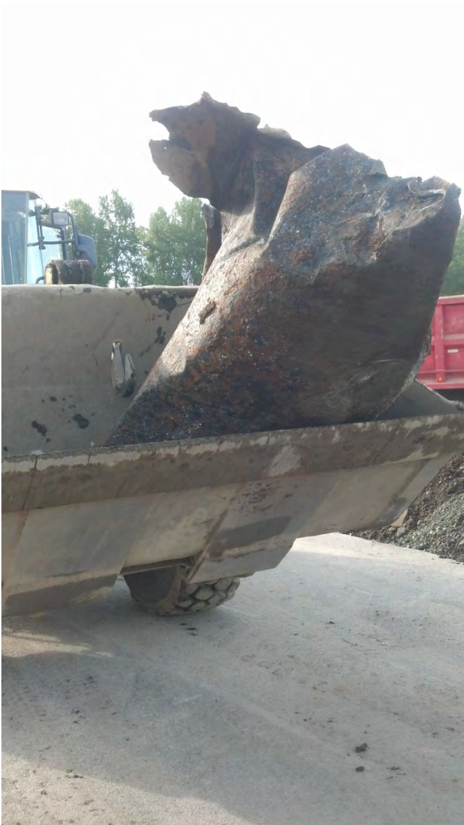
Photo 24 – 300-gallon UST after removal
