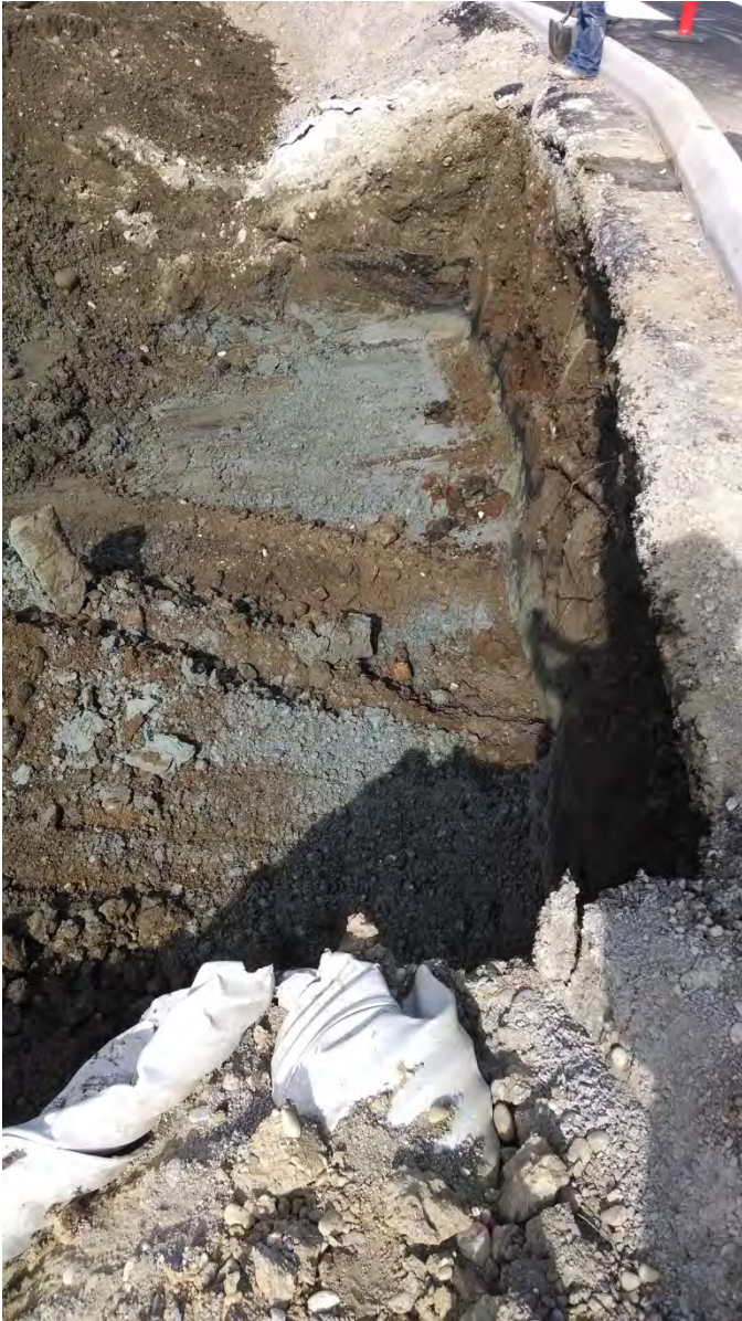
Photo 26 – Overexcavation of soils adjacent to and underlying Main Street
