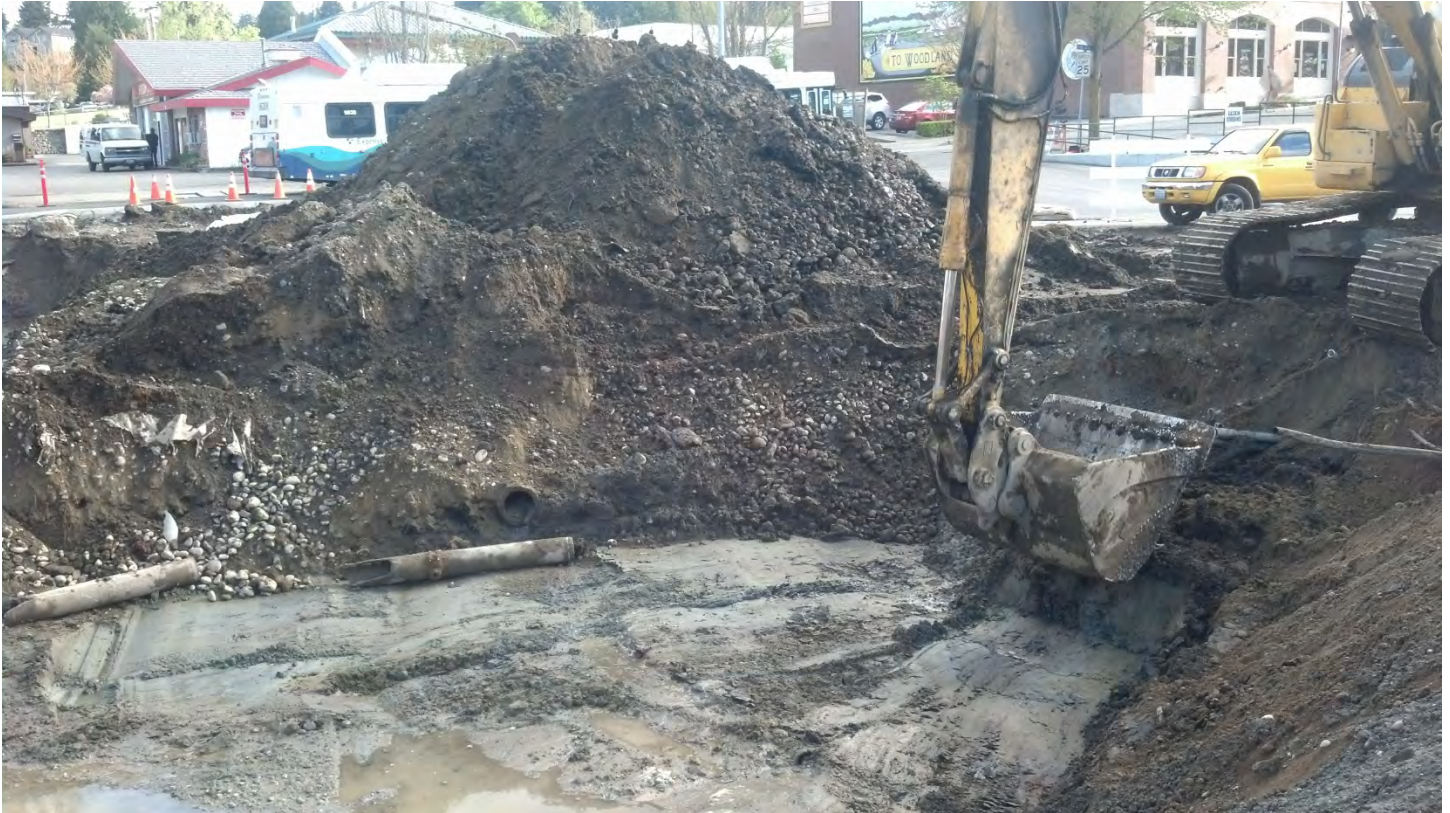
Photo 19 – Excavation along former SR-522, view north
