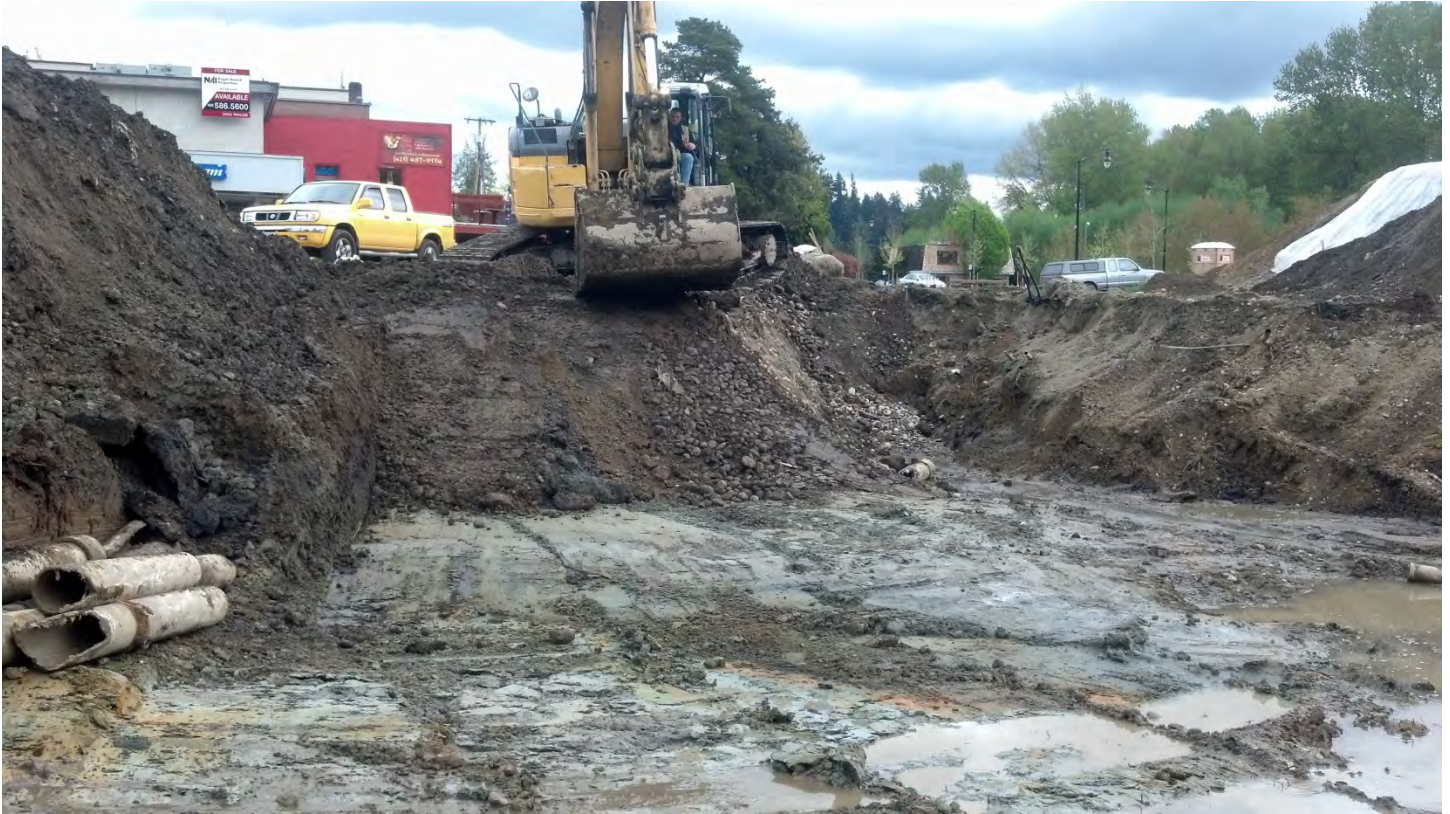
Photo 18 – Excavation along former SR-522, view east
