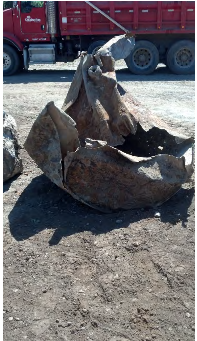
Photo 25 – UST emptied of soils and crushed for disposal
