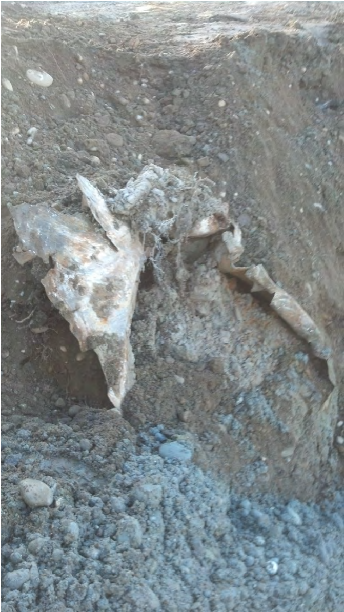
Photo 22 – Detail of UST end and underlying soils
