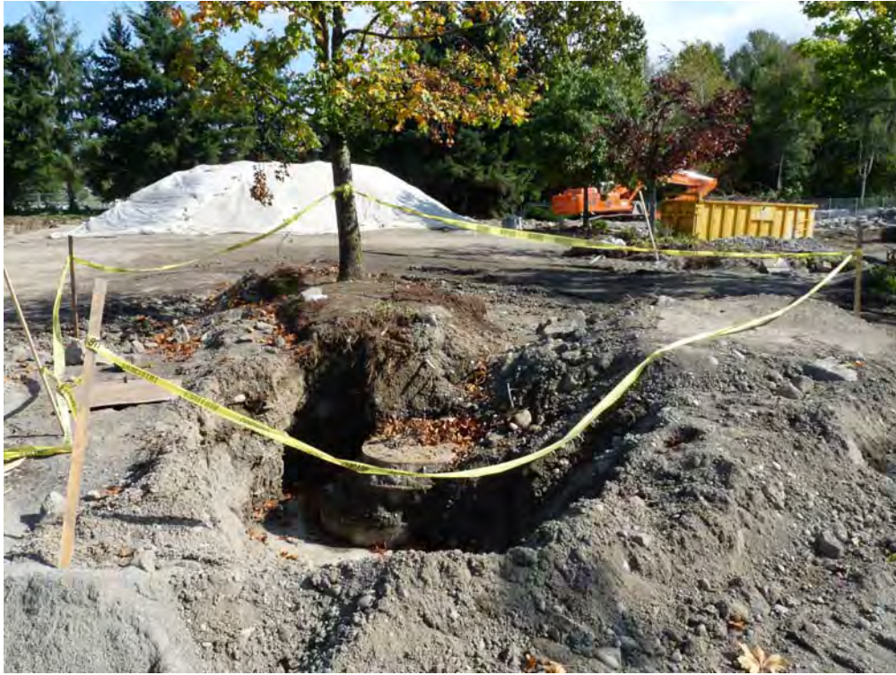
Photo 7 – Exposed manhole to Horse Creek culvert (looking to south)
