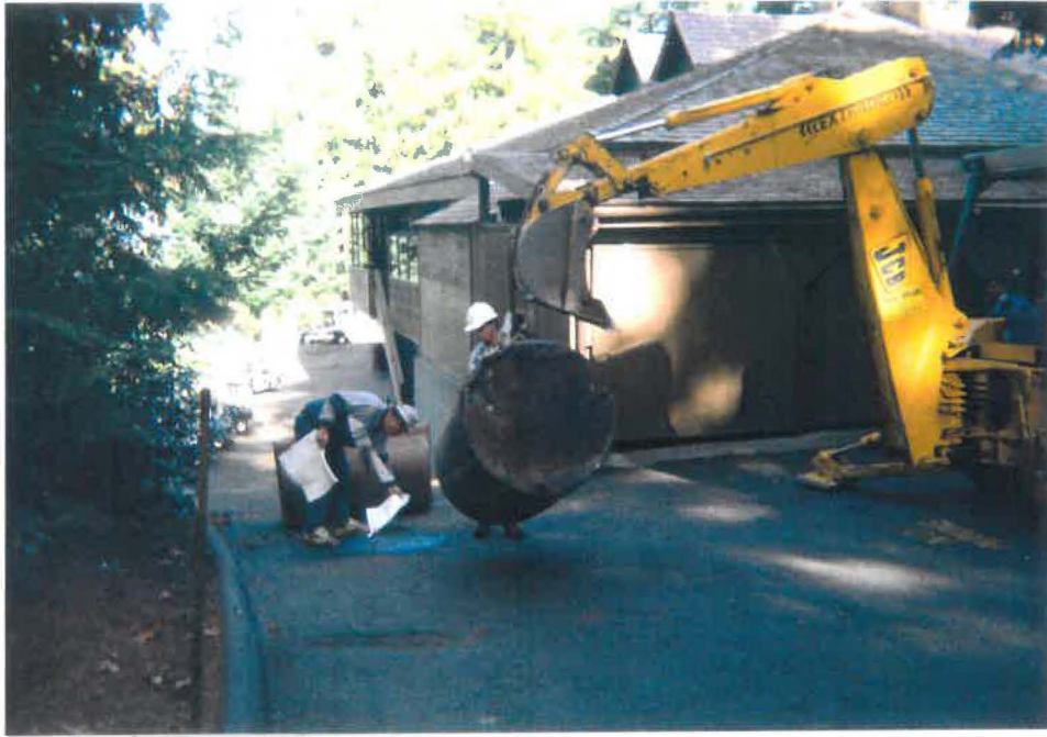
VIEW OF EXCAVATED TANK NEAR RESTAURNT/CLUB HOUSE
