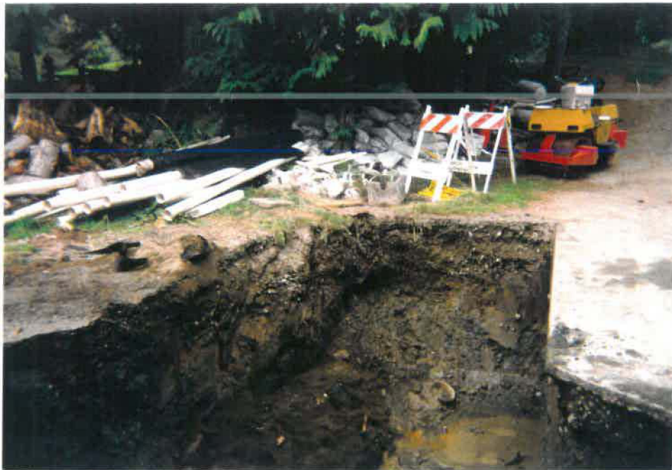
PIT FROM TANK #2 AT MAINTENANCE BUILDING
