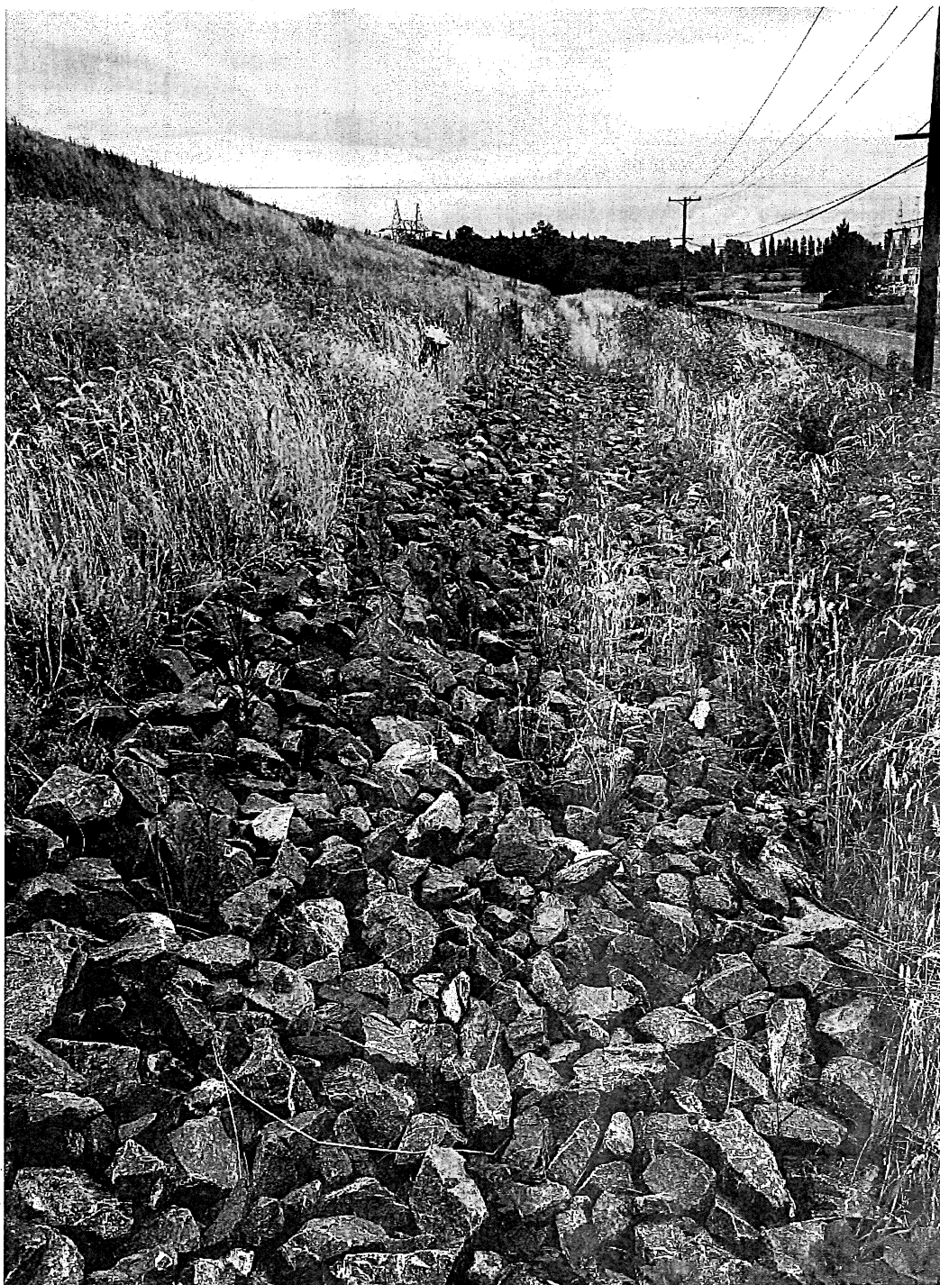
Photo 5: TLL south side anchor trench
