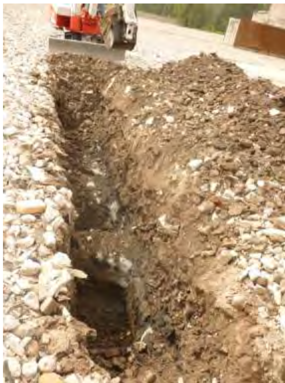
Photograph 10: Middle section of northern trench showing ecology blocks at TP-3 and TP-4 sampling locations, looking south.
