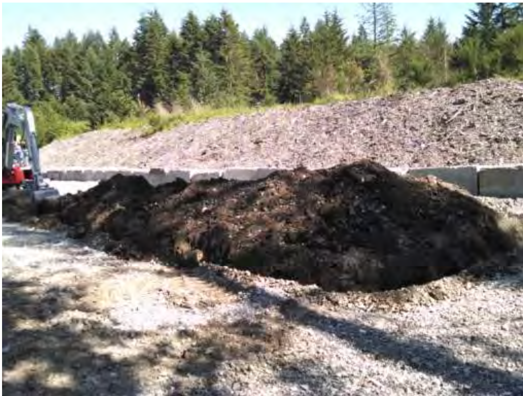
Photograph 8: Southern trench, looking southeast.
