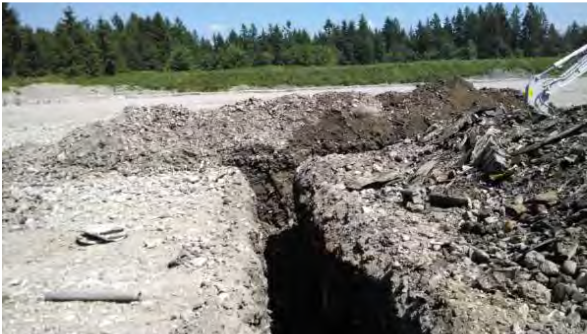
Photograph 9: North section of northern trench showing TP-1 and TP-2 sampling locations, looking east.
