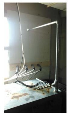
On October 6, 2015, the NAPL return and air supply lines were connected to MW15, MW22, and MW25.
