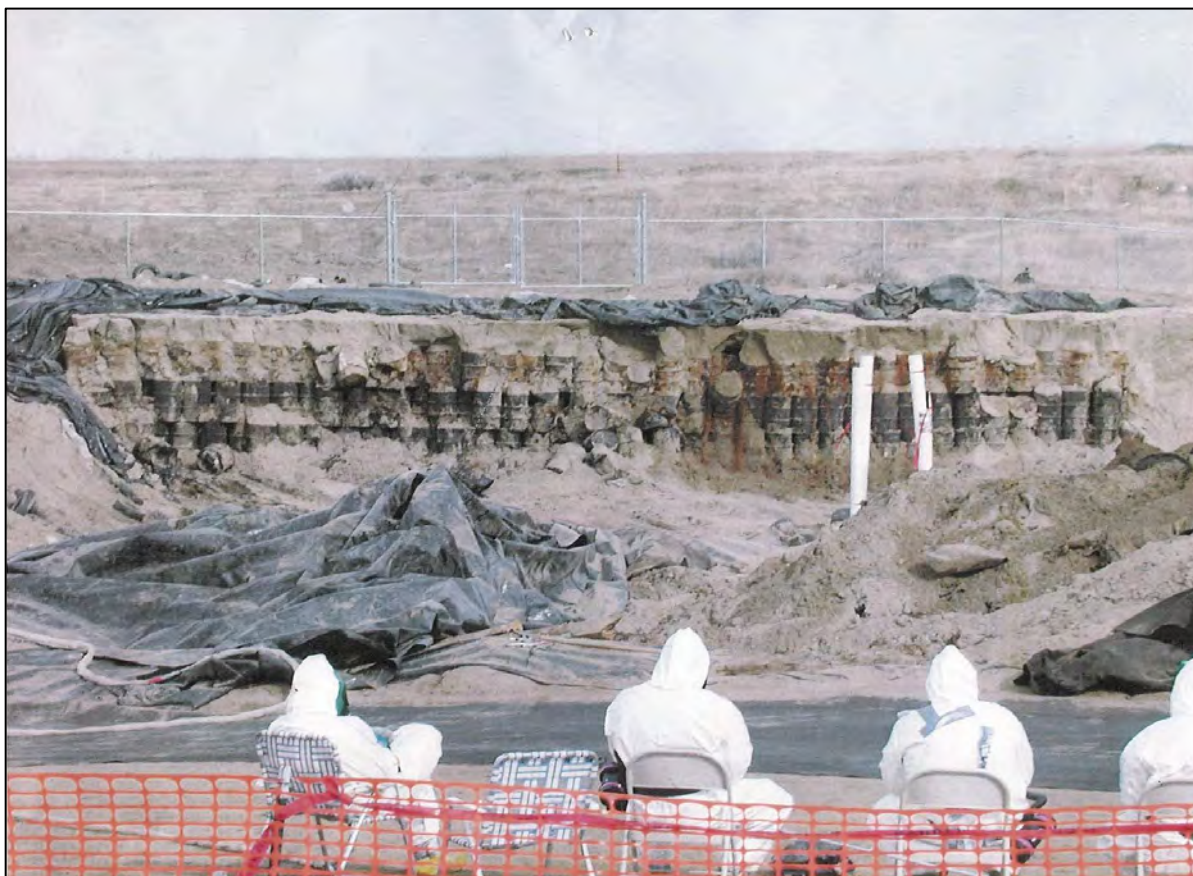
Figure 2.4. Zone B drum excavation. Some drums near the surface in contact with soil appear to have collapsed, while most of the drums in the interior of the drum stack still appear structurally intact (although they may have pitting failures that cannot be seen in the photo).
