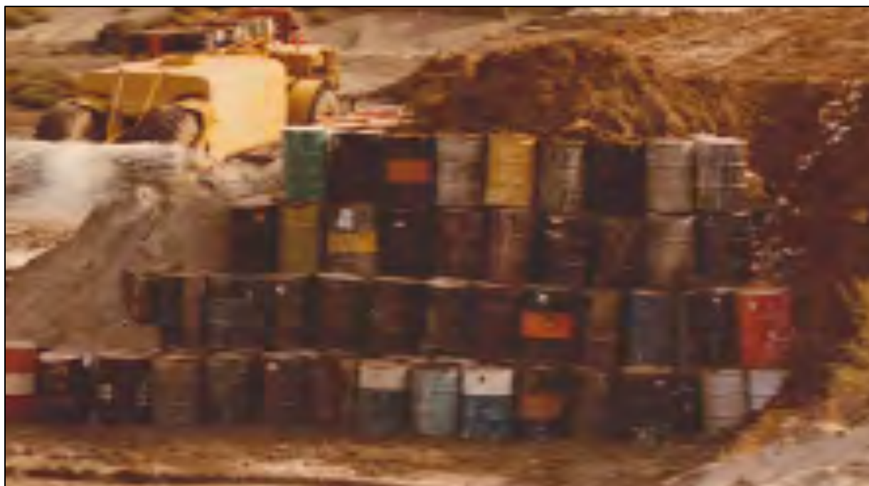
Figure 2.2. Close up photo of Zone A Stacked Drum emplacement. The Franklin County Planning Commission (1987a) wrote: “The space between the drums was backfilled with common debris, empty pesticide drums and small unidentified amounts of waste.”
