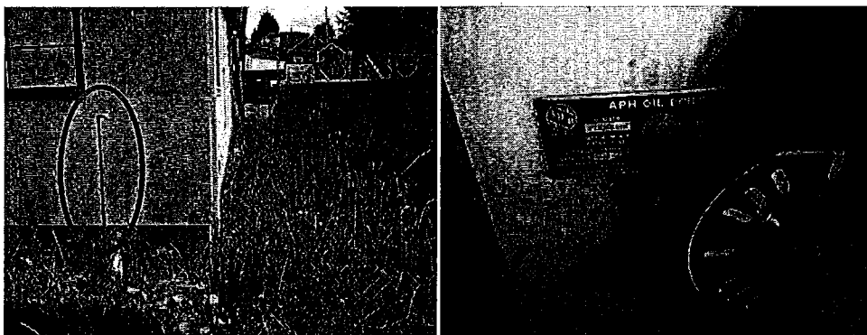
Suspected fuel tank vent line
