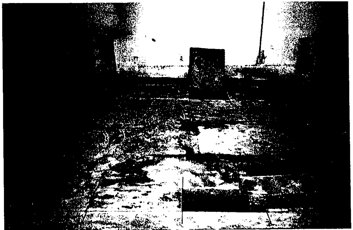
Photograph 2: A view of the former dry cleaning room inside of the building, looking west. Two trenches were cut in the concrete slab to access soils beneath the site..
